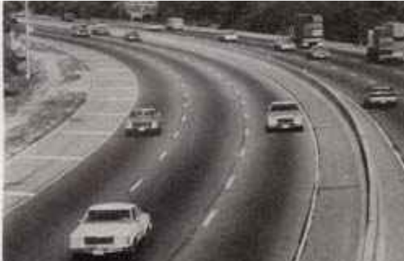
Level of Service A: Free-flow traffic with individual users virtually unaffected by the presence of others in the traffic stream.
