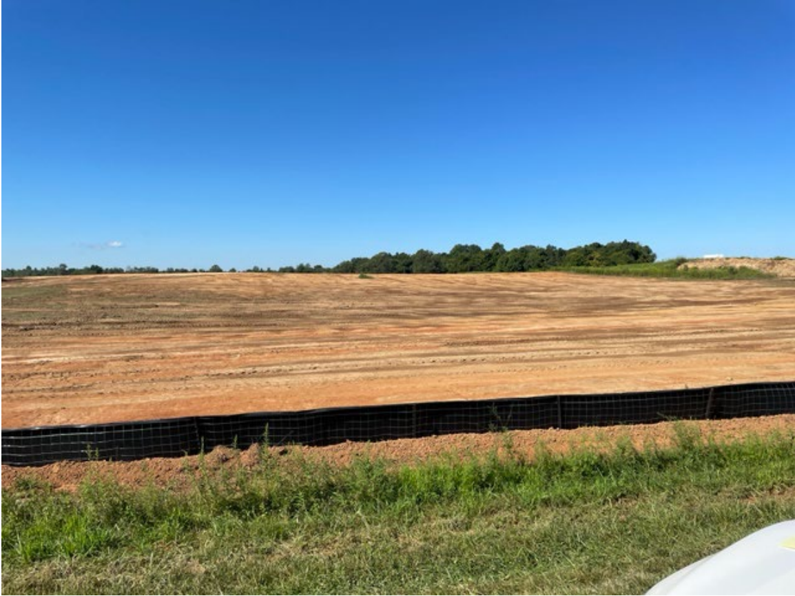
Figure C-16. Future project substation location across road from EKPC substation
