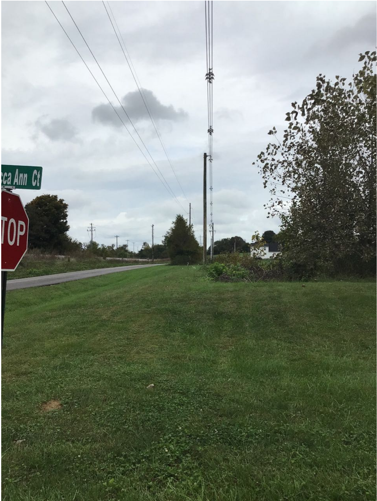
Figure 70 Existing 69 Bonnieville-Hardin County Transmission Line off Rebecca Ann Court
