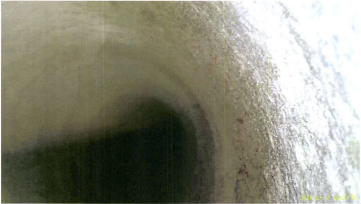
Competent Limestone bedrock at a depth of 25'
