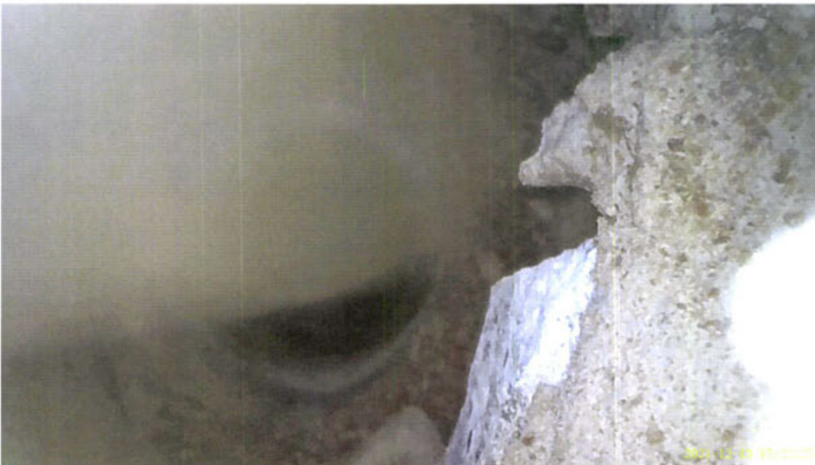
Void/weathering at a depth of 30'
