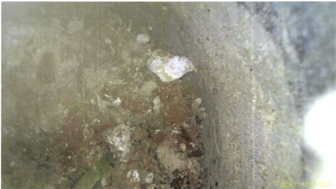
Closeup of the base of the core hole at -35'
