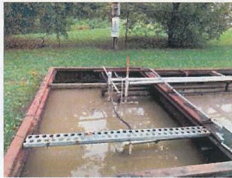
Clarifier Performance During Wet Weather (and No Aeration in Aeration Tank)
