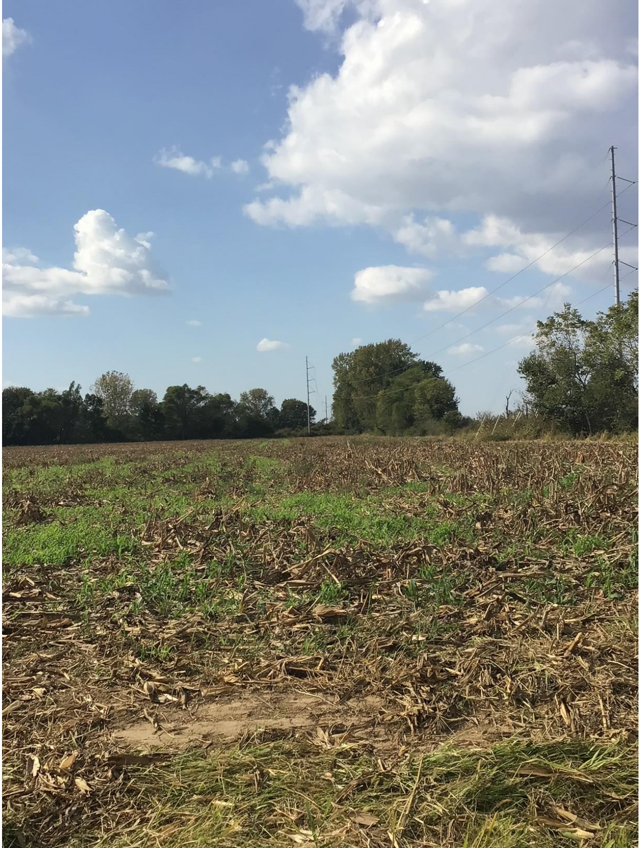
Figure 54 161 kV Transmission Line near the Proposed South Henderson Switching Station
