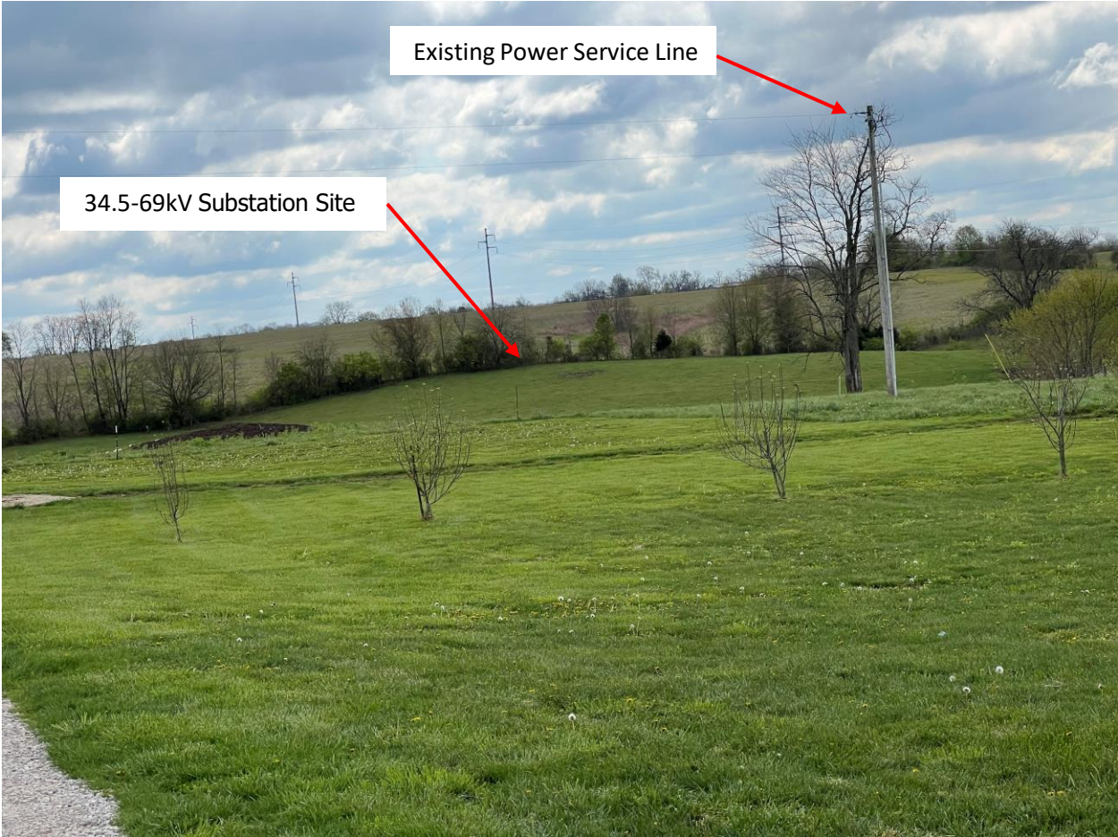
Picture (7) Location #6 Substation Site
