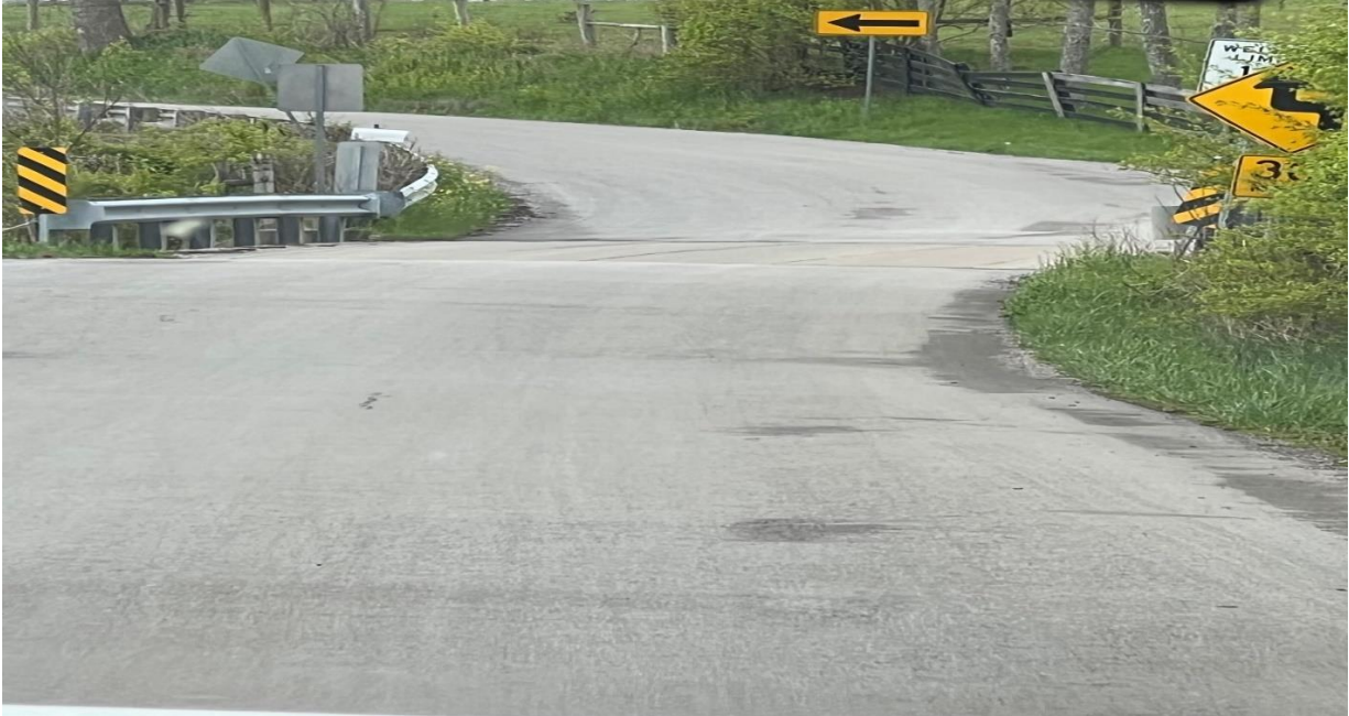
Picture (14) Bridge/Culvert on State Highway 393
