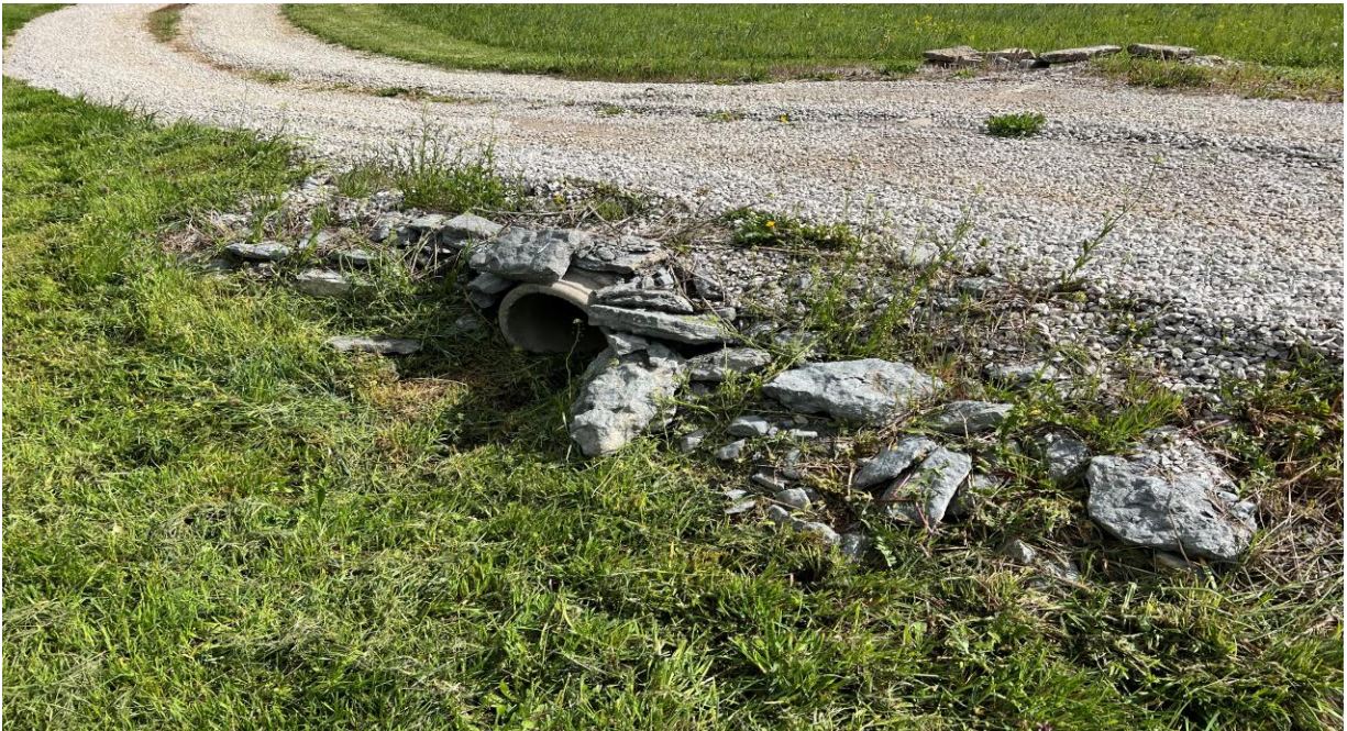
Picture (15) Gravel Road and drainage- (Republican Pike Rd /SR 393)
