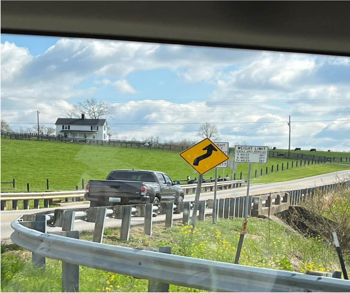
Picture (13) Bridge/Culvert on State Highway 393
