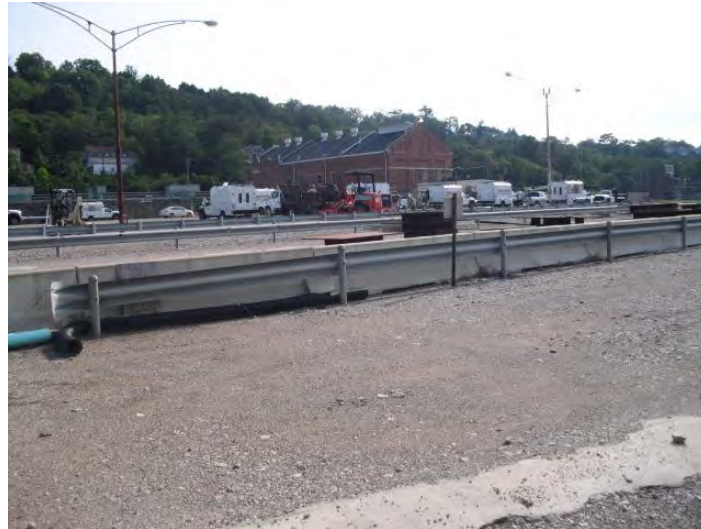
Figure 51: East Gas Works Plant
