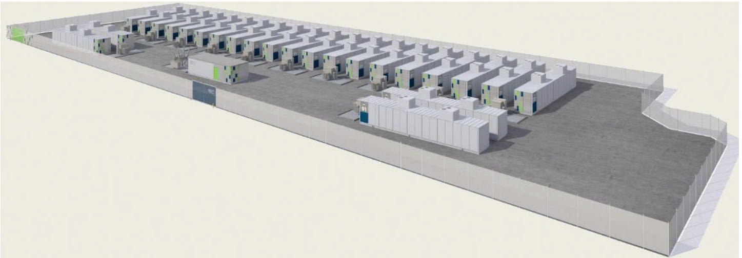
Figure 5: Typical 30 MW, 120 MWh Lithium-Ion Energy Storage Site 13
