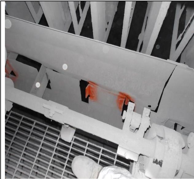
Top Left: Another example of missing collecting plate hammers along with broken shock bars in the same area. Top Right: A pallet of replacement hammers for the ESPs. A few different hammer bracket styles are being used in the unit. Bottom Left: A photo of a broken high voltage rapper rod. This rod was touching the high voltage from the field beside it. Bottom Right: A photo of a broken high voltage lifting rod.
