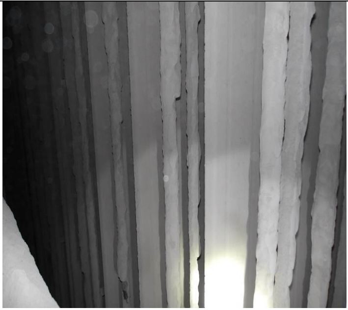
Top Left and Right and Bottom Left: Examples of dirty wires where the high voltage rappers were not in operation. Bottom Right: An example of a broken collecting plate hammer. Many hammers were found broken, missing or laying on the ground.
