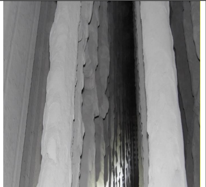
Top Left and Right and Bottom Left: Examples of dirty wires where the high voltage rappers were not in operation. Bottom Right: An example of a broken collecting plate hammer. Many hammers were found broken, missing or laying on the ground.
