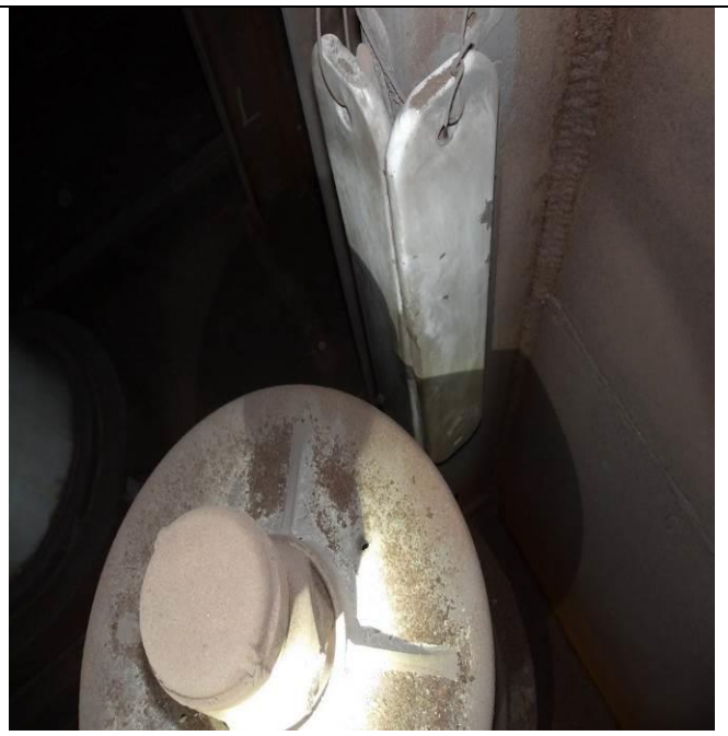
Top Left and Right: General views of the rooftop area. Bottom Left: A general view of an insulator compartment area. In view is a high voltage lifting rod insulator. Bottom Right: A photo of the insulator compartment stiffeners that were added in the past. In many areas, these were located too close to the top plates of the high voltage support insulators. Spark and arc damage was observed on every one that was inspected during this outage.
