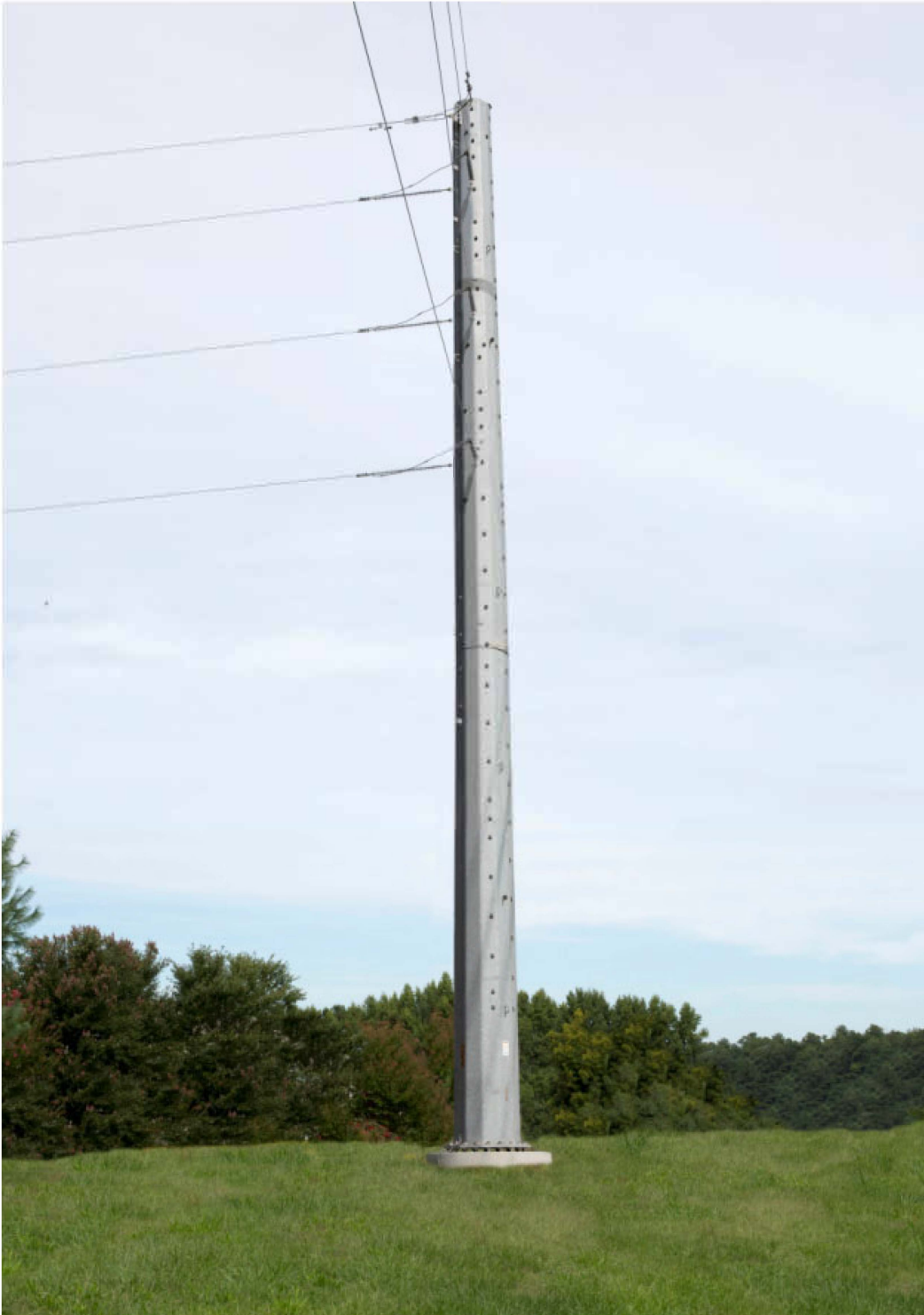
COMPARABLE EXISTING STRUCTURE PHOTOGRAPH
