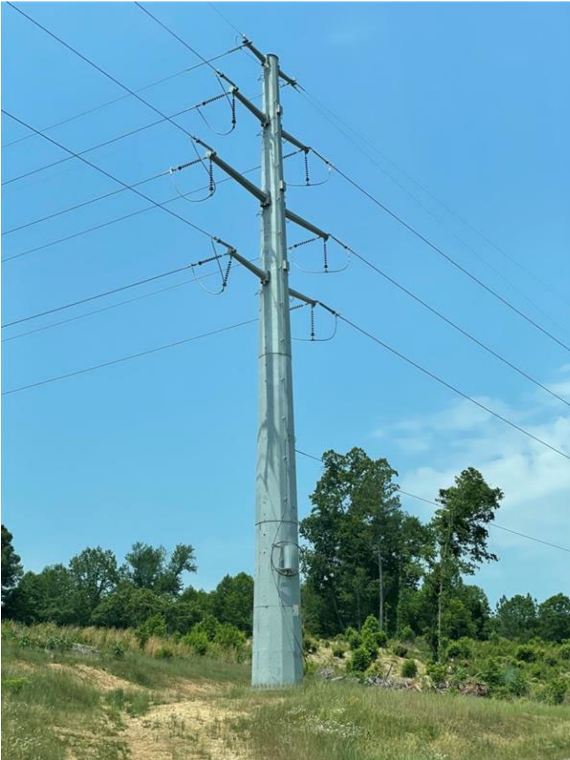
COMPARABLE EXISTING STRUCTURE PHOTOGRAPH
