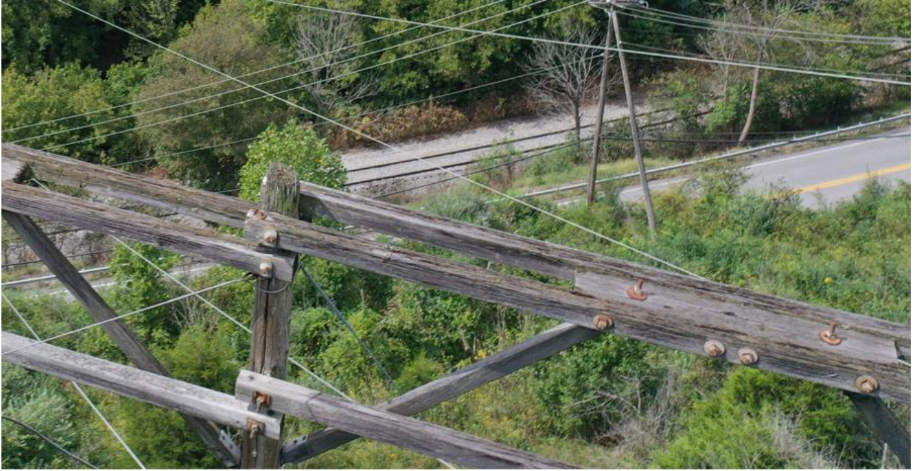
Beaver Creek-Garrett 2 Structure K336-58 Crossarm Splitting Page 1 of 1
