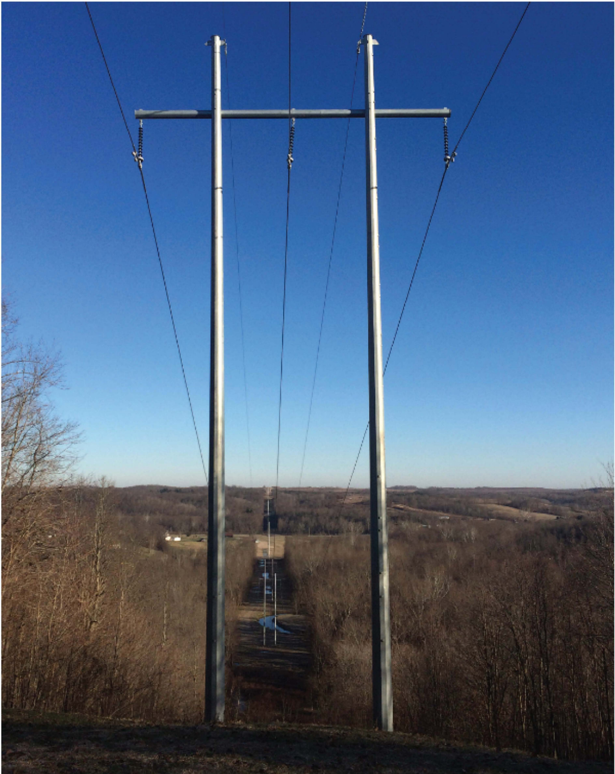
COMPARABLE STRUCTURE PHOTOGRAPH
