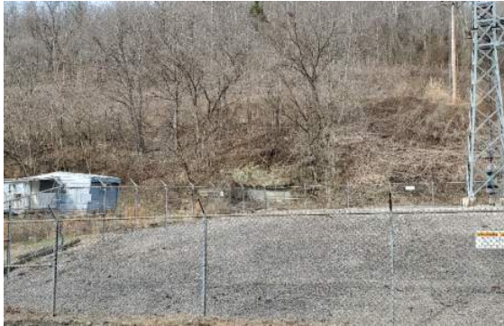
Photograph 1 Portal Location behind Existing Garrett Substation
