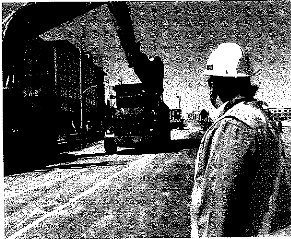
Figure 17-1: High-visibility Clothing Helps Equipment Operators See Workers
