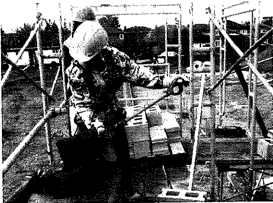
Figure 16-1: Wear Gloves and Cover Exposed Skin To Protect Against Hazards
