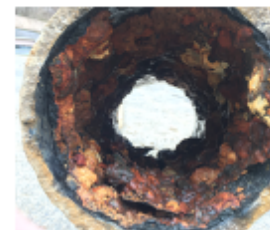
6" unlined cast iron pipe
