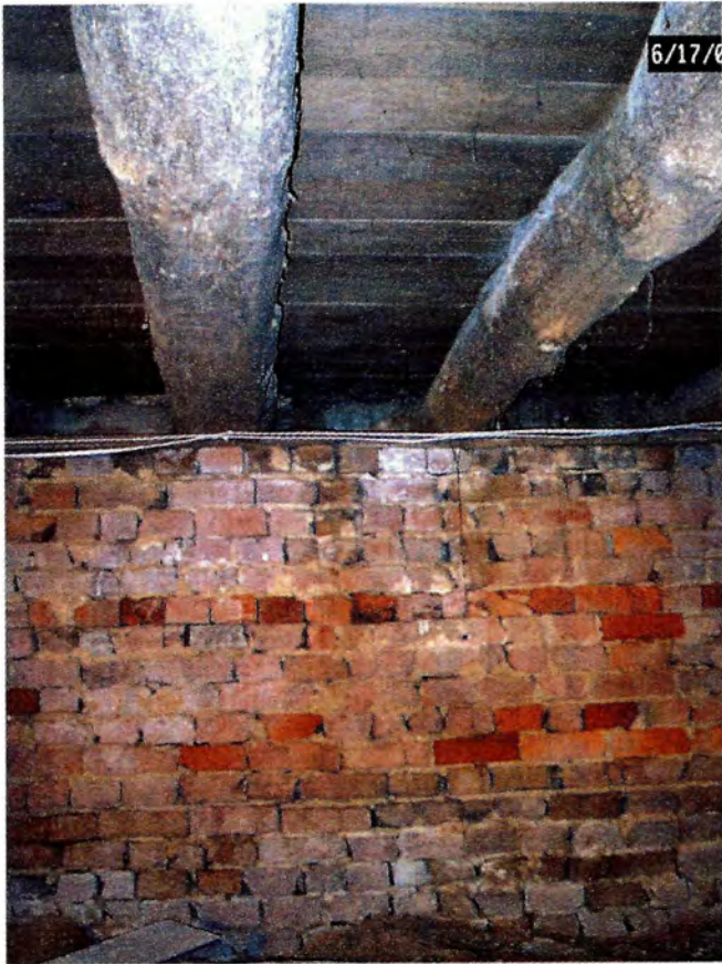
South wall of basement
