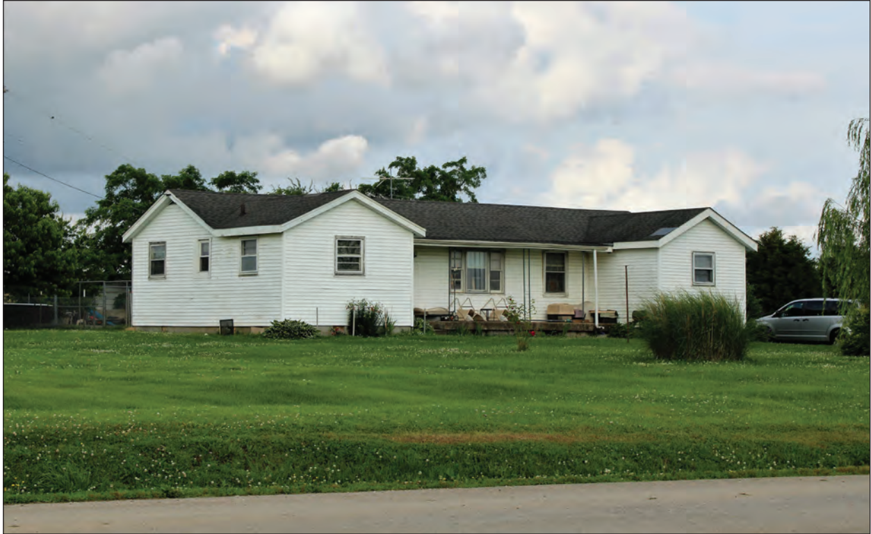
A. Looking Southeast
