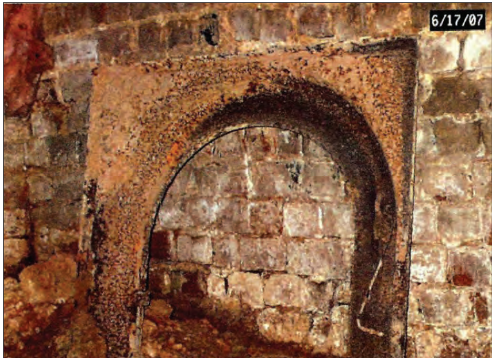
B. Basement Fireplace Frame Source: Stuart 2007
