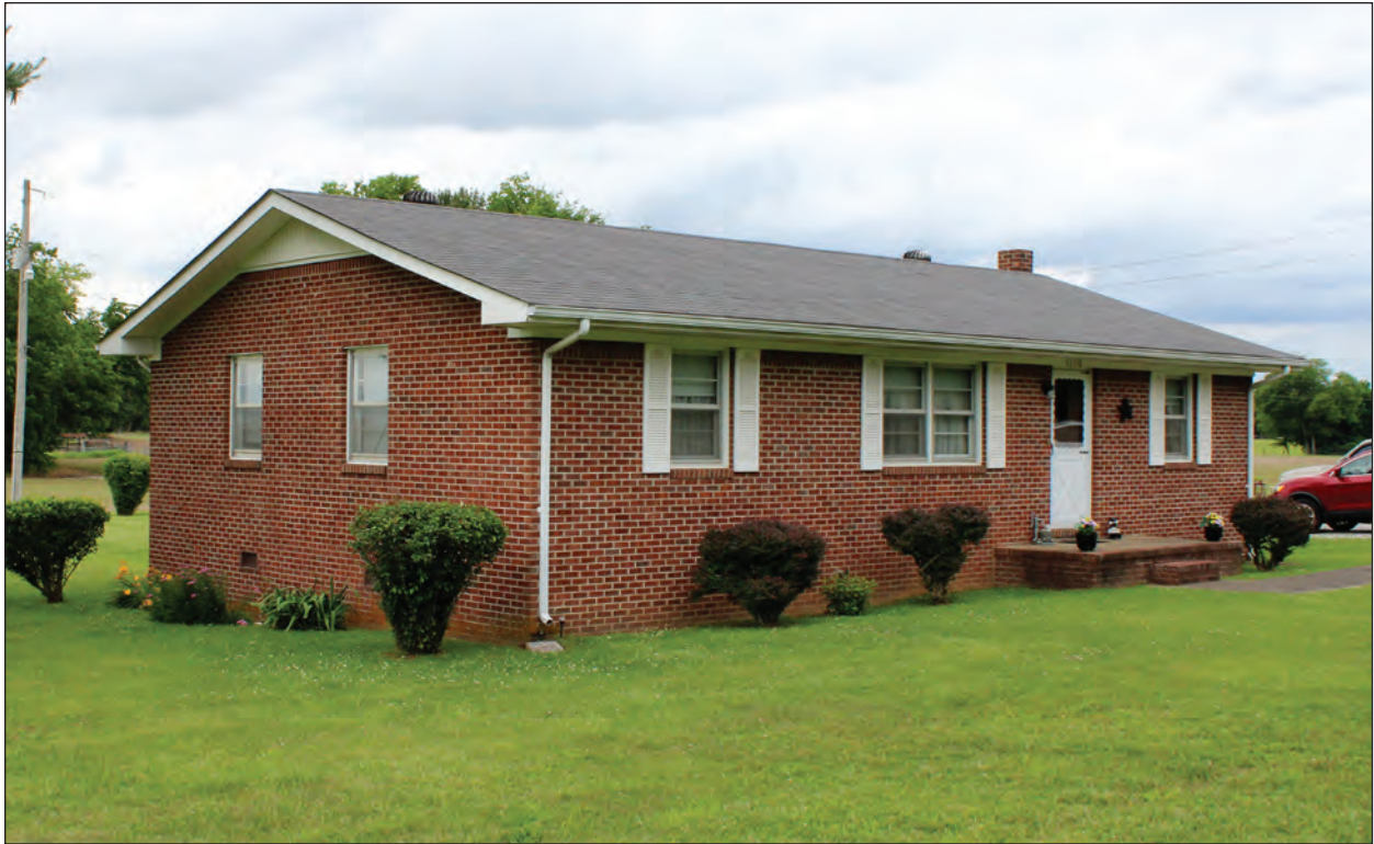
A. Looking Northeast
