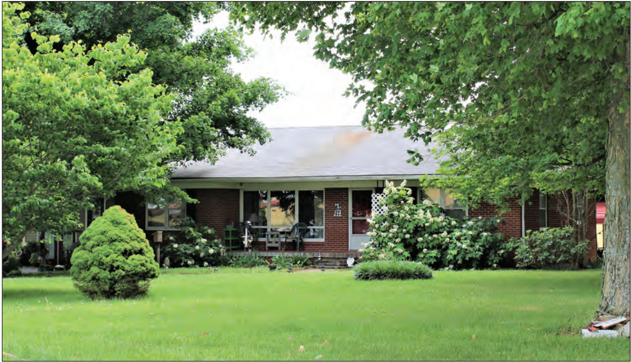
A. Looking East
