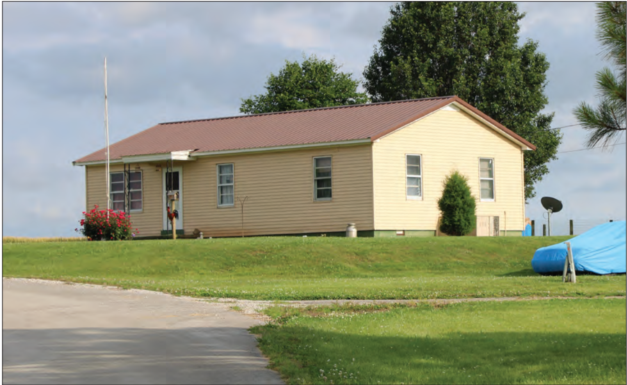
A. Looking Southeast
