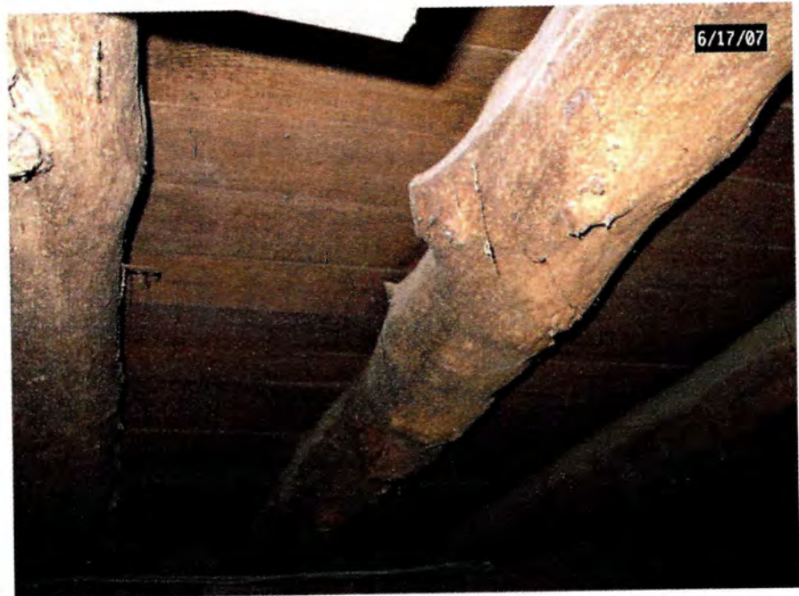
Logs used as floor supports.
