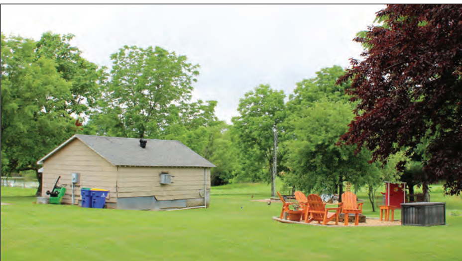
C. Outbuilding, Looking Southwest
