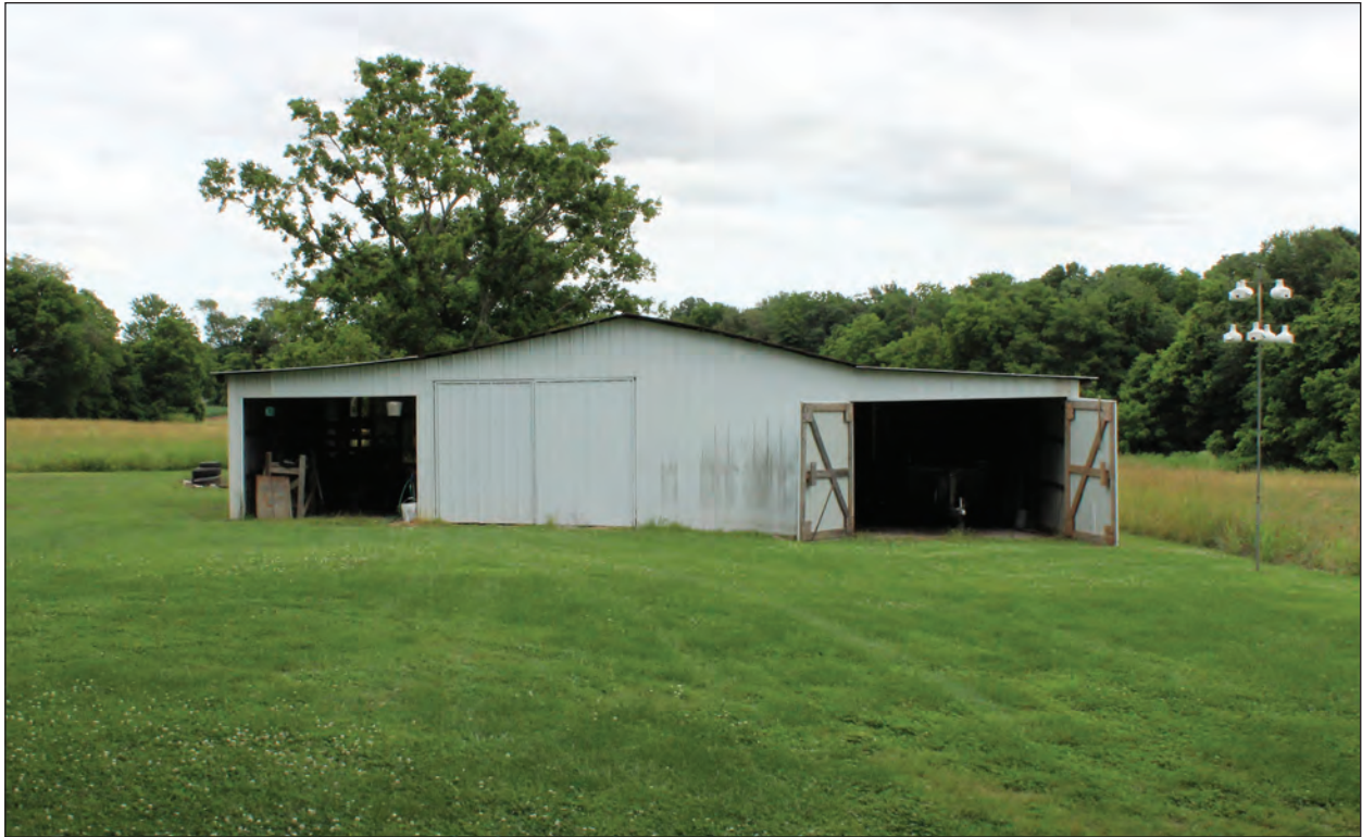
A. Barn, Looking Southeast
