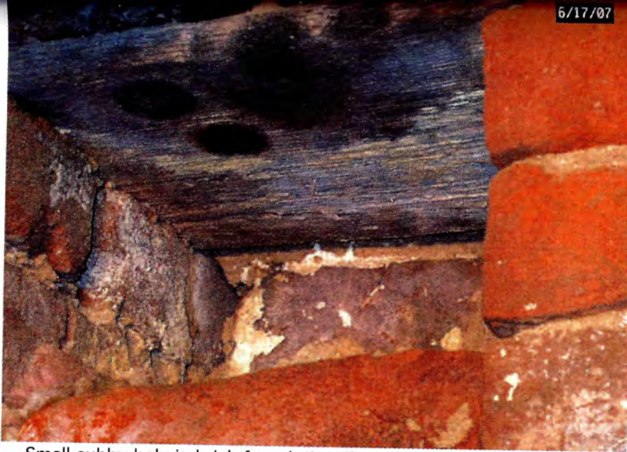
Small cubby hole in brick foundation showing where former residents had placed candles or lamps scorching the wood above.
