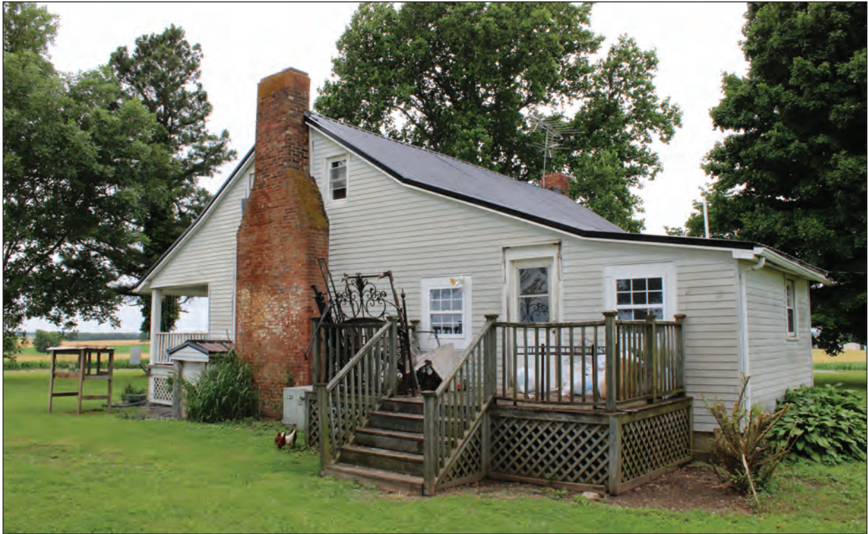
A. Looking West
