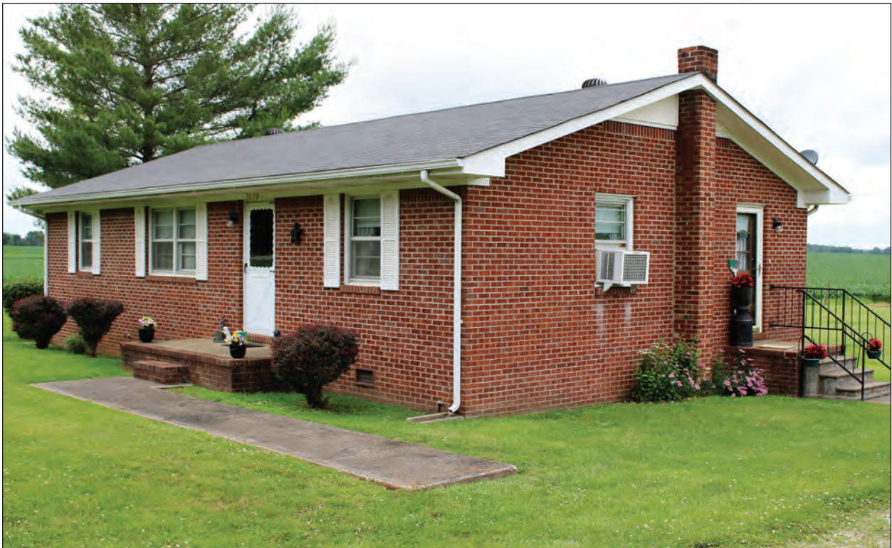
B. Looking Northwest
