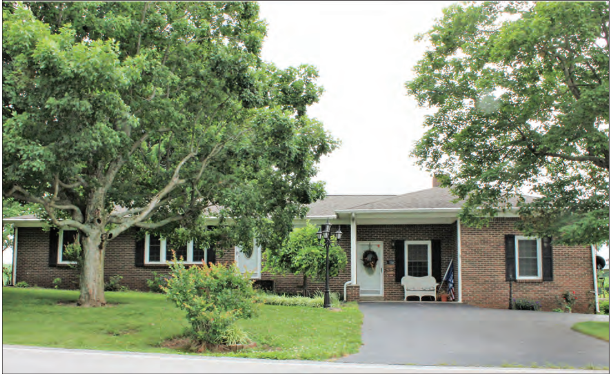
A. Looking East
