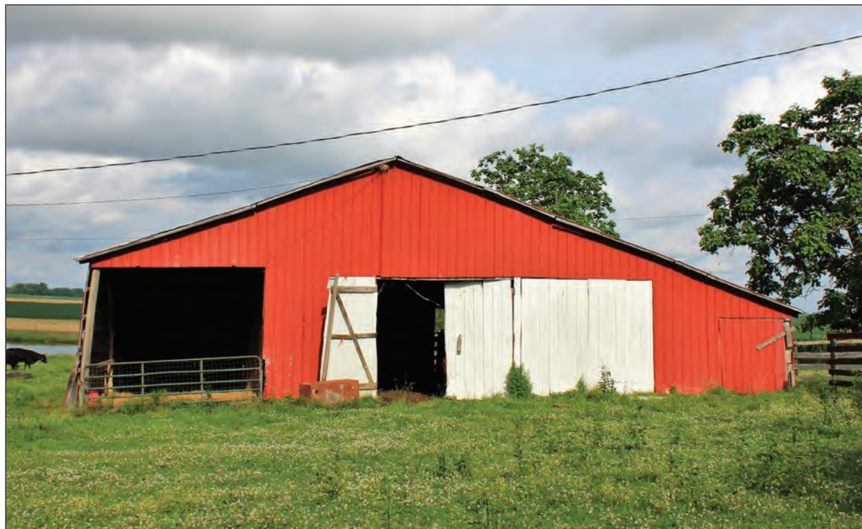
B. Barn, Looking East
