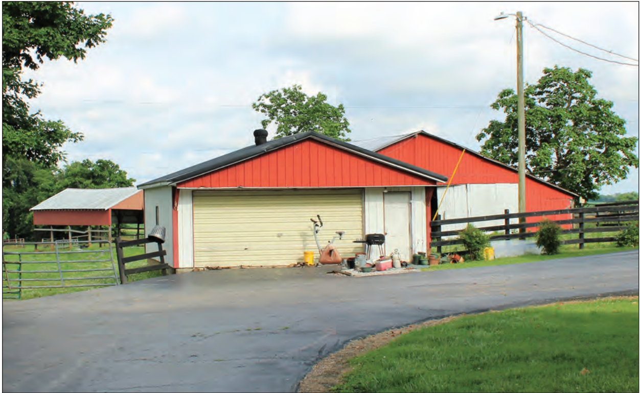
A. Equipment Shed, Garage and Barn, Looking East
