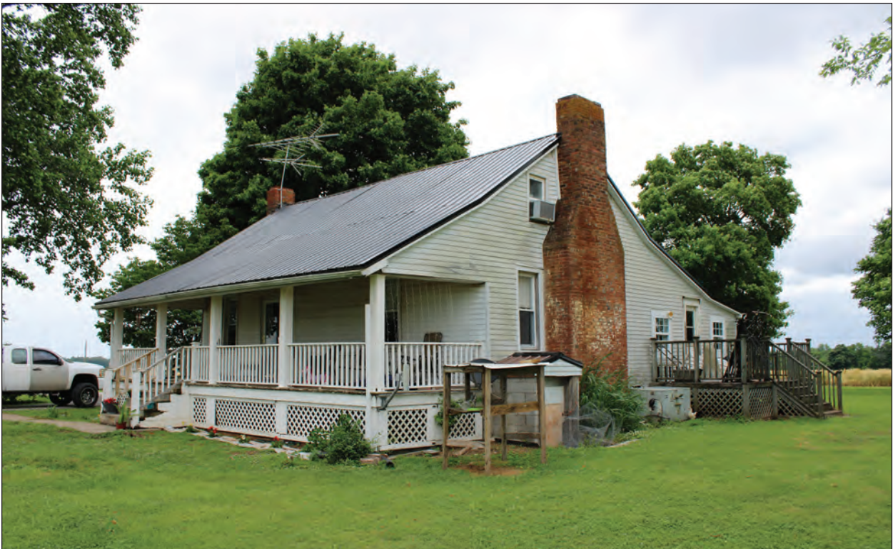
B. Looking Northwest
