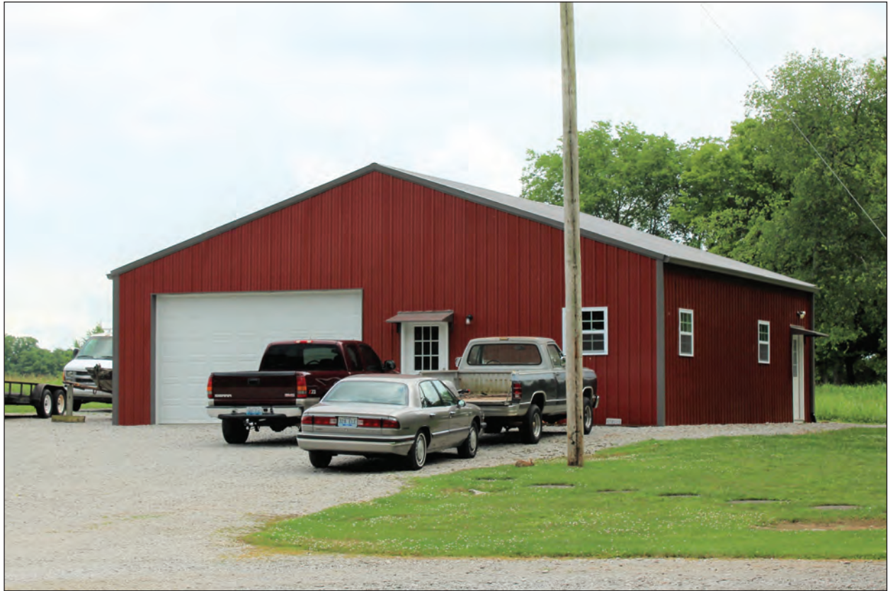
Figure 108. Photographs, Marion Acres Farm Machine Shop, Looking Southeast
