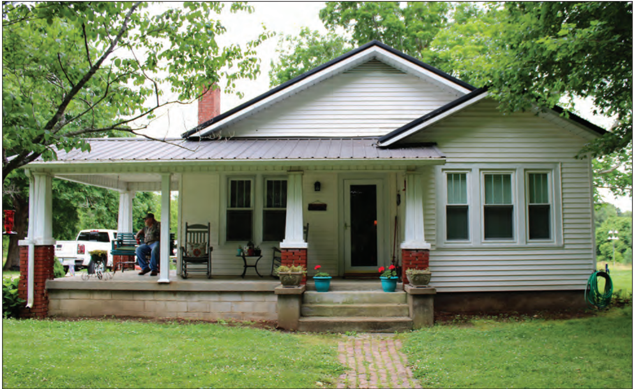
A. Looking Southeast
