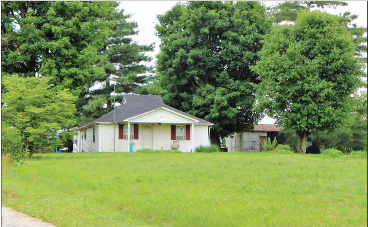
A. Looking Southwest
