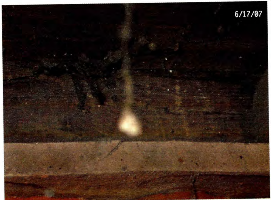
possible view of log used in original construction.
