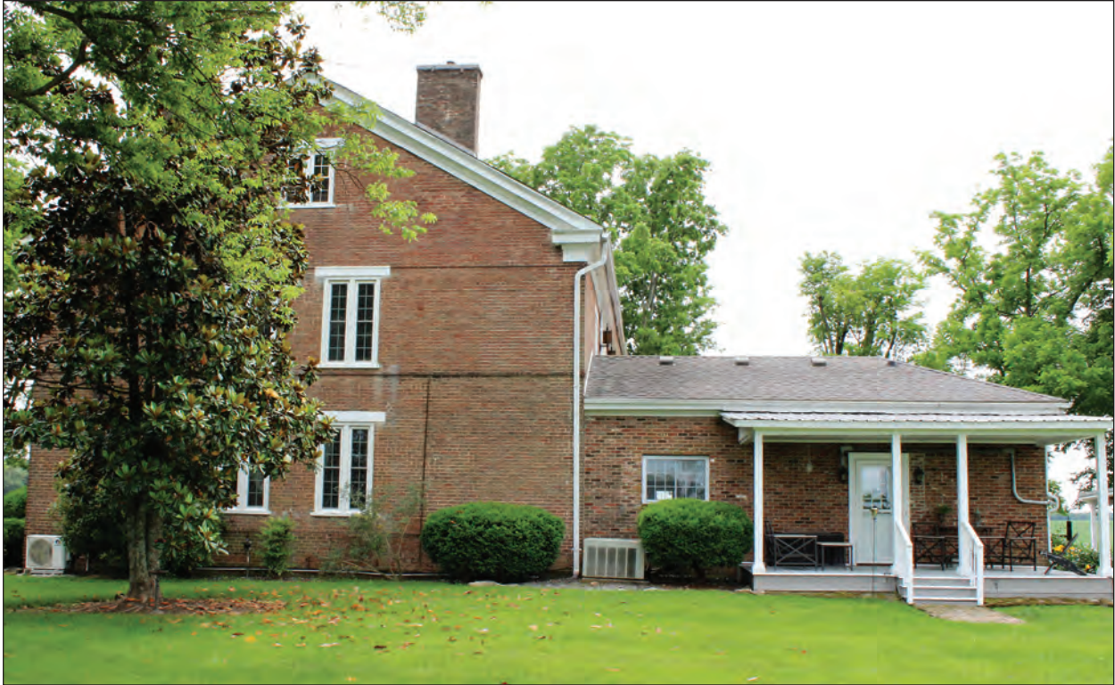
A. Looking West
