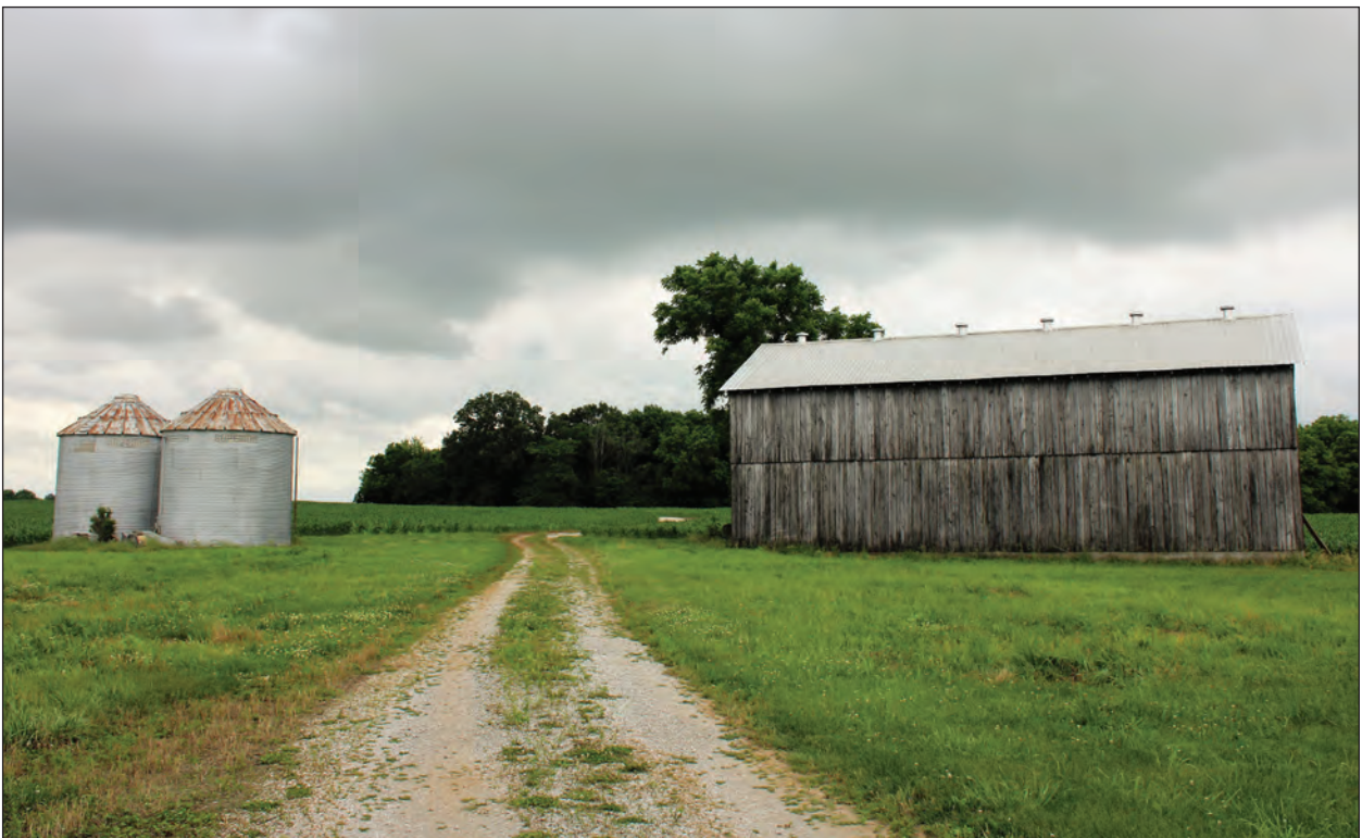
B. Silos and Tobacco Barn, Looking Southwest
