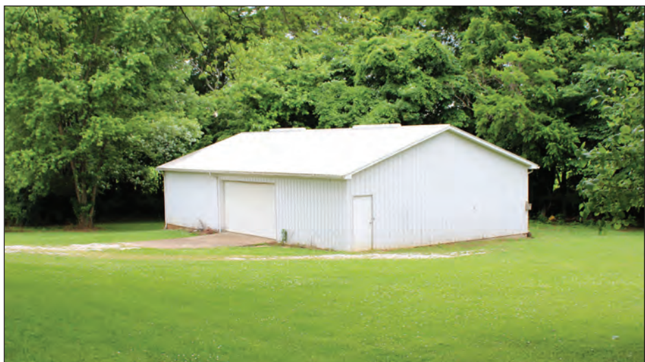
C. Metal Shop, Looking Northwest
