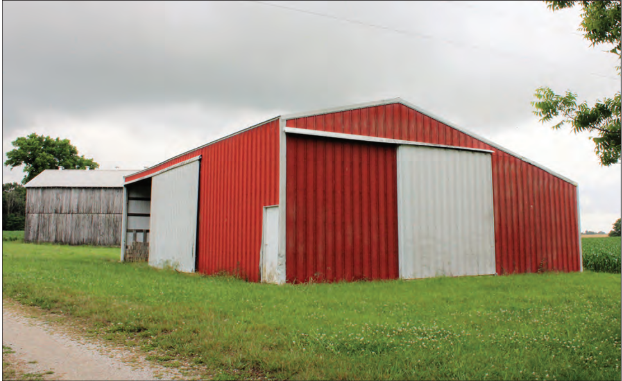
A. Utility Shed, Looking South
