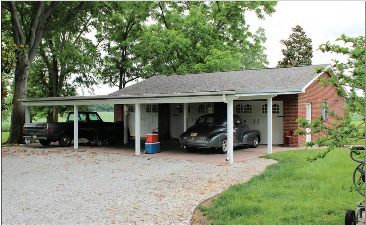
A. Garage, Looking Northeast
