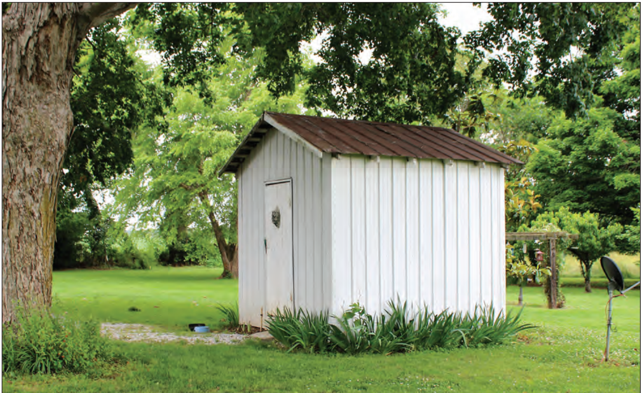
B. Shed, Looking East
