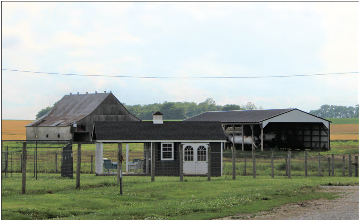
B. Storage Shed and Equipment Shed, Looking Northwest
