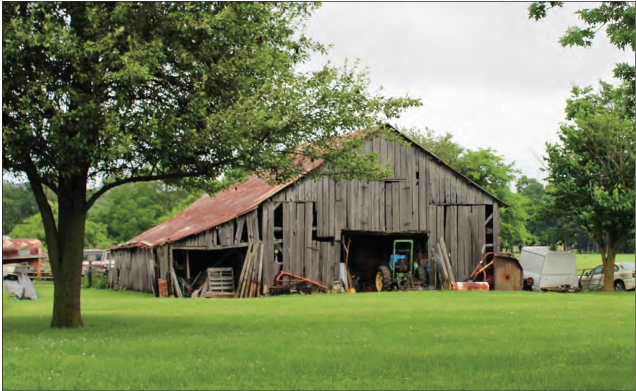
A. Barn, Looking Northeast
