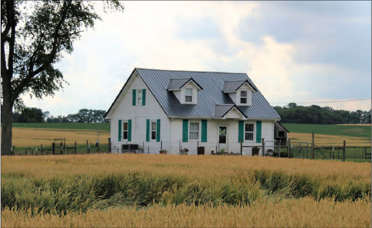
A. Looking West
