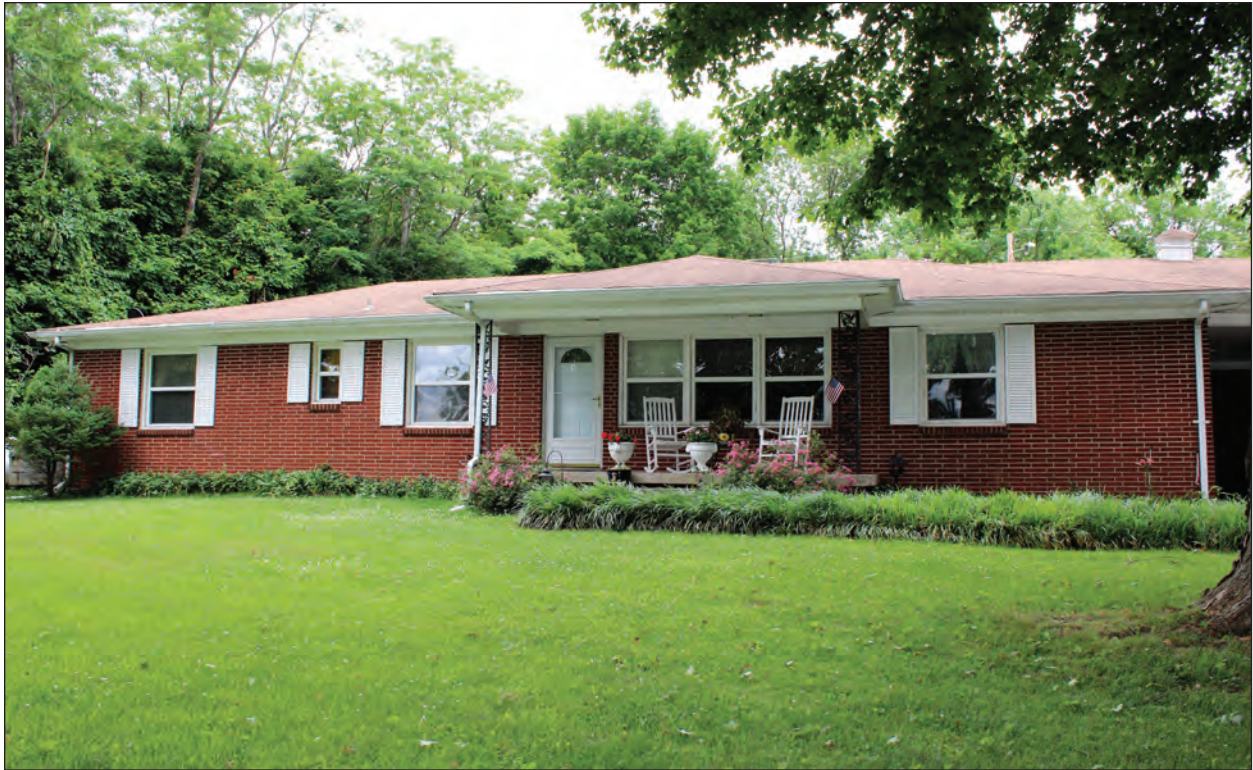
A. Looking Southeast
