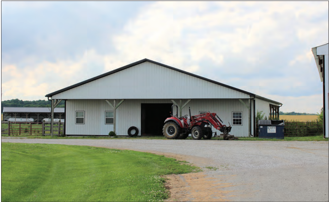
A. Office Shed, Looking Northwest
