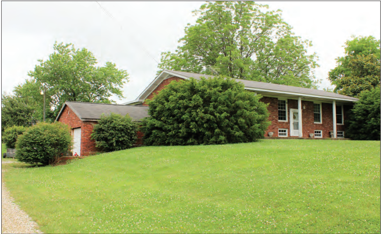
A. Looking Northeast
