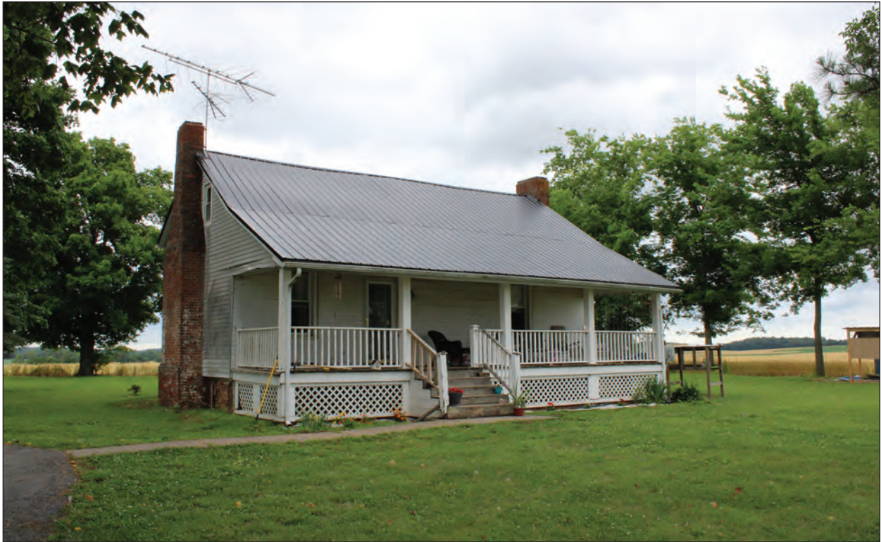
A. Looking Northeast
