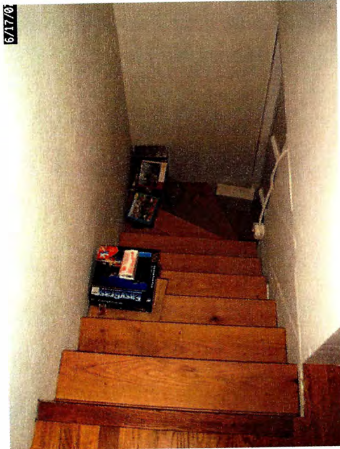
Looking down existing steps from upper level.
