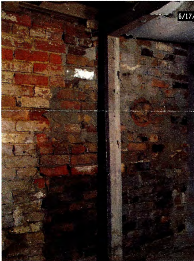
View of basement East wall where a wood furnace once set.
