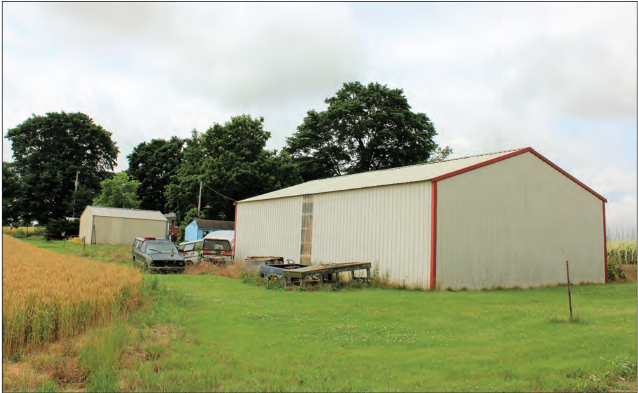
A. Workshop and Shed, Looking Southwest
