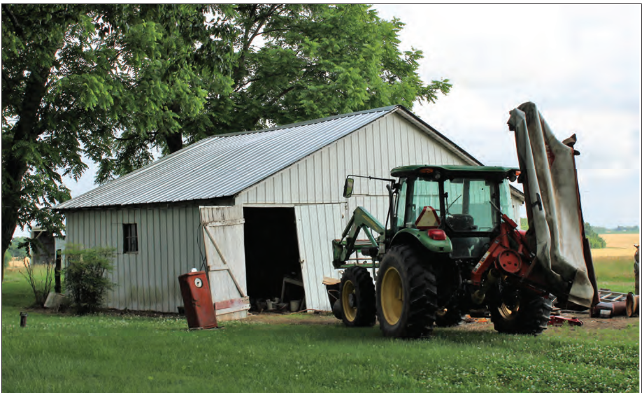
B. Shed, Looking Southeast
