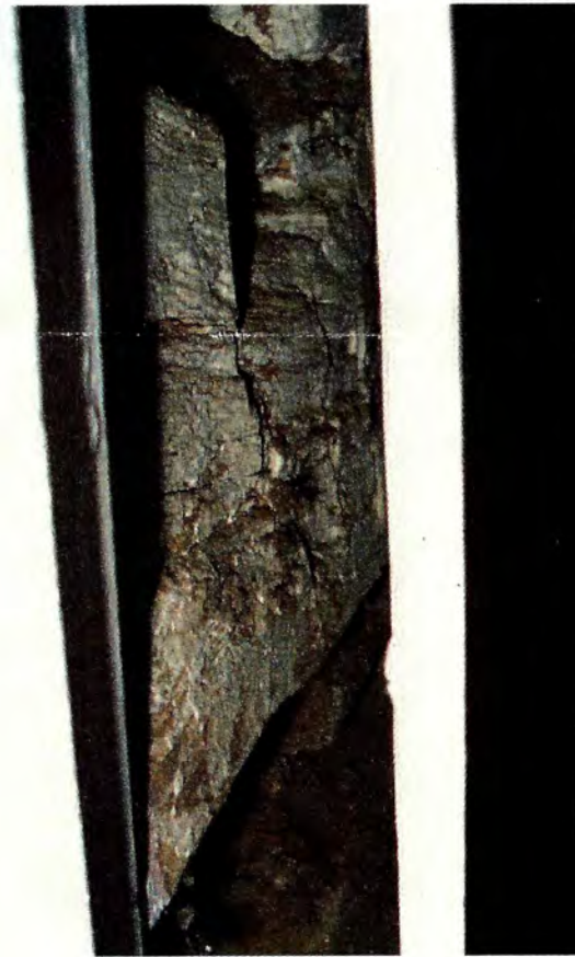
Close up of gap between doorway + wall at top of the stairway
