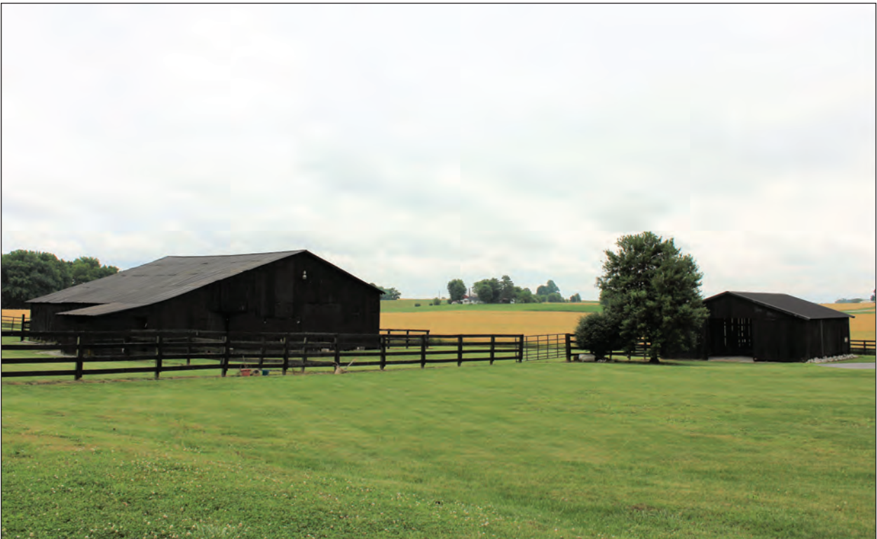
B. Outbuildings, Looking East
