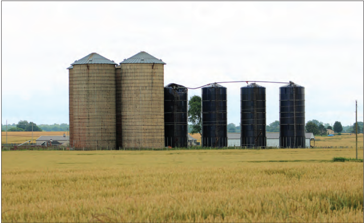
A. Silos, Looking Southeast
