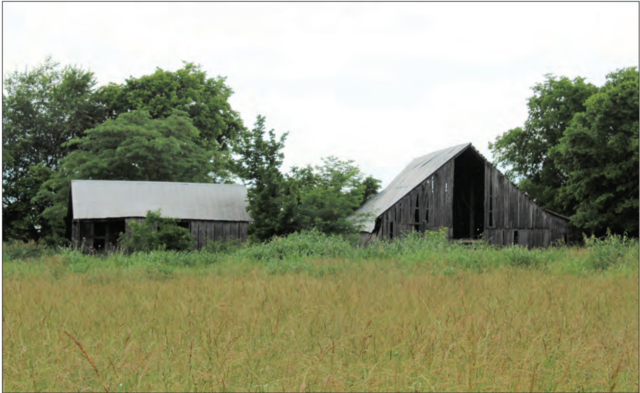
A. North Tobacco Barn and Small Barn, Looking West
