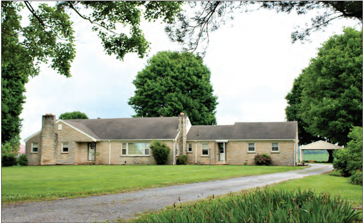
A. Looking Northeast
