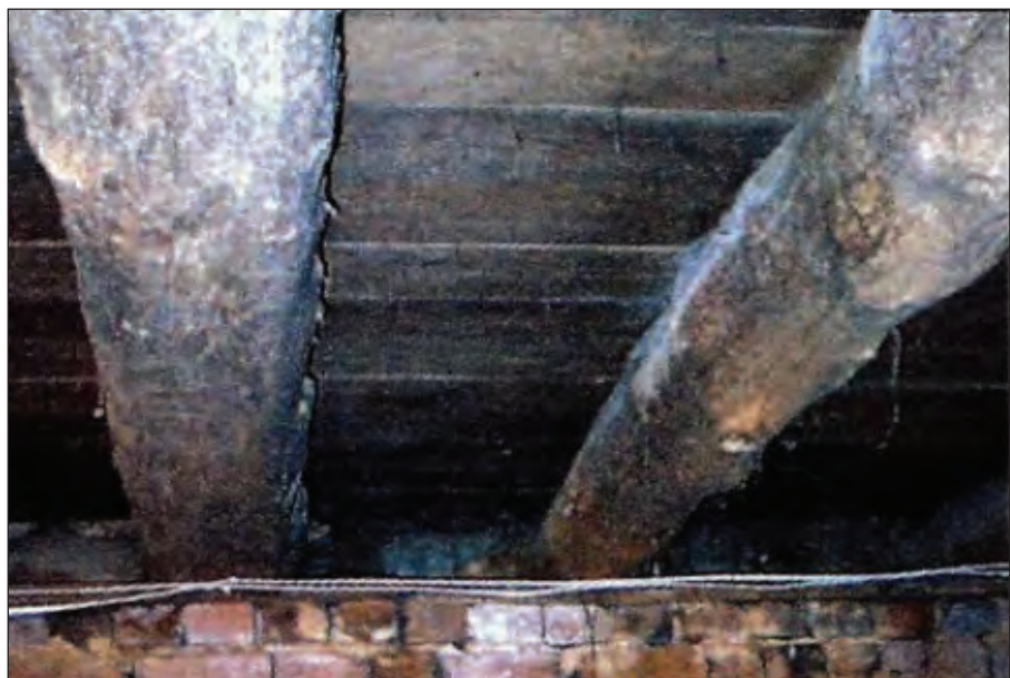
B. South Basement Wall Showing Log Beams
