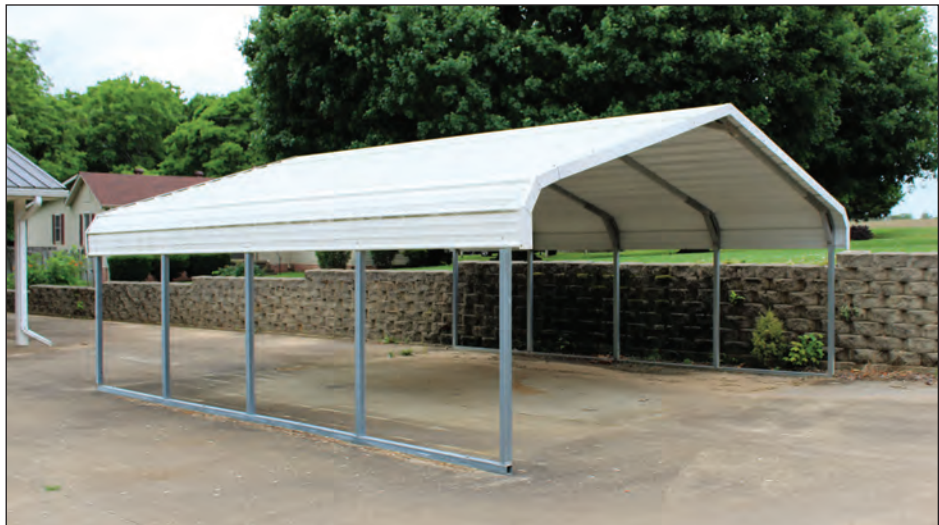
B. Carport, Looking Northeast
