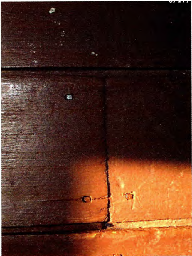
Upper level wood floor showing cut nails
