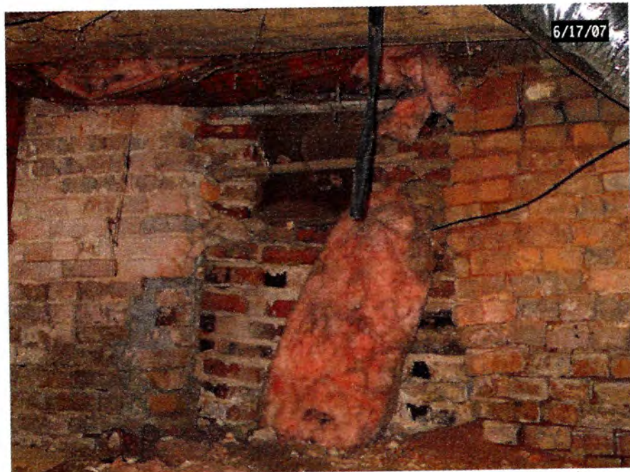
Southwest basement wall shows multiple bricks styles and previous opening.
