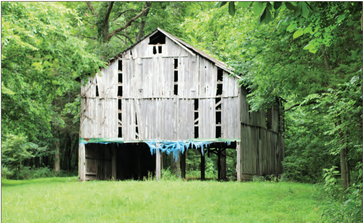
B. Abandoned Tobacco Barn, Looking West
