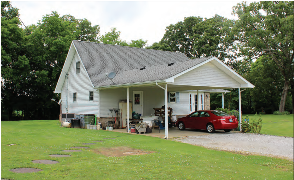
B. House, Looking Northwest
