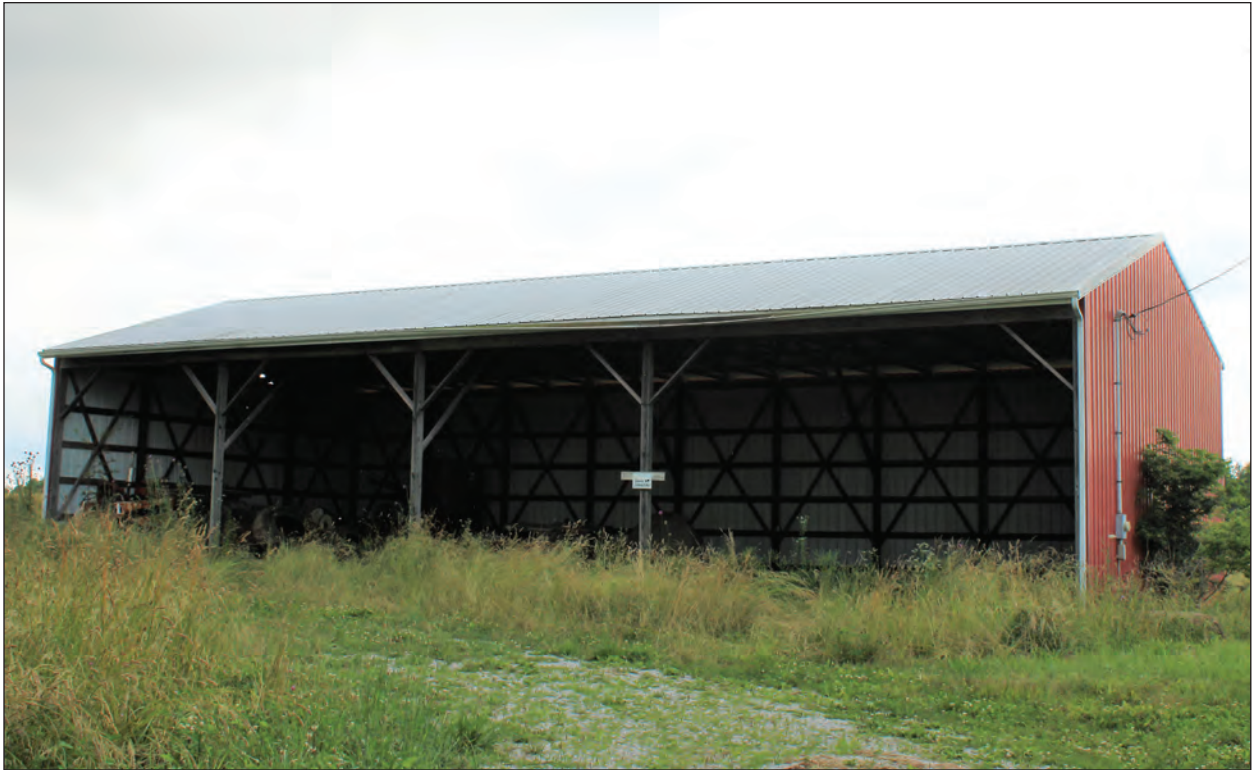
A. Equipment Shed, Looking Southwest
