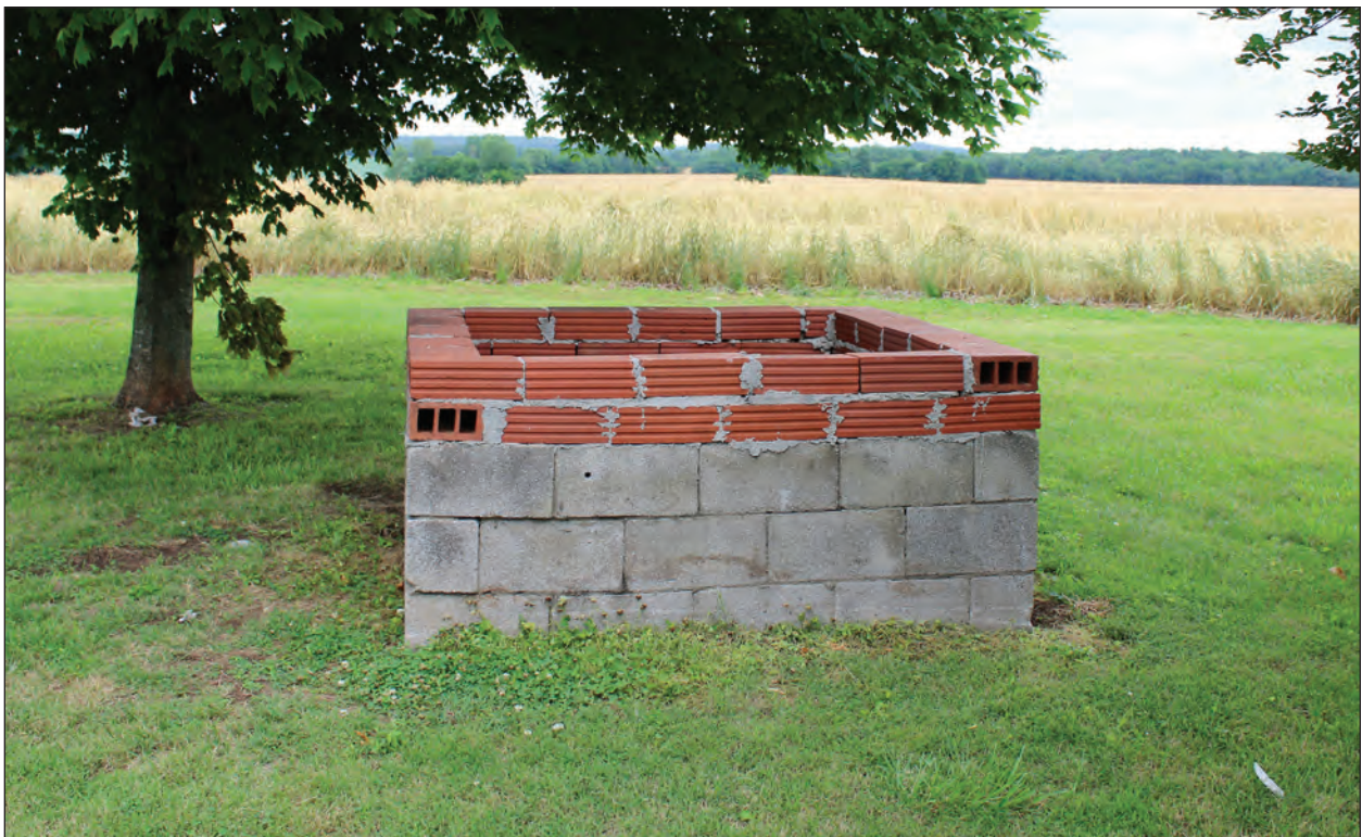
B. Utility Shed, Looking East
