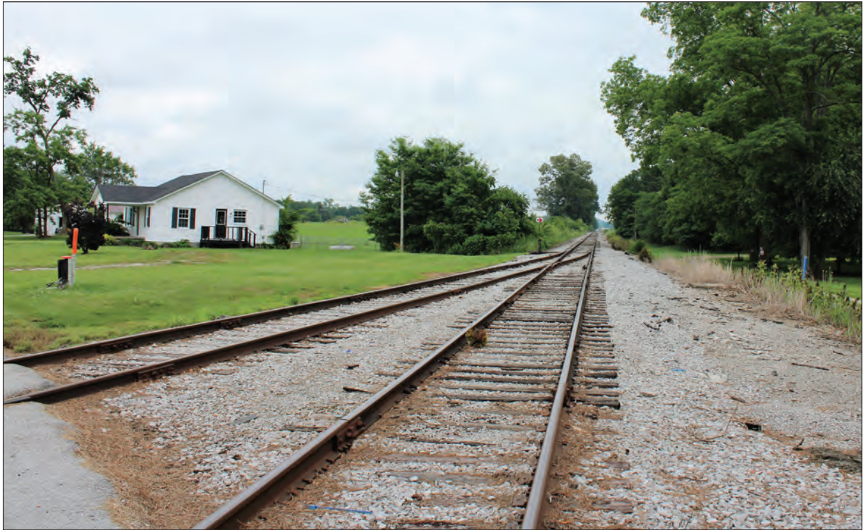
A. Looking Northeast
