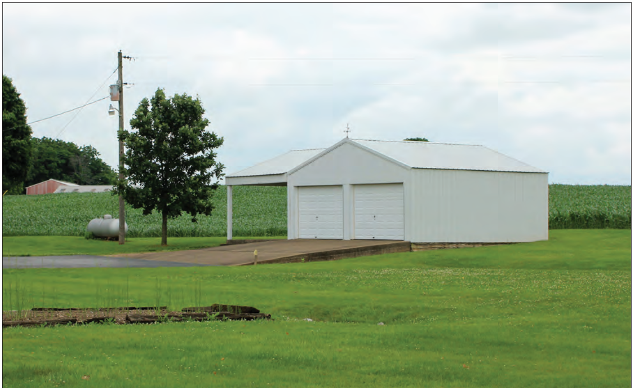
B. Garage, Looking Northeast
