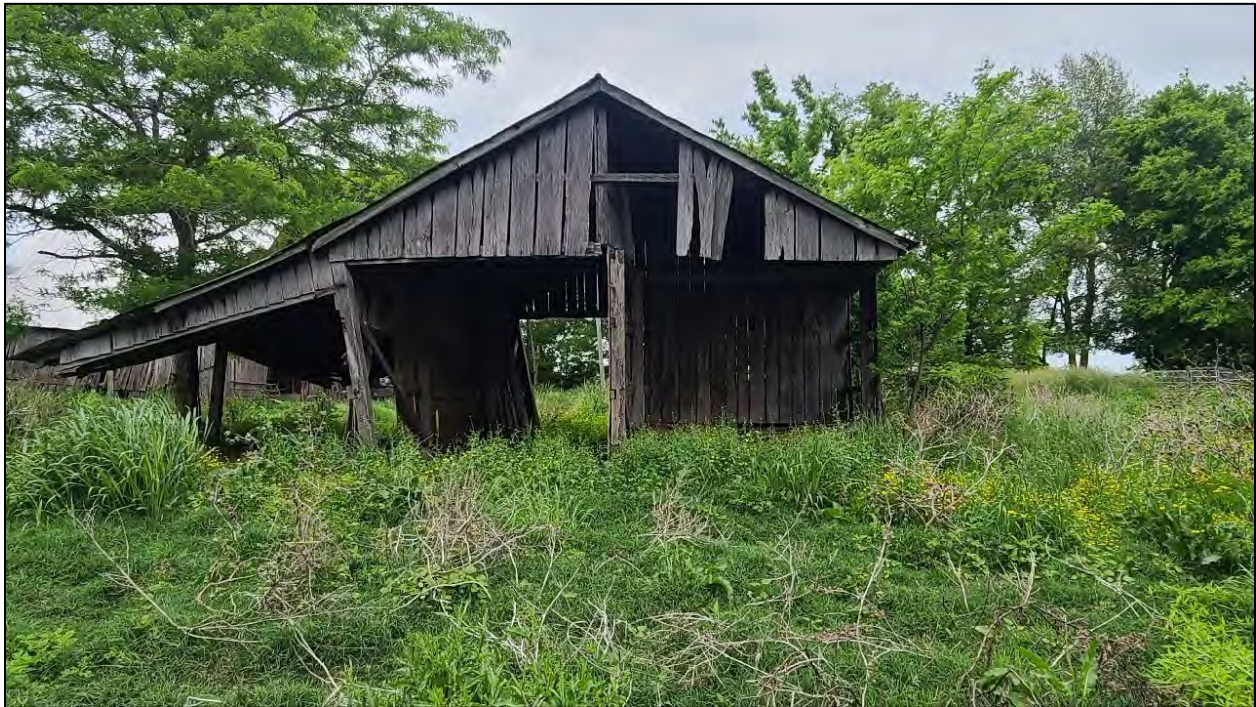
Photograph 6 – Shed on Project Area parcel 055-00-00-016-00, view to the north.
