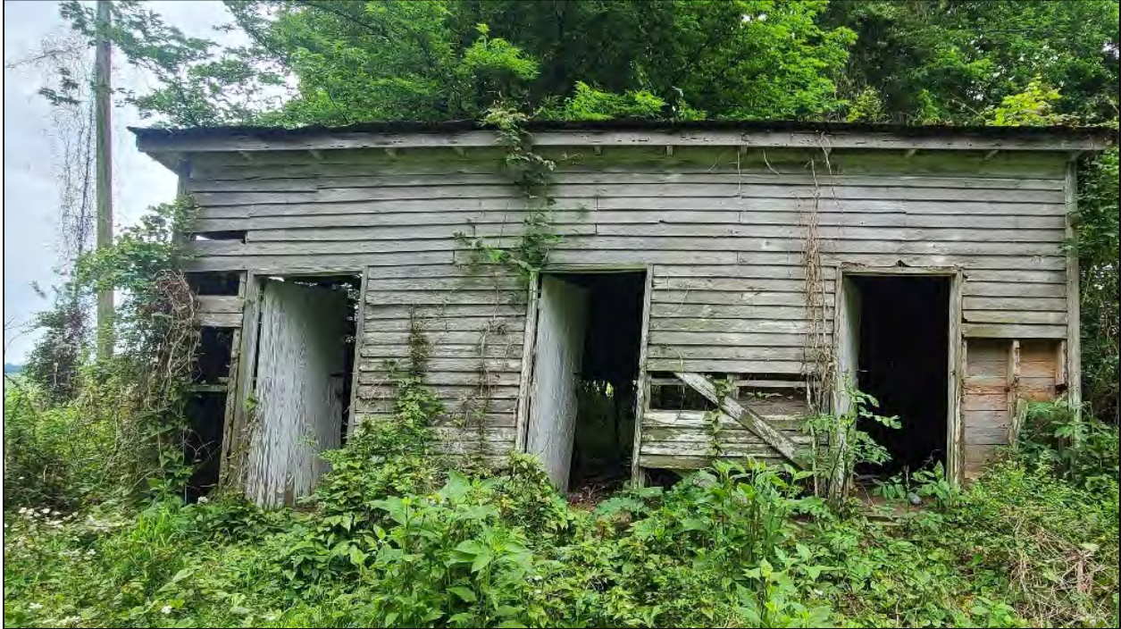
Photograph 13 – Homestead outbuilding on Project Area parcel 055-00-00-016-00, view to the east.
