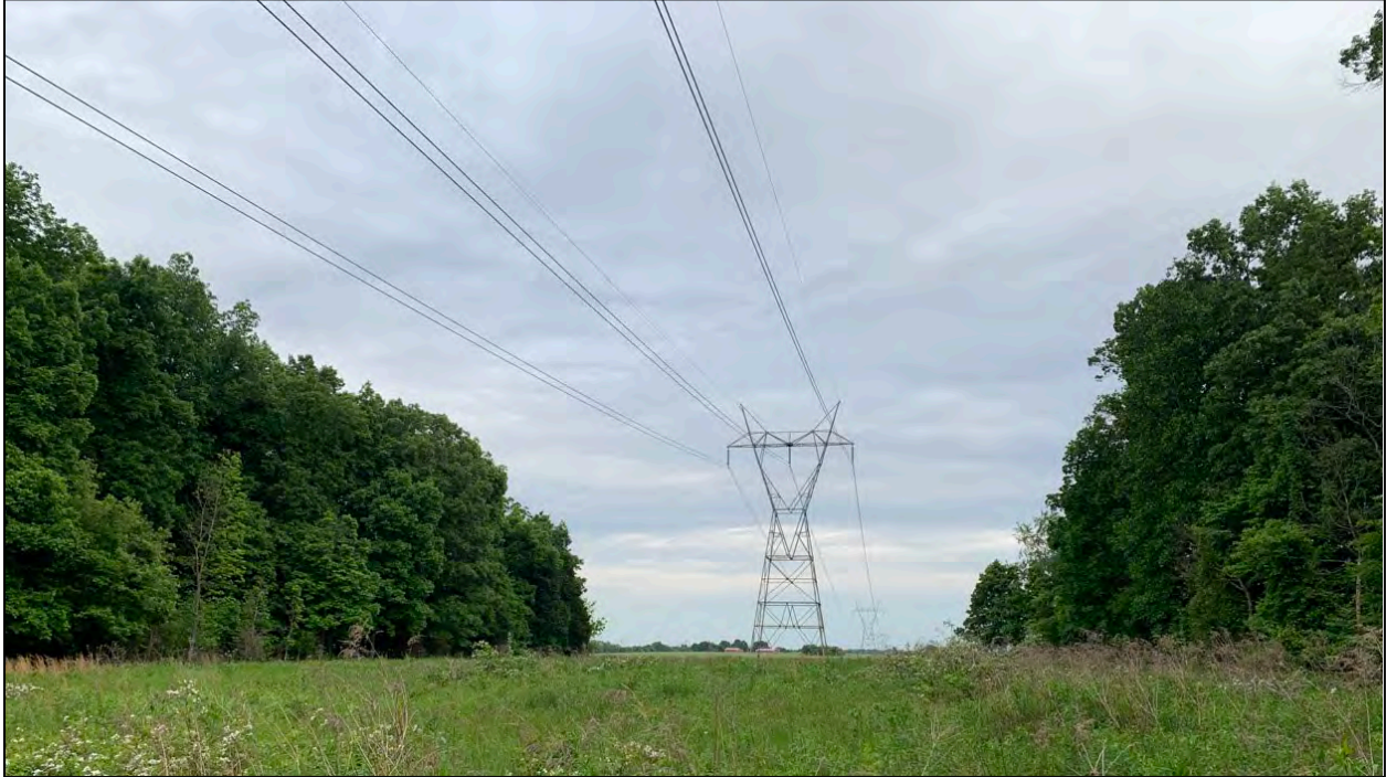
Photograph 19 – Electric utility corridor on Project Area parcel 055-00-00-016-00, view to the southeast.
