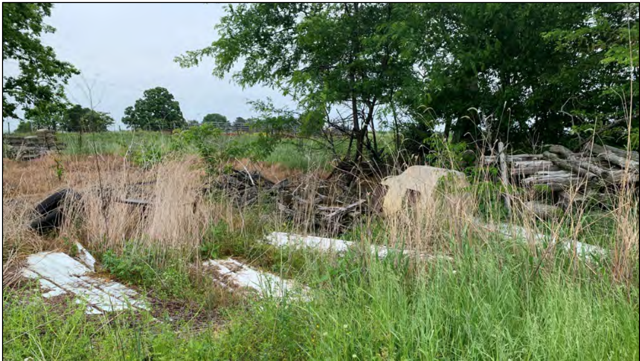
Photograph 26 – Concrete pad with bolt anchors on Project Area parcel 041-00-00-005-00, view to the southwest.
