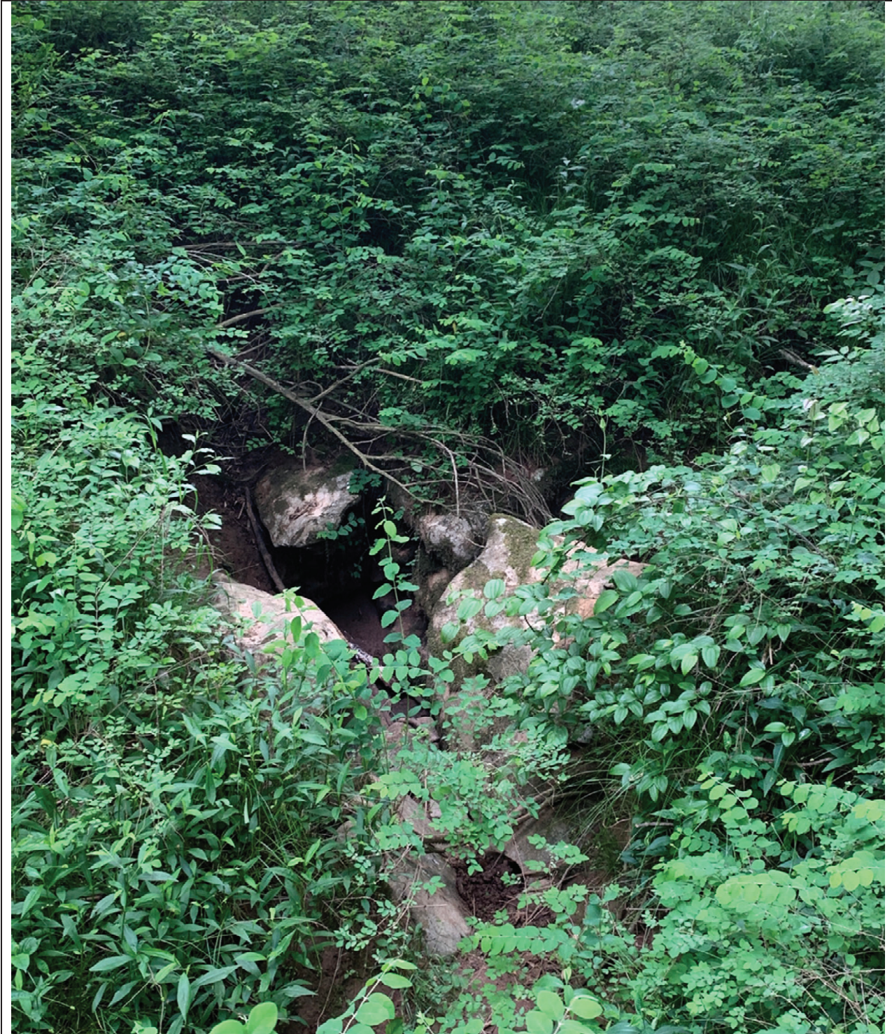
Photograph 43 – Forest stand 8, sinkhole karst fissure with limestone rock opening
