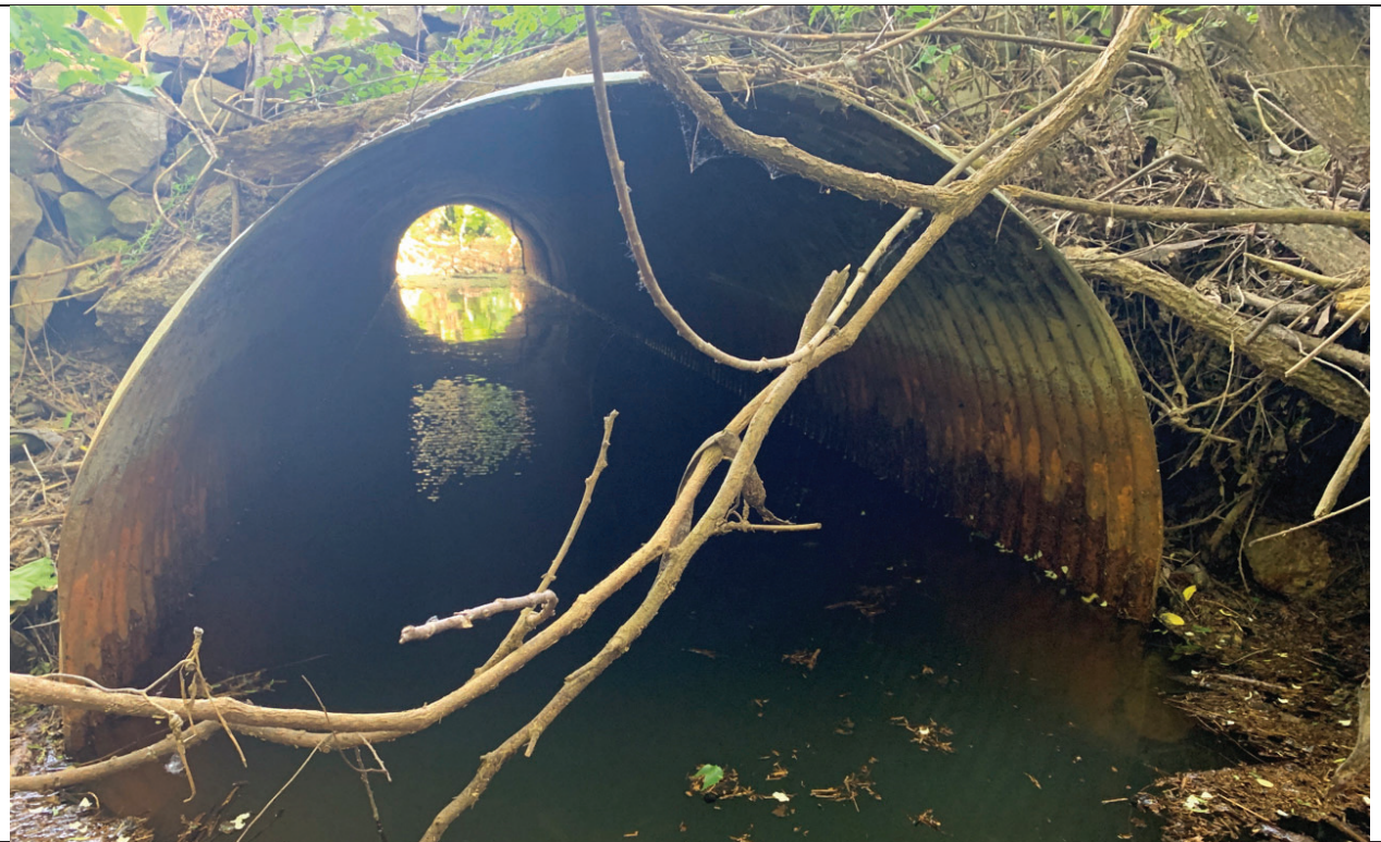
Photograph 6 – Road culvert, bat habitat, facing southeast
