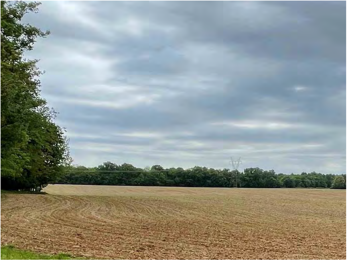
Figure C-14. Transmission line and substation area.
