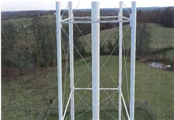
Photo shows the middle west side panel members.
