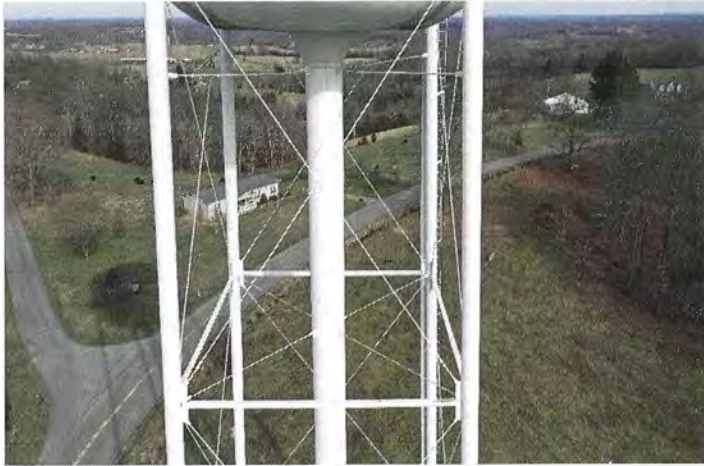
Photo shows the upper south side panel members.
