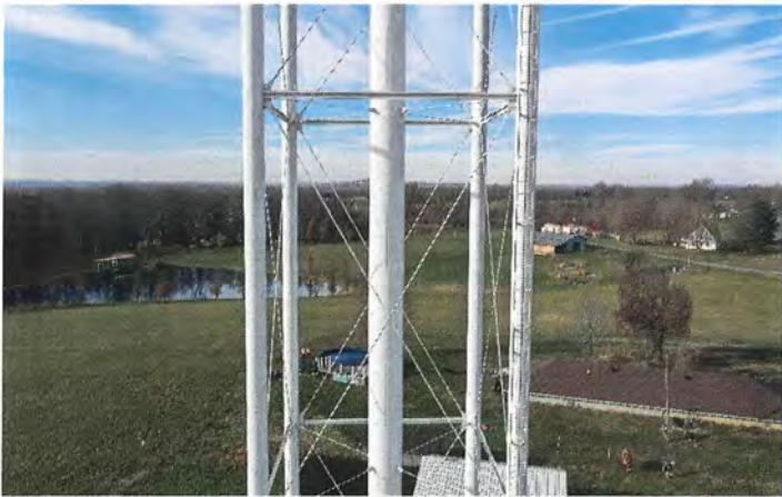
Photo shows the middle east side panel. All connections appear sound.
