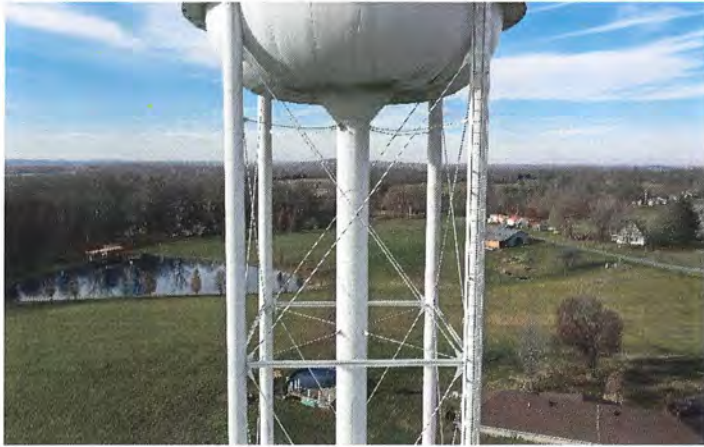
Photo shows the upper east side panel and the lower knuckle surfaces. The bowl is covered with mildew.
