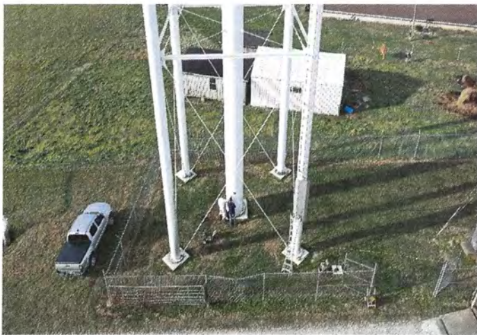
Photo shows the lower east side panel. The tank has four 24" diameter legs.
