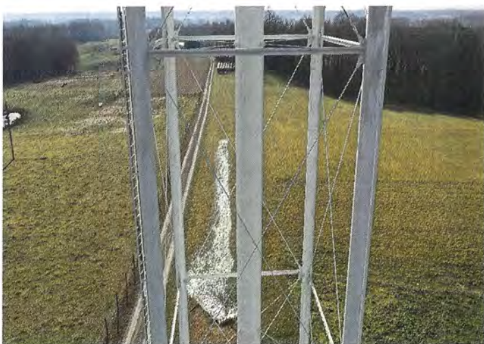
Photo shows the middle panel members on the north side.
