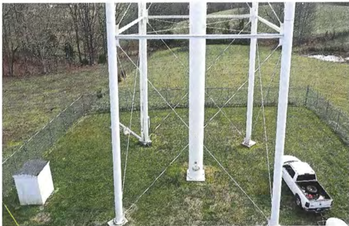
Photo shows the lower portion of the legs on the west side. The riser pipe manway is located on the west side facing the road.
