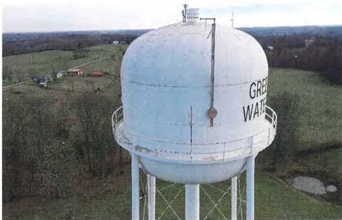
Photo shows the west portion of the shell and the level indicator.
