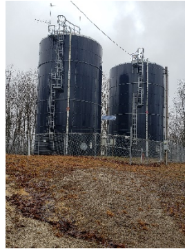
Spaws Creek (2 Tanks)
