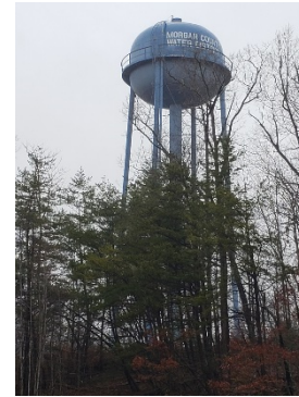
Highway 1002 Ditney Ridge Tank
