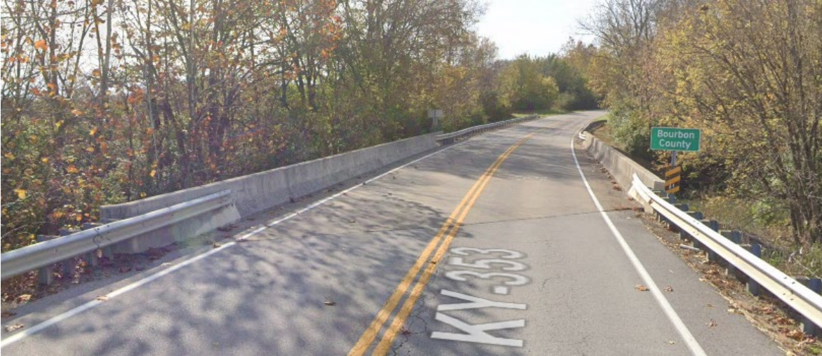
Picture (12) Bridge on KY-353
