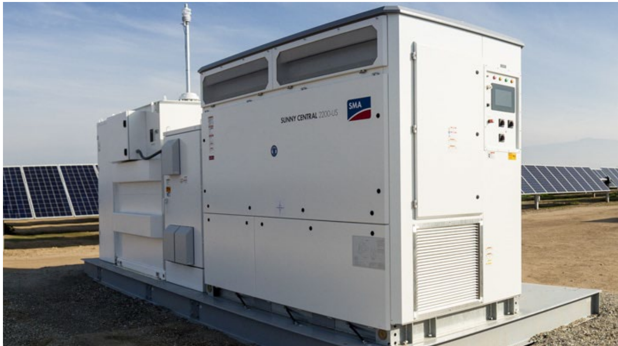
Figure (4) Industrial Solar Inverter 4
