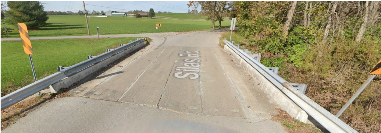
Picture (15) Bridge on Silas Road near Silas Baptist Church
