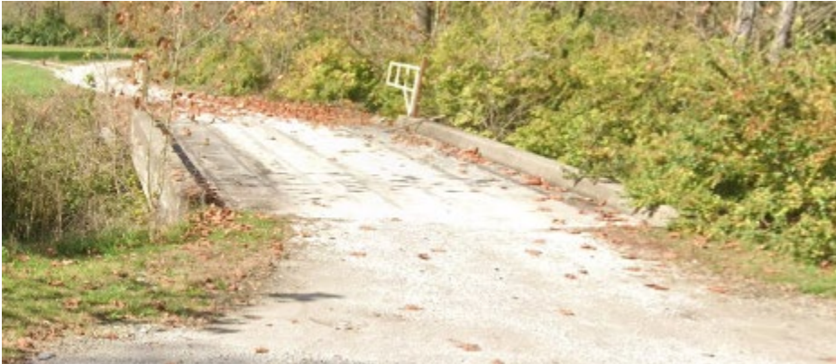
Picture (13) Culvert/Bridge for the site entrance off KY-353
