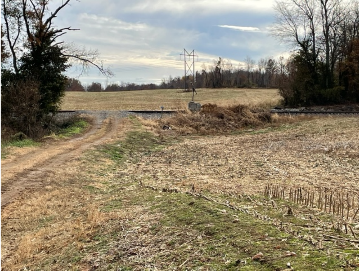
Figure C-14. Existing Grade Level Railroad Crossing in Phase 5 of the Proposed Project.
