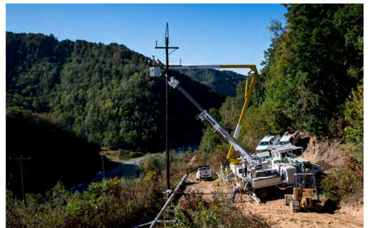
Multiple crews from the service centers work near Prestonsburg.
