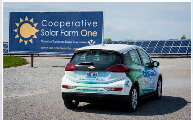
Cooperative Solar Farm One is one of Kentucky's largest sun-to-electricity projects.
