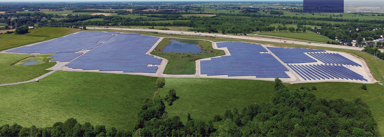
Located in Winchester along Interstate 64, Cooperative Solar Farm One is one of Kentucky's largest sun-to-electricity farms. More than 32,000 photovoltaic panels produce enough electricity to power about 1,000 Kentucky homes.
