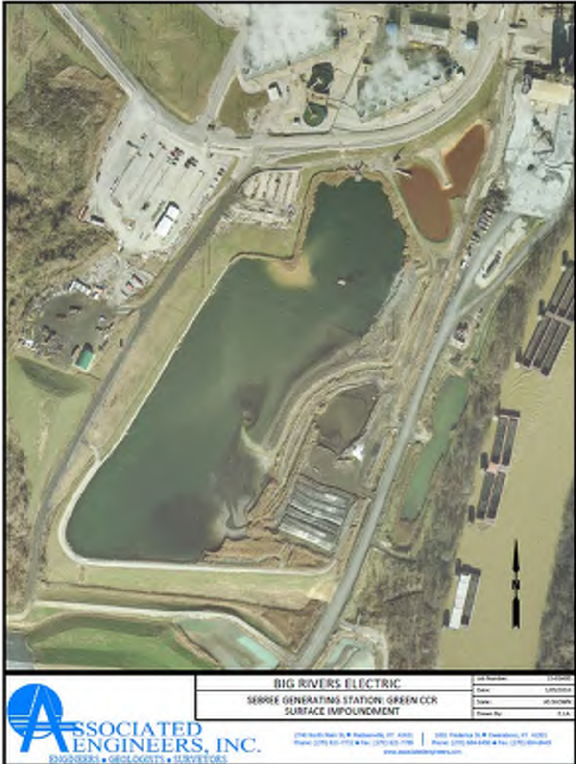
Attachment A. Aerial Photo of the Green CCR Surface Impoundment
