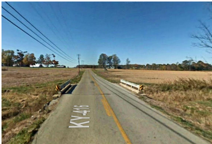
Picture (20) Culvert/Bridge on KY416
