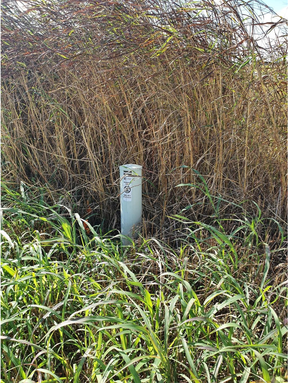
Picture (9) Existing Underground Communication line on KY283
