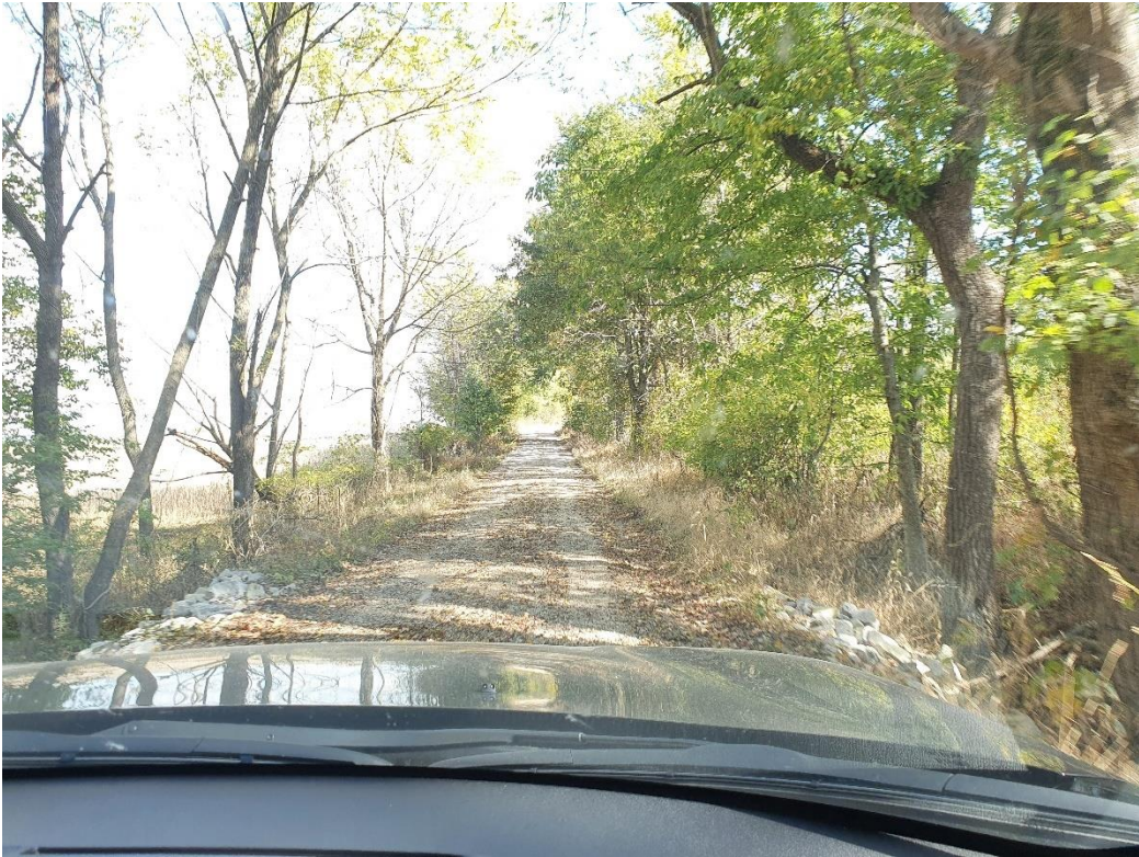
Picture (5) Location #2 – Existing gravel road
