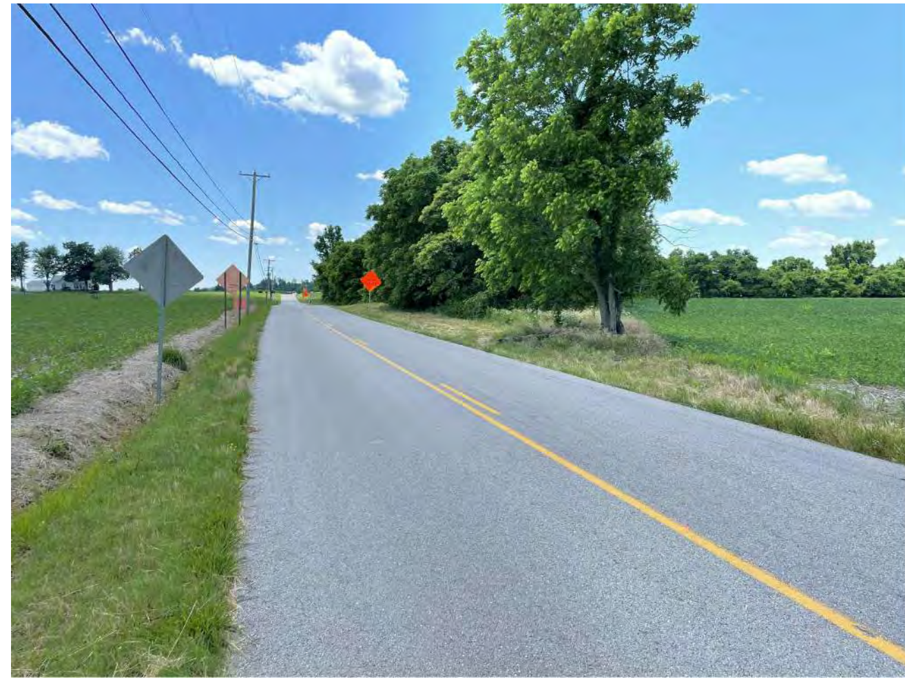
SITE ENTRANCE # 7A KY 416
