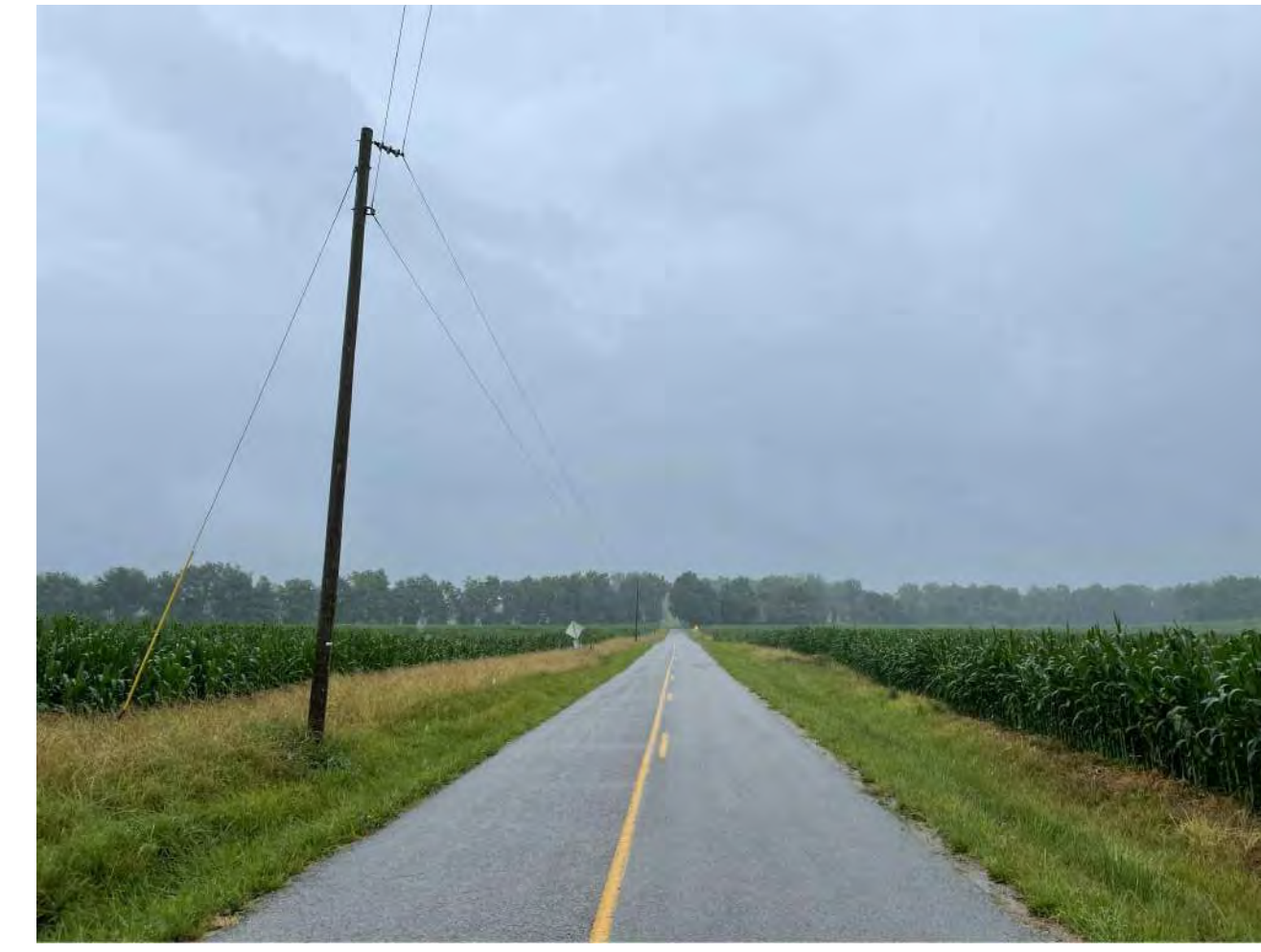
Proposed Transmission Line Crossing on KY 1299
