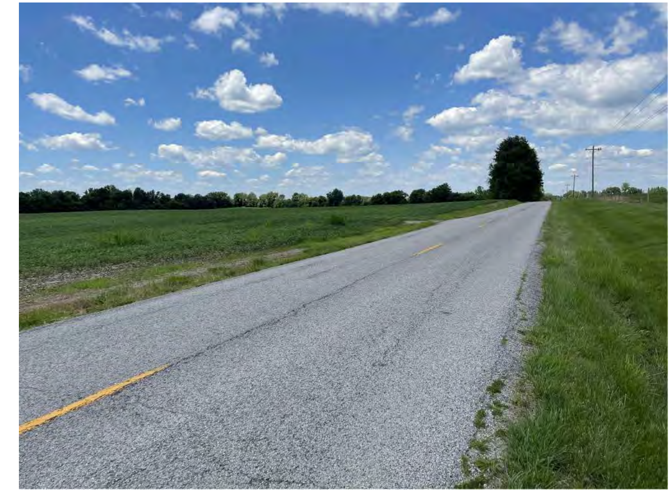
SITE ENTRANCE # 8A KY 283
