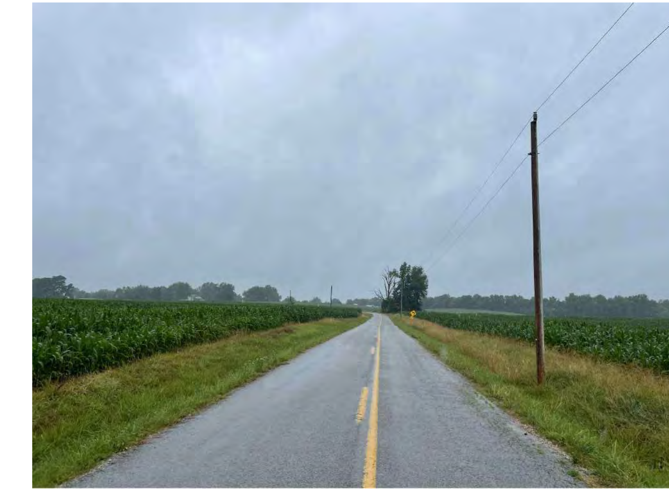
Proposed Transmission Line Crossing on KY 1299
