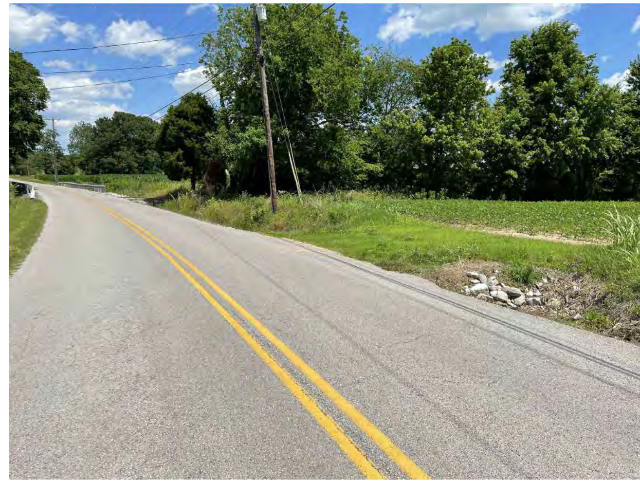
SITE ENTRANCE # 1 alt. B KY 416 (Possible future entrance evaluated for flexibility in design.)
