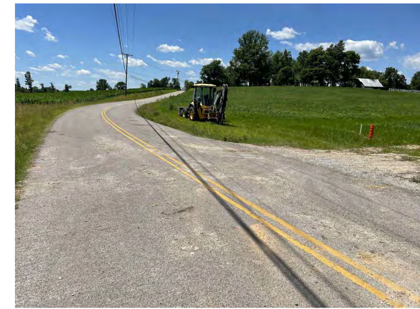
SITE ENTRANCE # 4A KY 416
