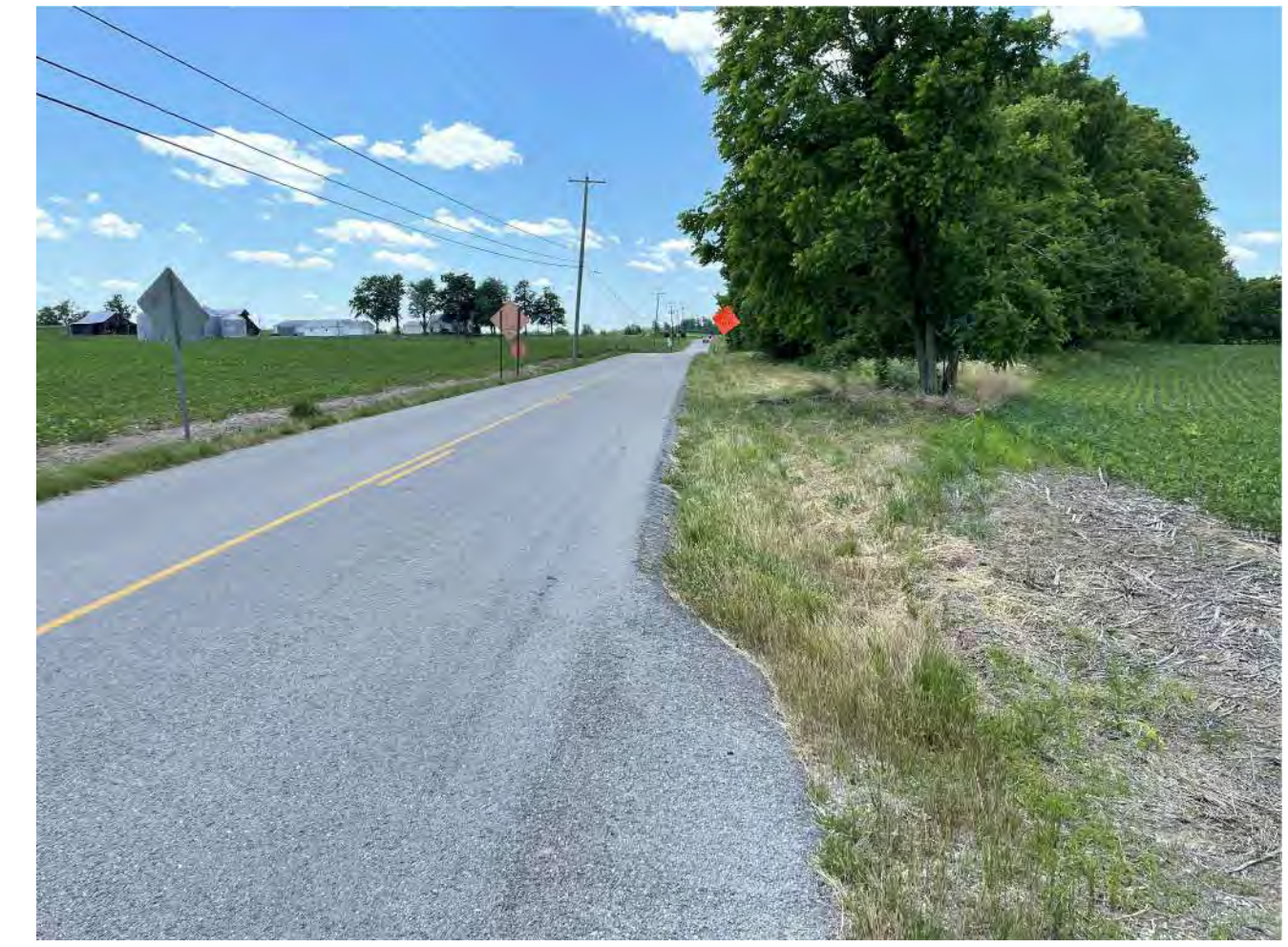
SITE ENTRANCE # 6A KY 416
