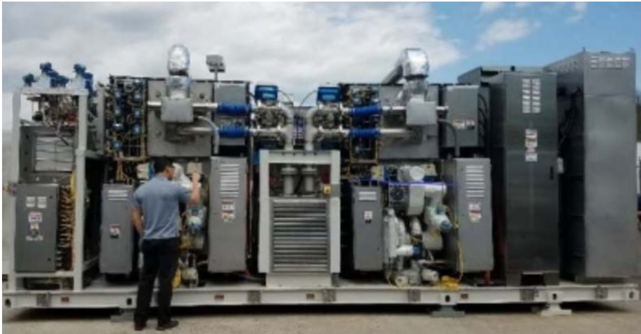
Figure 10-2 — Typical Solid Oxide Fuel Cell Project
