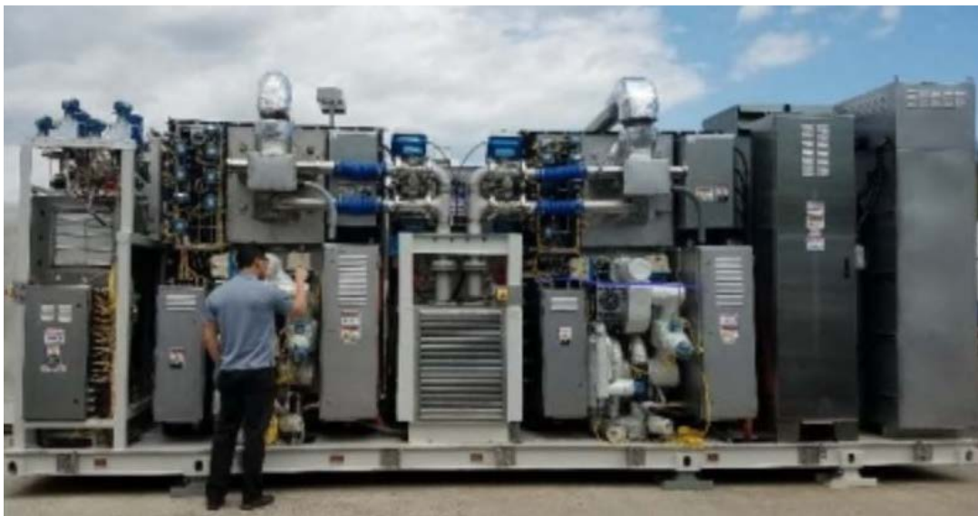
Figure 10-2 — Typical Solid Oxide Fuel Cell Project
