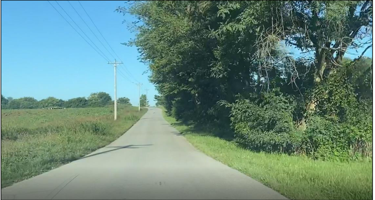
Representative Photo of Geddes Road Conditions:
