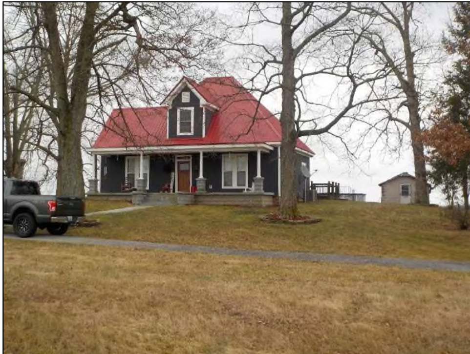
Figure 10. Resource No. SI 130, facing northeast.
