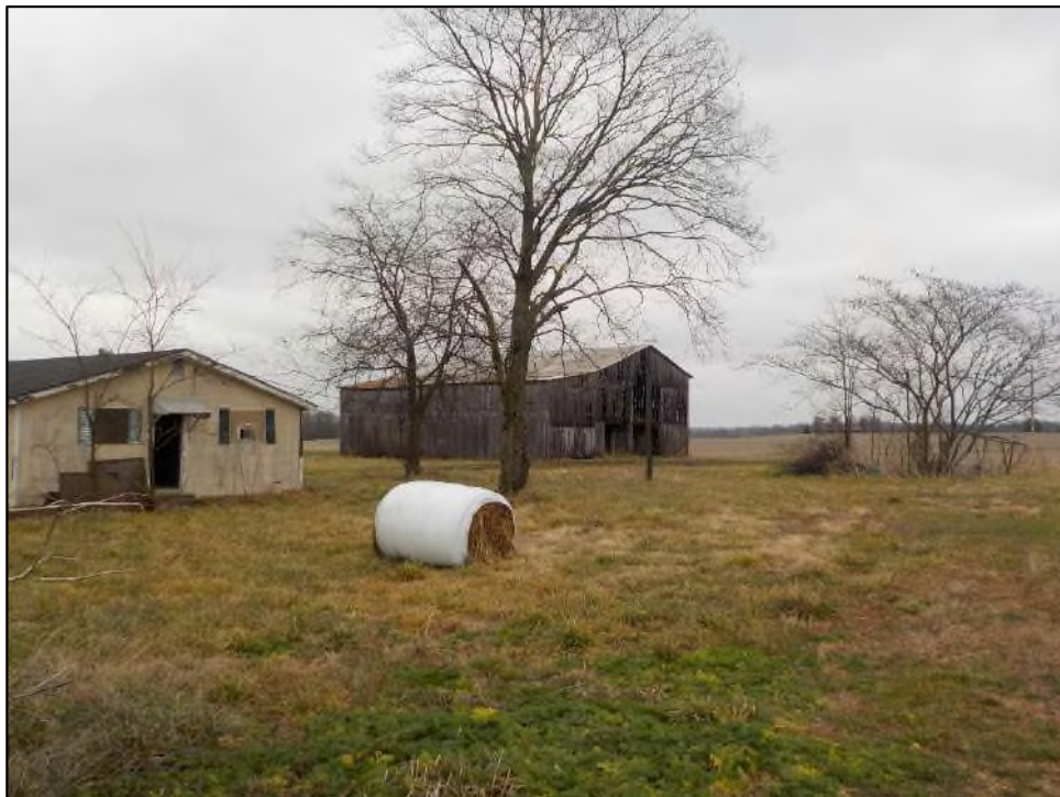
Figure 13. Resource No. SI 138, facing northeast.
