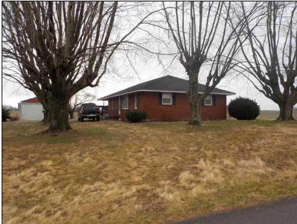
Figure 17. Resource No. SI 138, facing northeast.
