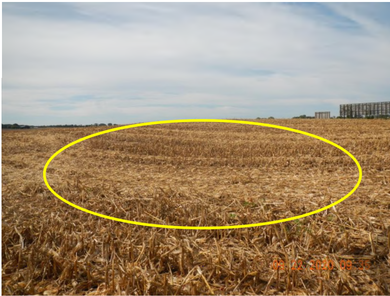
Figure 18: View of feature F-59, small, gentle sloped cover subsidence sinkhole with no open throat observed.
