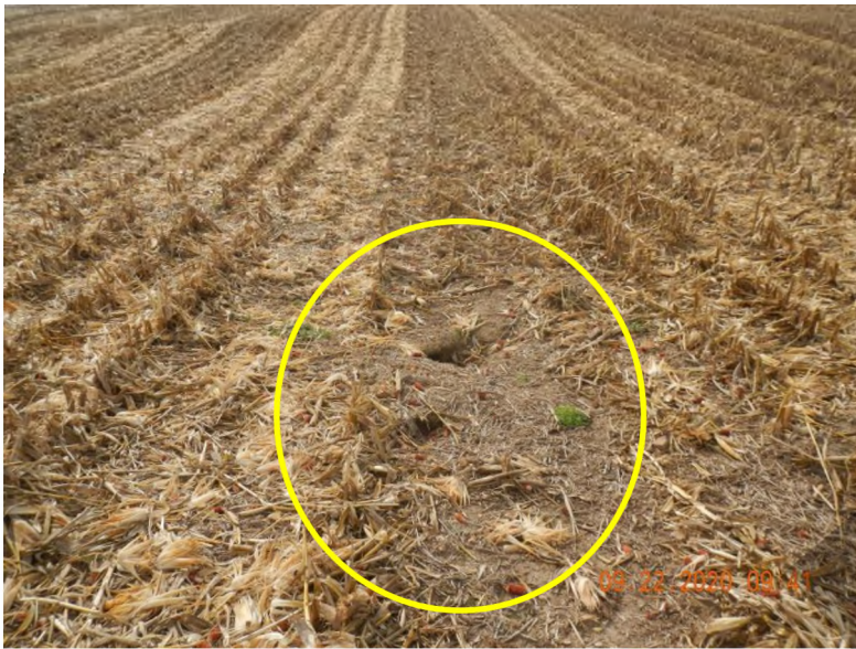
Figure 6: View of feature F-60, soil piping on central portion of parcel.
