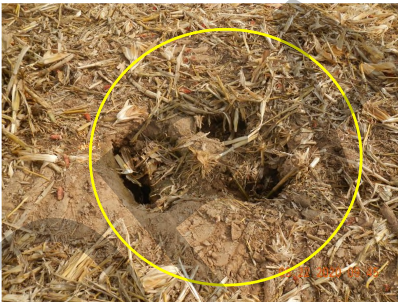
Figure 7: View of feature F-61, soil piping on central portion of parcel.
