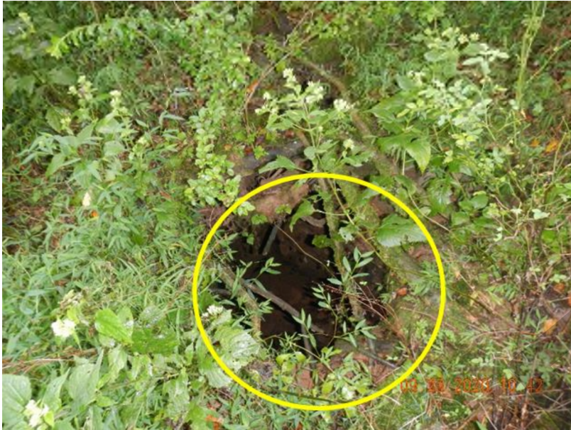
Figure 26: View of feature F-79, cover-collapse feature, open throat observed.
