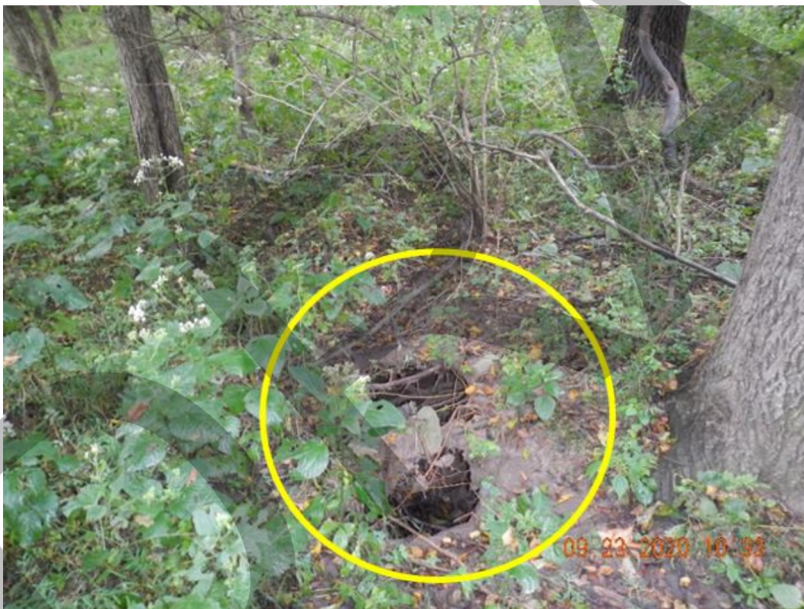
Figure 25: View of feature F-78, multiple soil piping features in one area.
