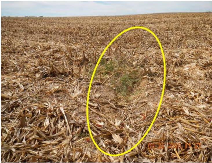
Figure 22: View of feature F-68, erosion Rill and surface drainage pathway on central of the parcel. No open throats or soil piping was observed.
