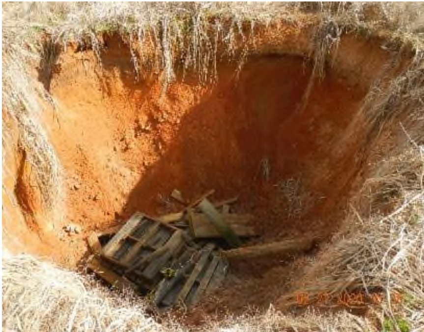
Figure 2: View of feature F-4, sinkhole filled with debris located on the west side of the project site
