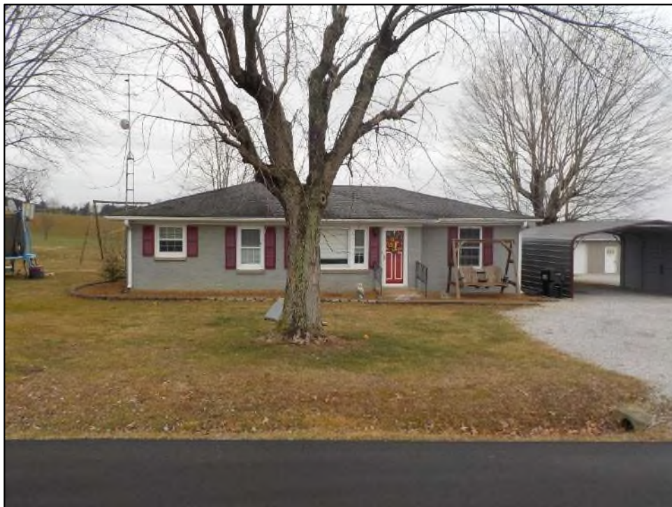
Figure 47. Resource No. SI 531, facing west.
