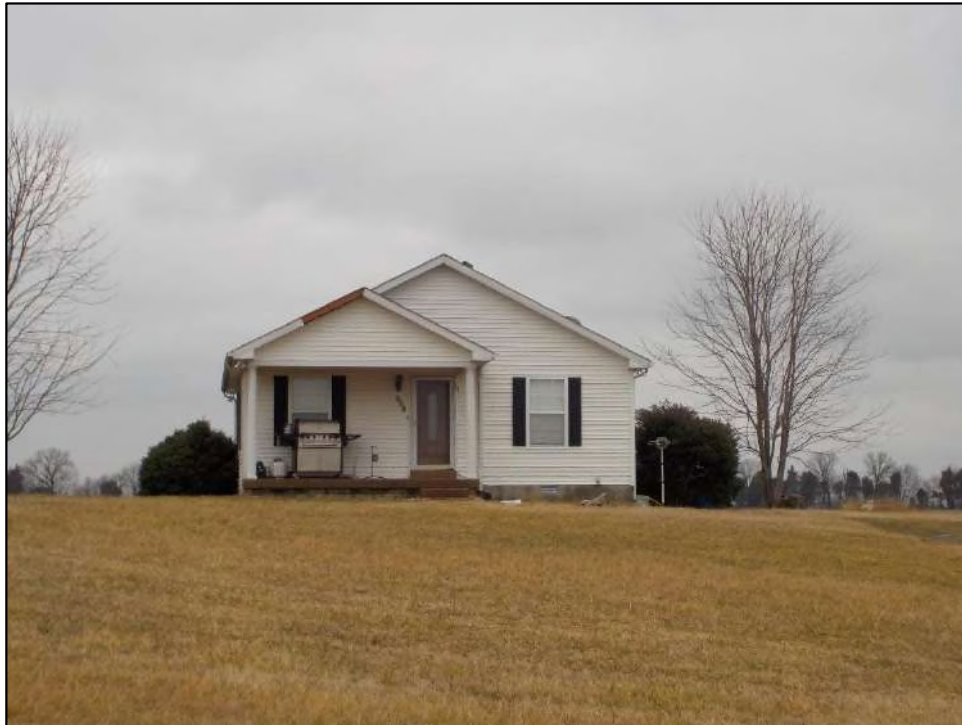
Figure 52. Resource No. SI 535, facing west.
