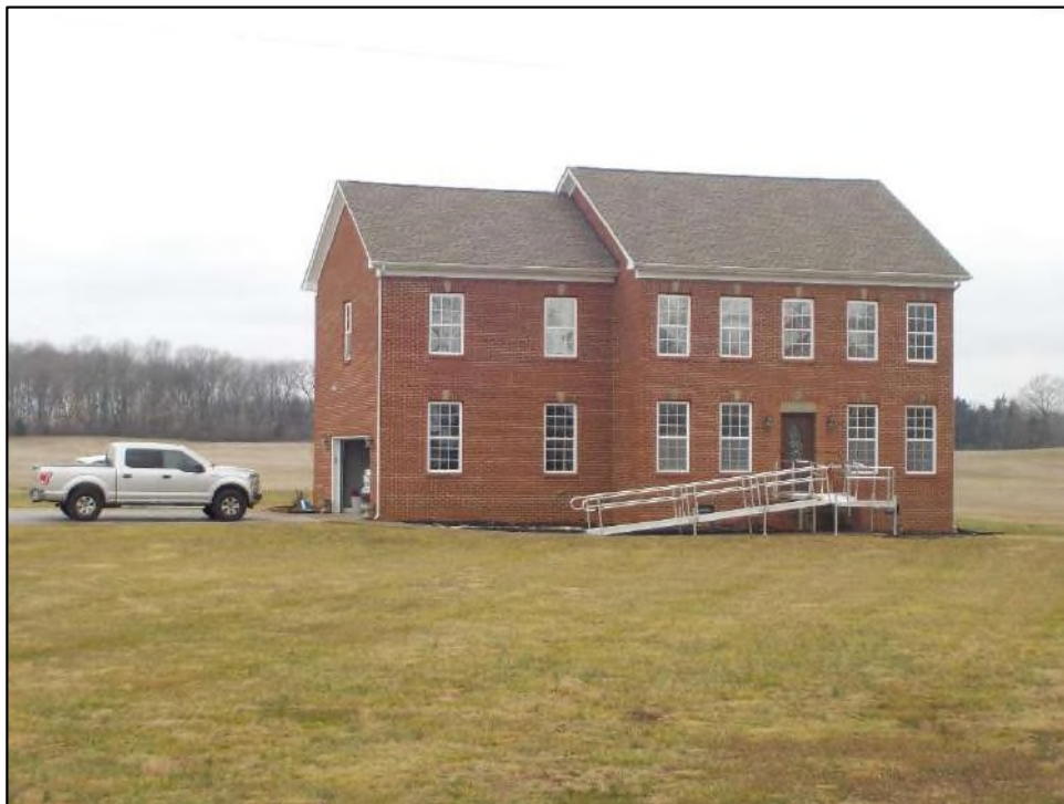
Figure 51. Resource No. SI 533, facing northwest.
