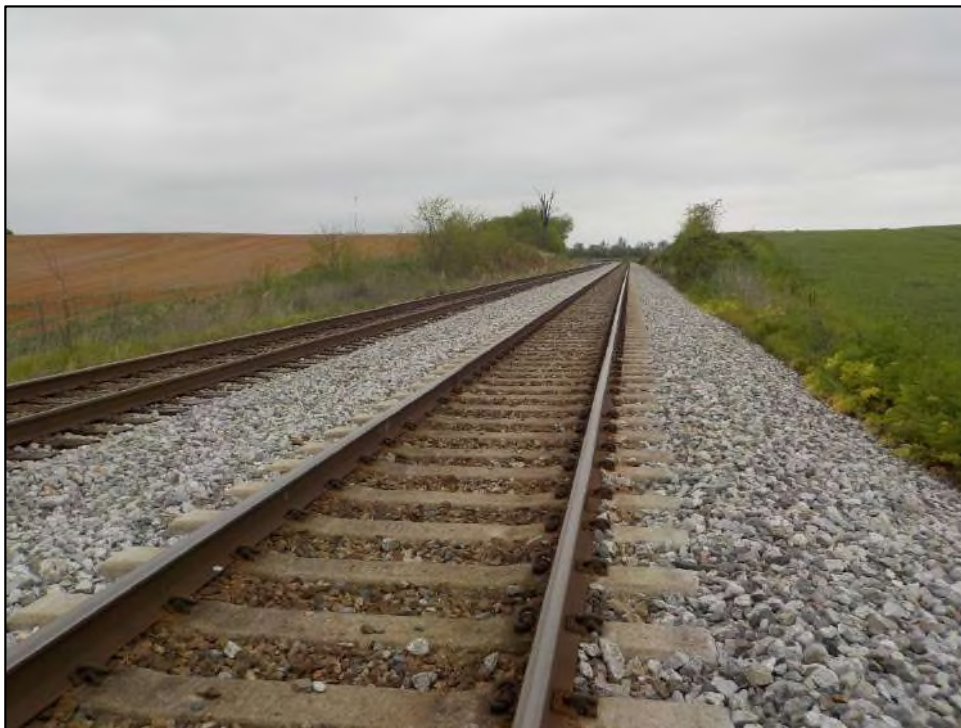
Figure 55. Resource No. SI 537, facing north.
