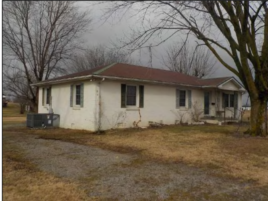
Figure 33. Resource No. SI 522, facing northwest.
