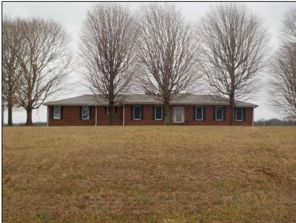
Figure 45. Resource No. 529, facing east.
