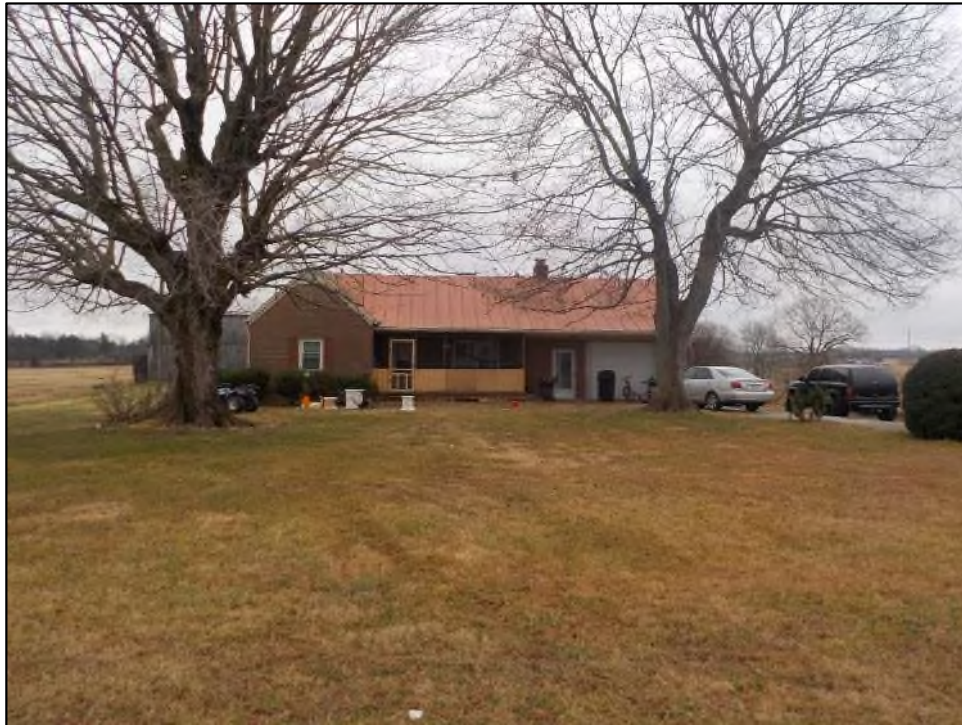
Figure 26. Resource No. SI 518, facing west.
