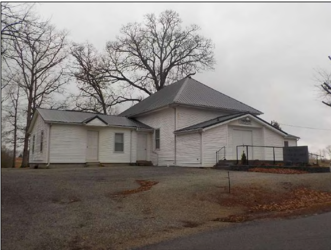
Figure 28. Resource No. SI 519 - Tyree Chapel Church of Christ, facing northwest.
