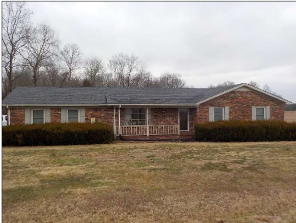
Figure 46. Resource No. SI 530, facing north.
