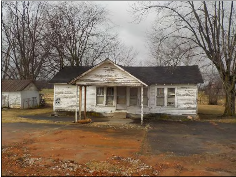
Figure 35. Resource No. SI 523, facing west.
