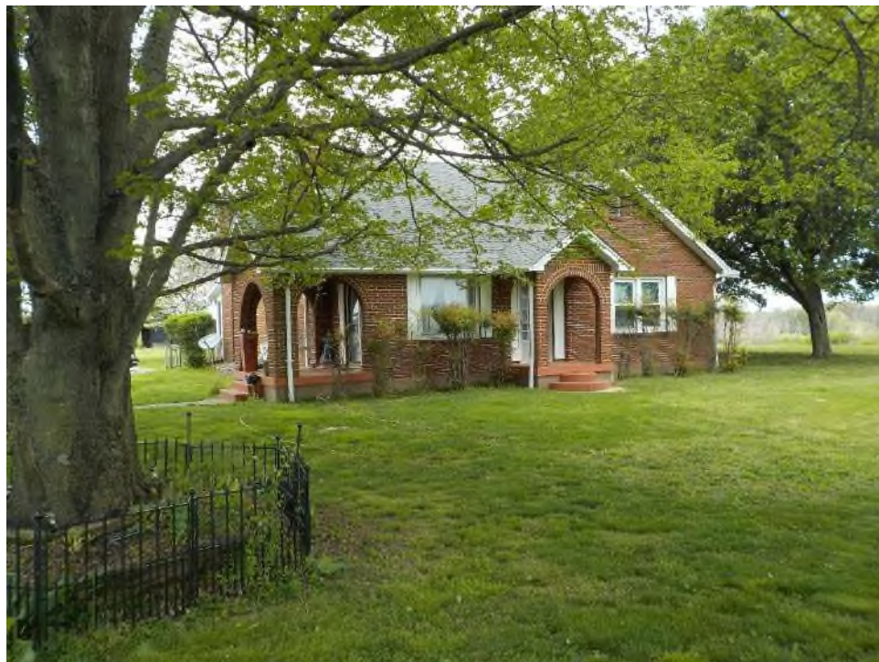
Figure 32. Resource No. SI 520, facing north.
