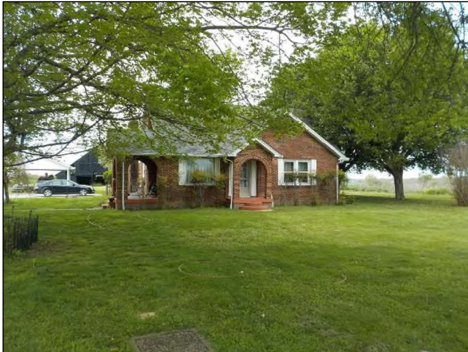
Figure 31. Resource No. SI 520, facing northwest.
