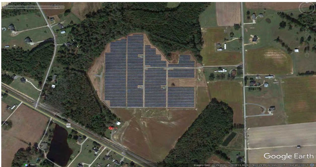
This solar farm is located at 4839 US 70 Highway just east of Herring Road. This solar farm was completed on October 25, 2016.
