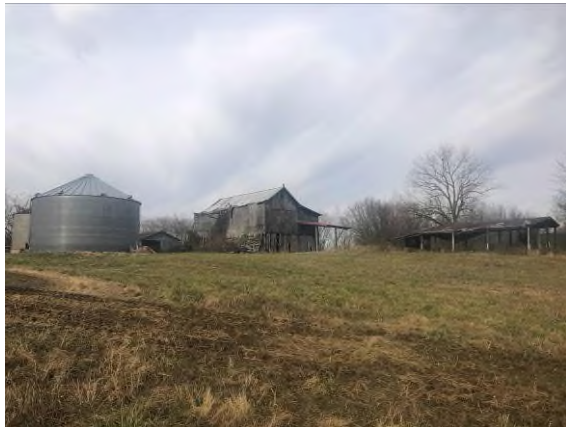
Photo #3 View of southeastern portion of site of site, and structures east of Tyree Chapel Road - facing northwest.
