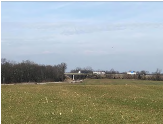
Photo #33 View of southwestern portion of site, adjoining railroad tracks, and adjoining I-65N - facing northwest.
