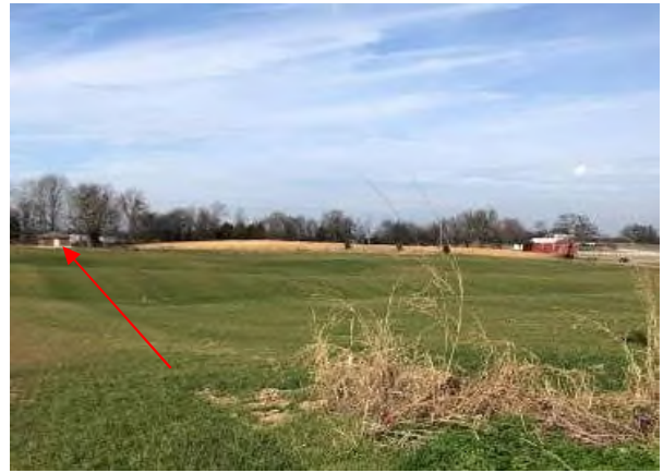
Photo #50 View of northwest portion of site, apparent offsite booster pump station (arrow), and adjoining property north of Old County Farm Road - facing north.
