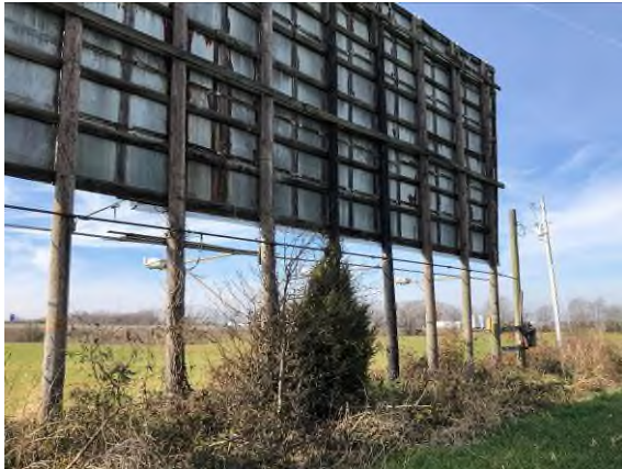
Photo #49 View of northwest portion of site, billboard, and electrical transformer - facing north.
