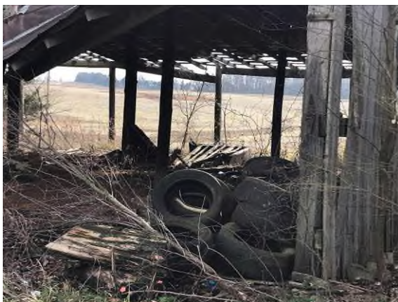
Photo #17 View of southeastern portion of site, and interior of structure east of Tyree Chapel Road - facing southeast.
