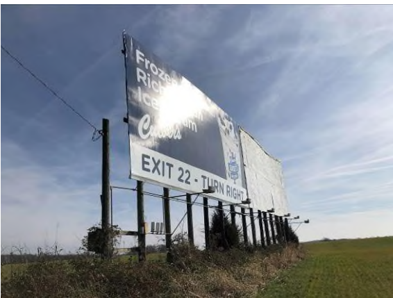
Photo #47 View of northwest portion of site, east billboard with lights - facing south.
