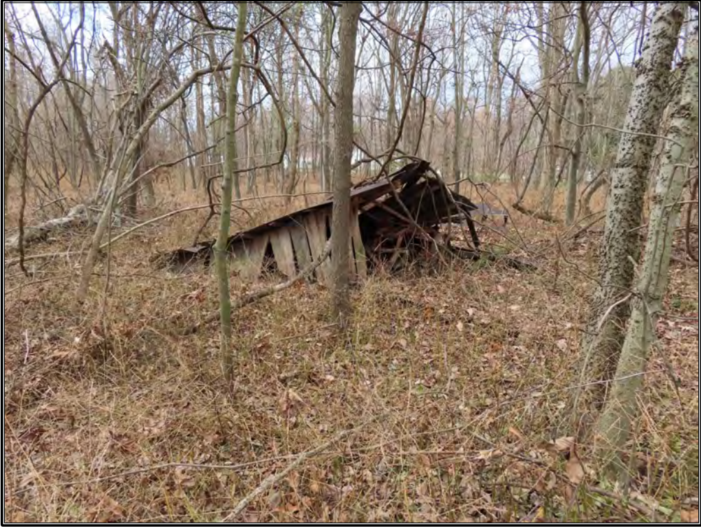
Figure 22. Collapsed shed near the location of MS 14, facing southwest.
