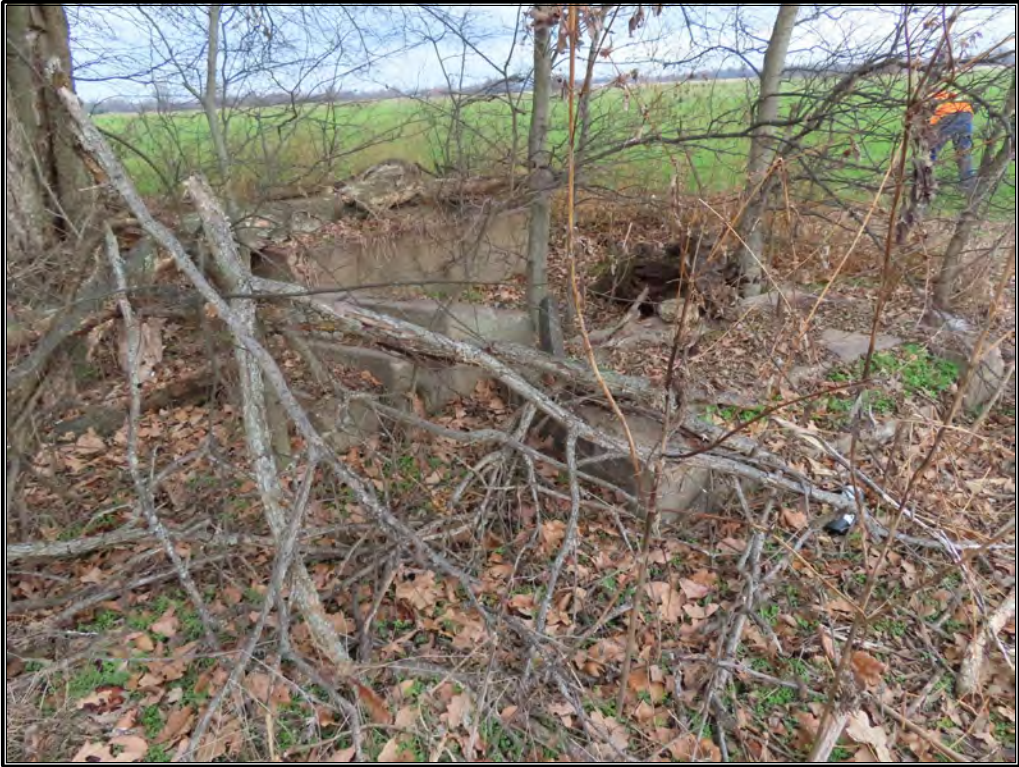
Figure 21. Concrete steps in the location of MS 6, facing northwest.
