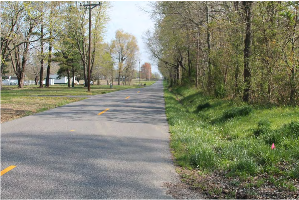
Figure 6 (MC 6) Access on KY 725 at Burney School Road (Looking North)
