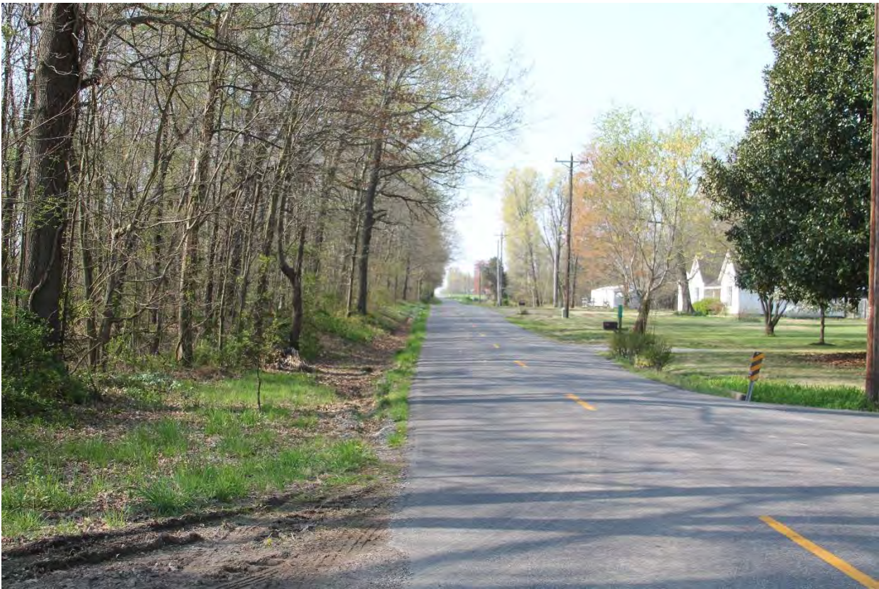
Figure 5 (MC 5) Access on KY 725 at Burney School Road (Looking South)
