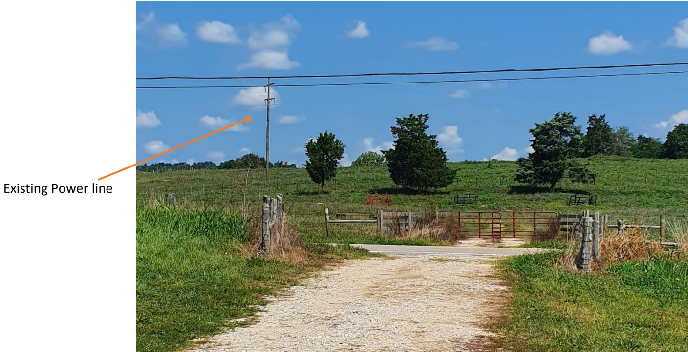
Picture (11) Location #7 – Big Rivers 69kV Interconnection
