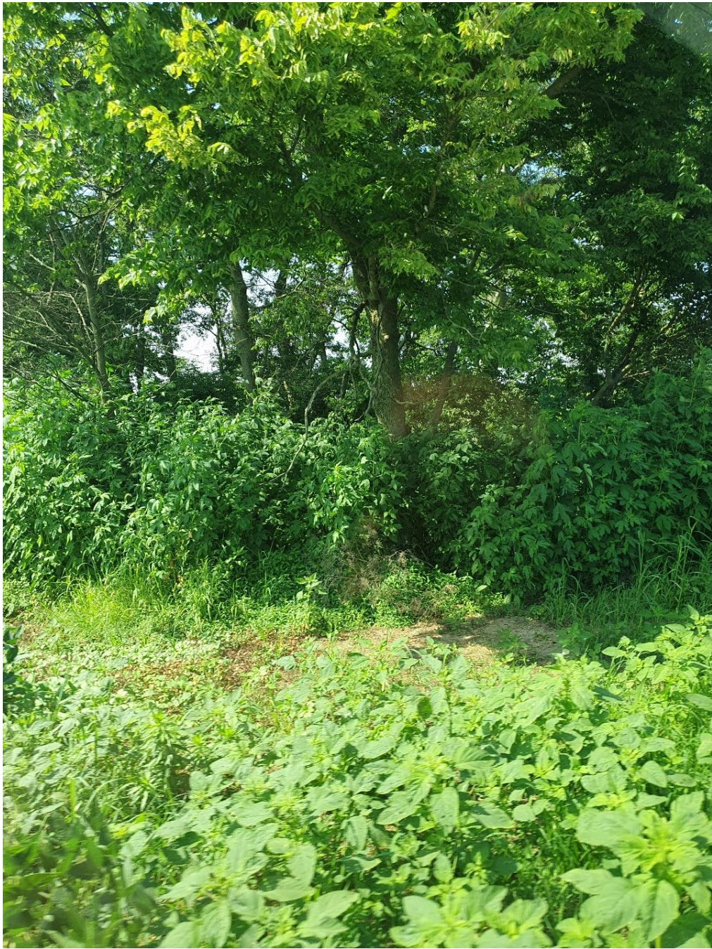
Picture (4) Location #2 – Sinkhole
