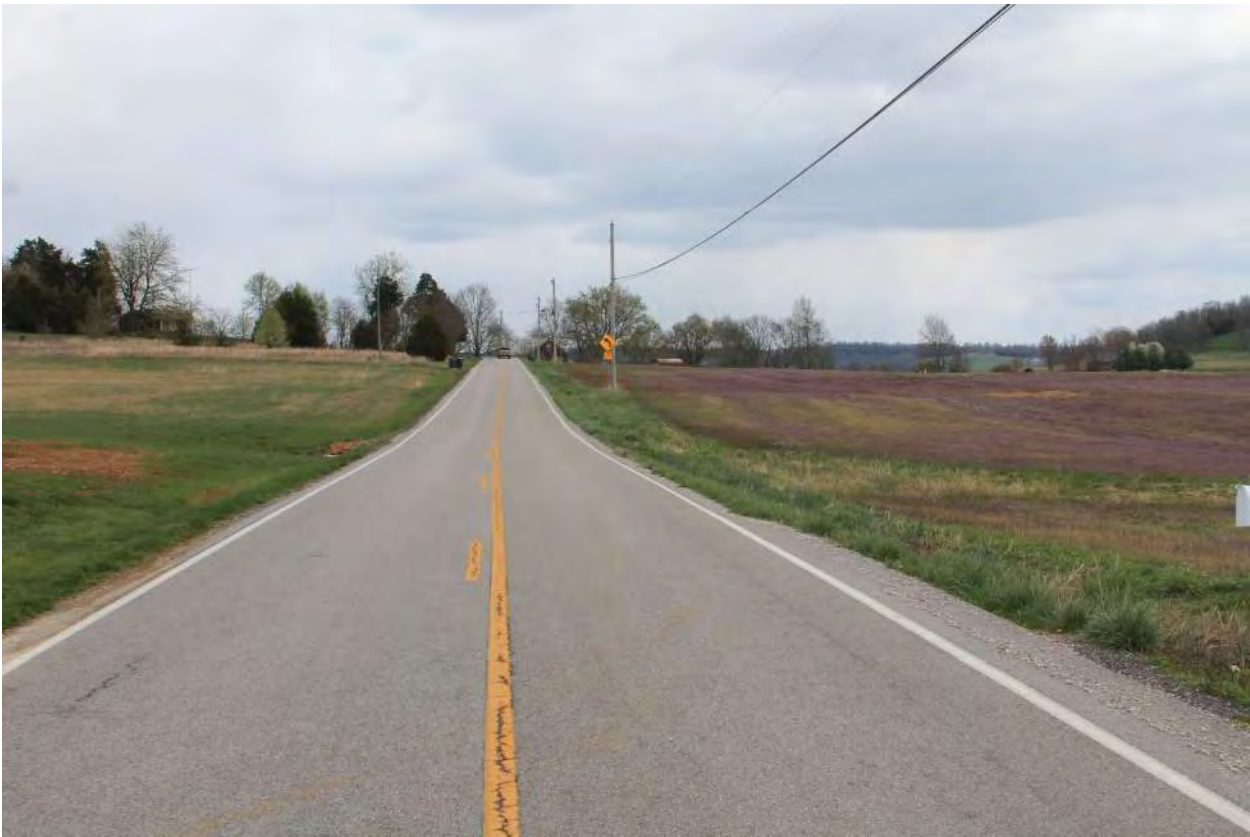
Figure 4 Meade Co Access Location on KY 1238 (Looking East)
