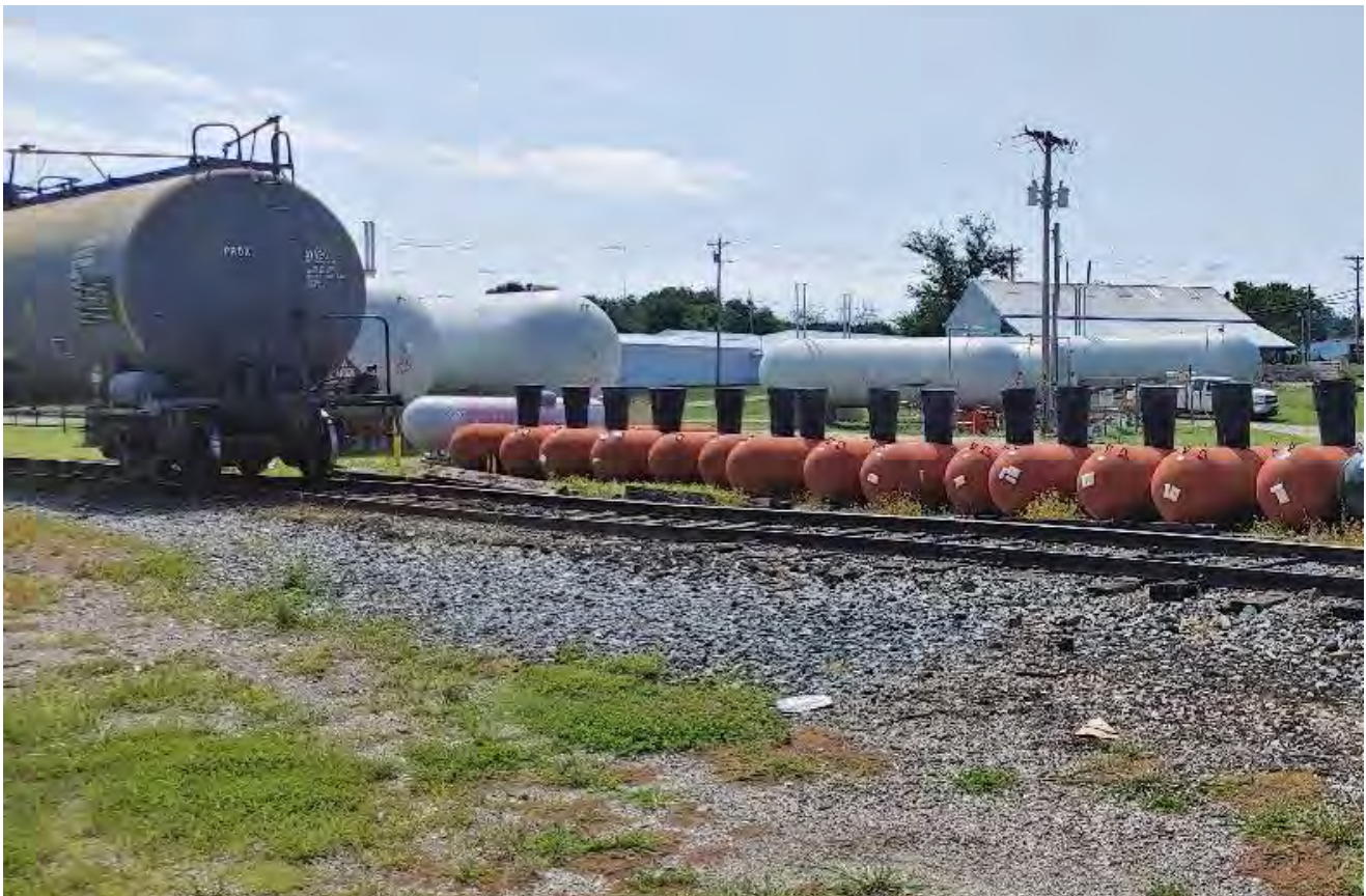
Photo 10: Railroad tracks running through the southern portion of the Site.
