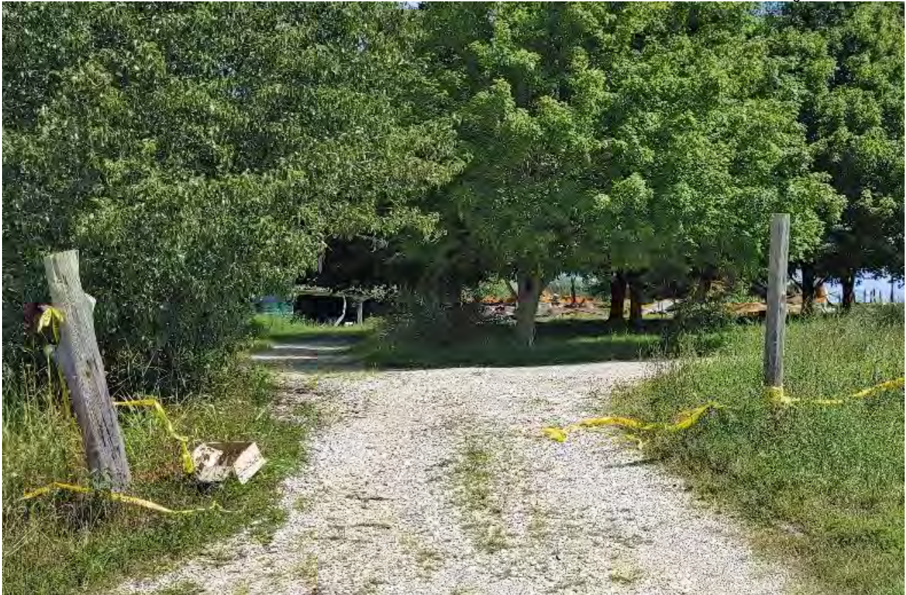
Photo 9: Collapsed house on adjoining property west of Parcel 19.
