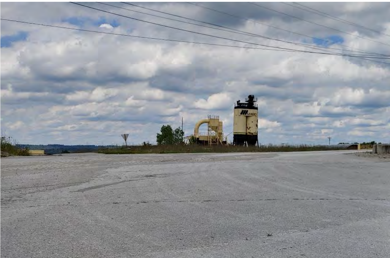
Photo 2: Adjoining asphalt plant located near the Mago Construction Co LLC north of Parcel 6.
