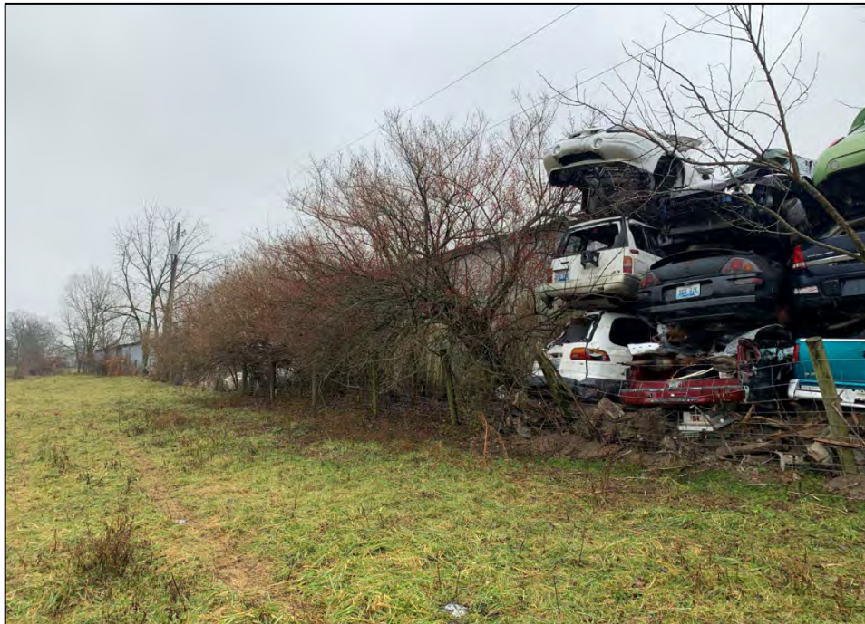
Photo 16: View of adjacent junkyard auto-shop along Old Convict Pike with transformers. View from southern Site boundary, facing east.
