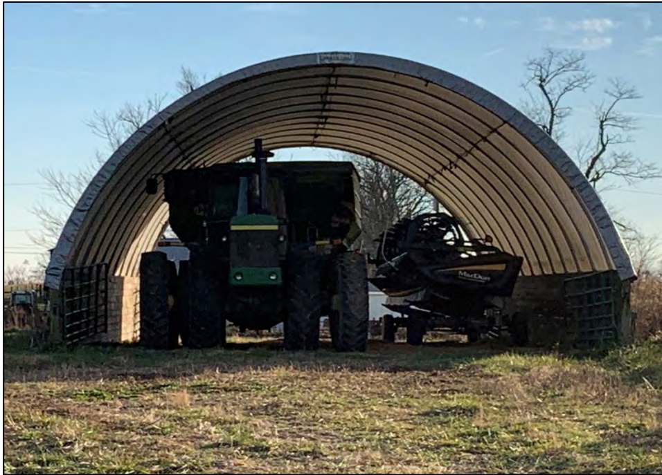
Photo 9: View of the hoop shed (Figure 2, Feature ID 11) with tractor, facing north.
