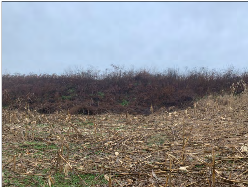
Photo 46: View of Pond 10 berm from the lowest downgradient position with no evidence of a channelized structure. View from Pond 10, facing northwest.
