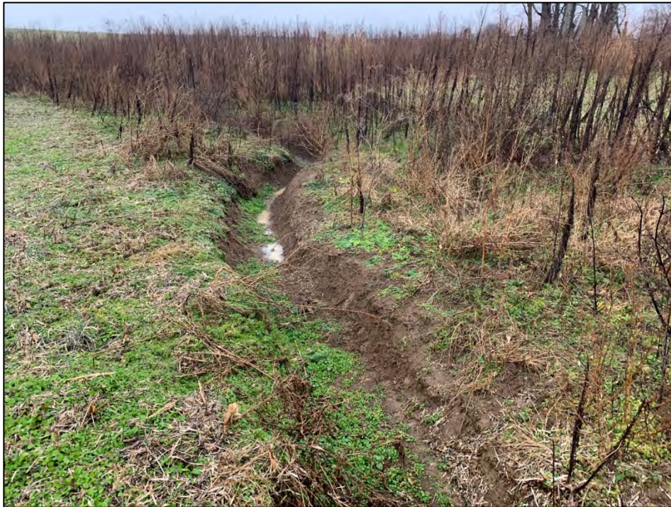
Photo 17: View of a typical excavated hillside ditch. View from Channel 4, facing west-northwest.
