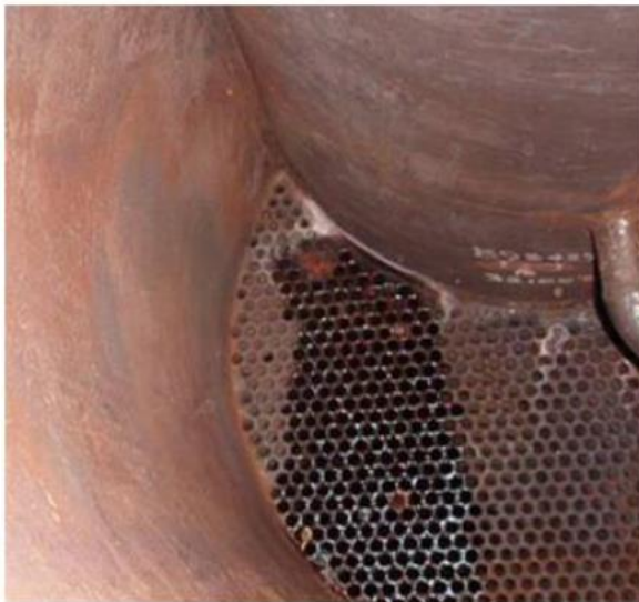
Industry photos of leaking Kettle Boilers and corrosion debris in rotor cooling air piping from ██████████ service bulletin.
