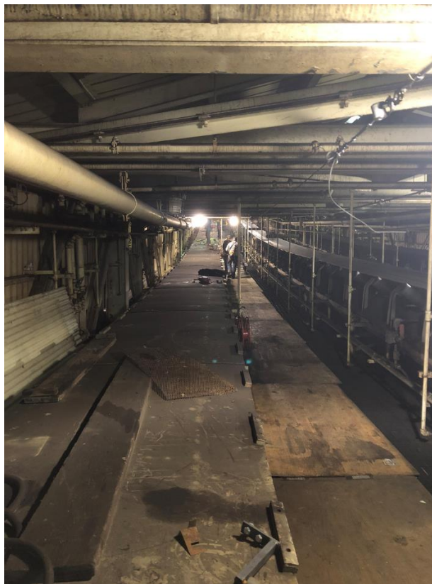
Figure 4: View of F coal conveyor galley looking south.
