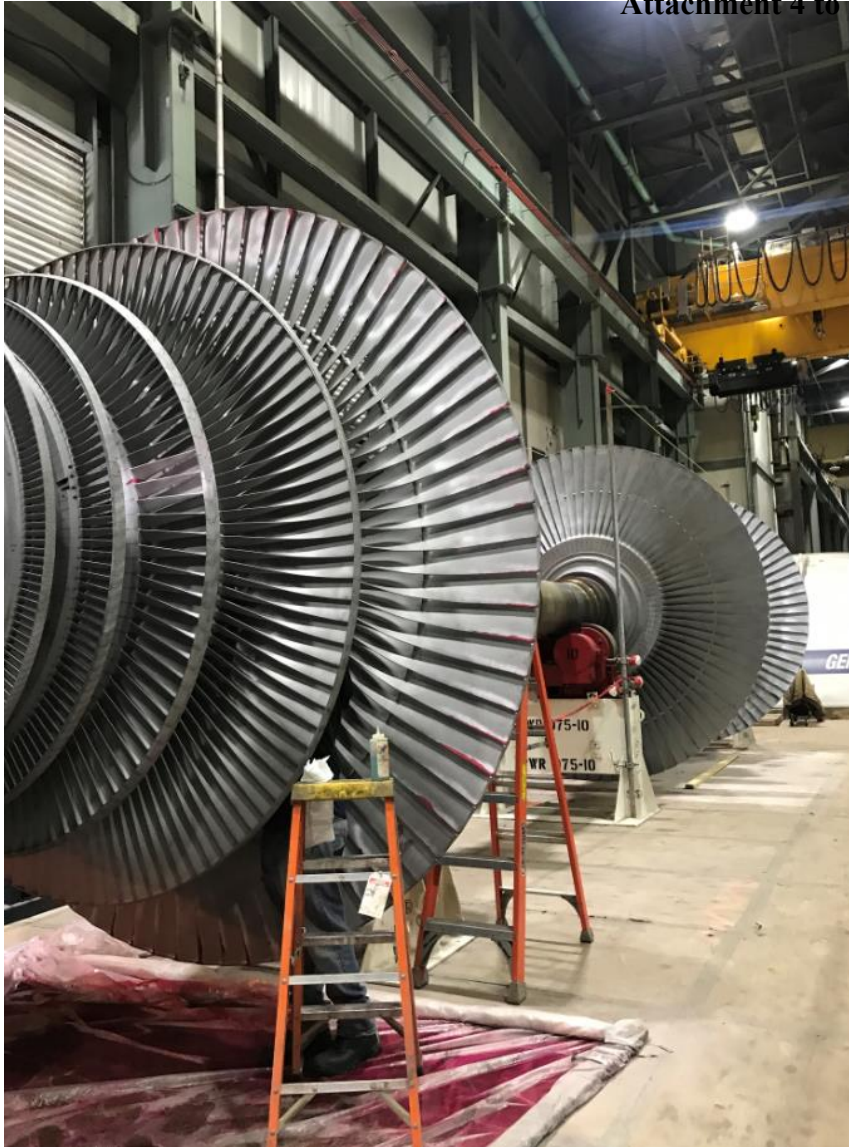
Figure 3. LP rotors on stands for inspection during 2019 spring outage
