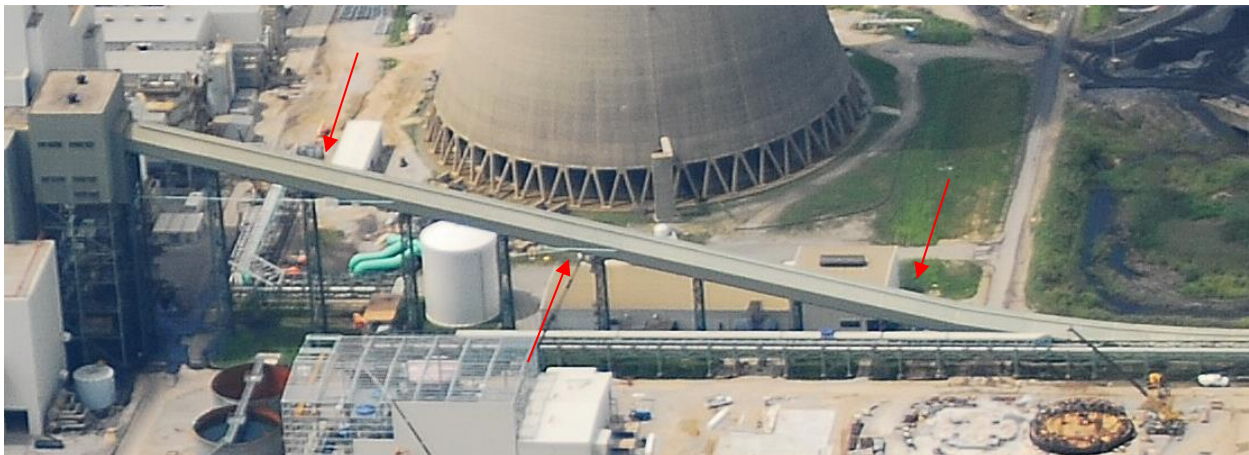
Figure 1. General overview of F coal conveyor gallery structure.
