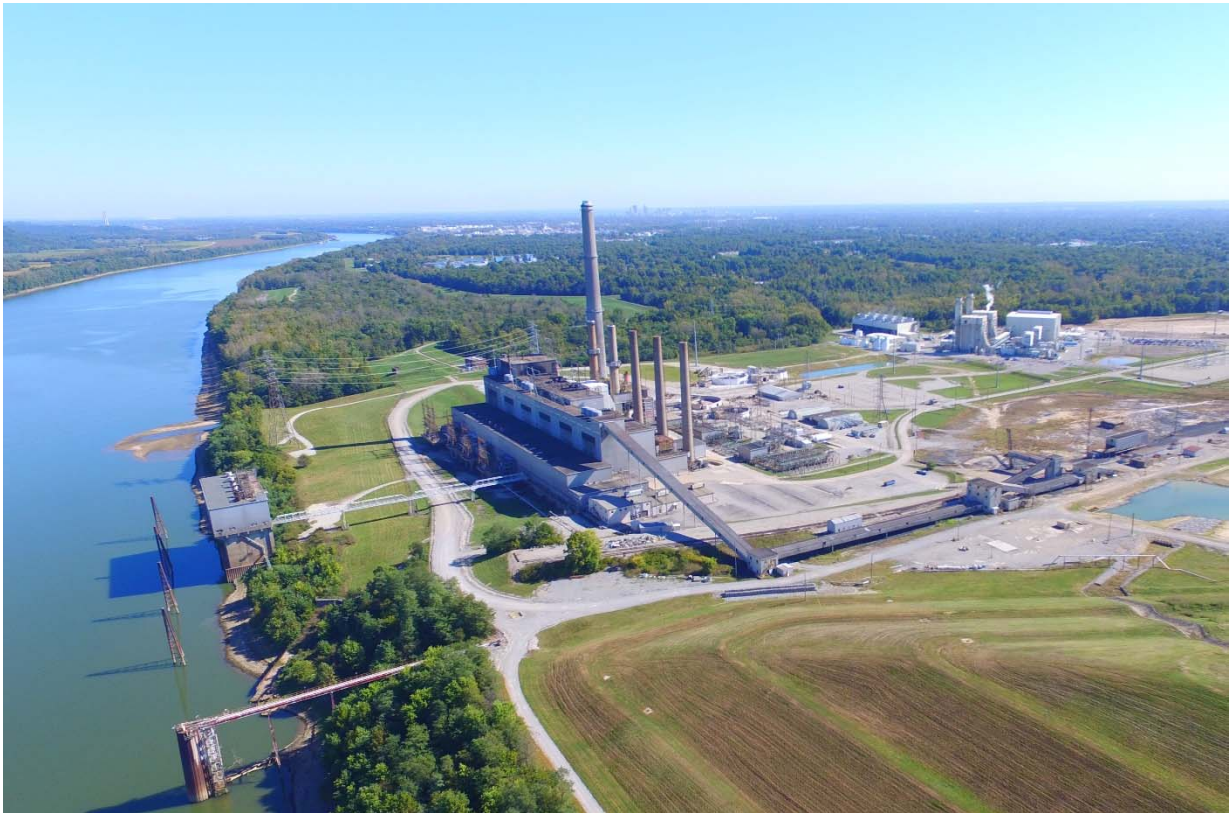
Cane Run Generating Station (2017)
