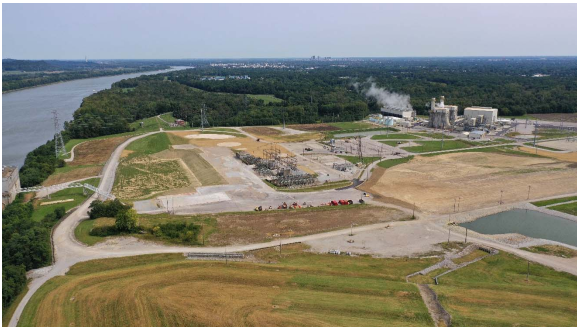
Cane Run Generating Station (2020)
