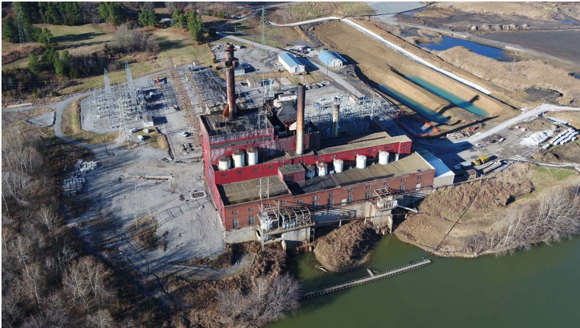
Green River Generating Station (2017)
