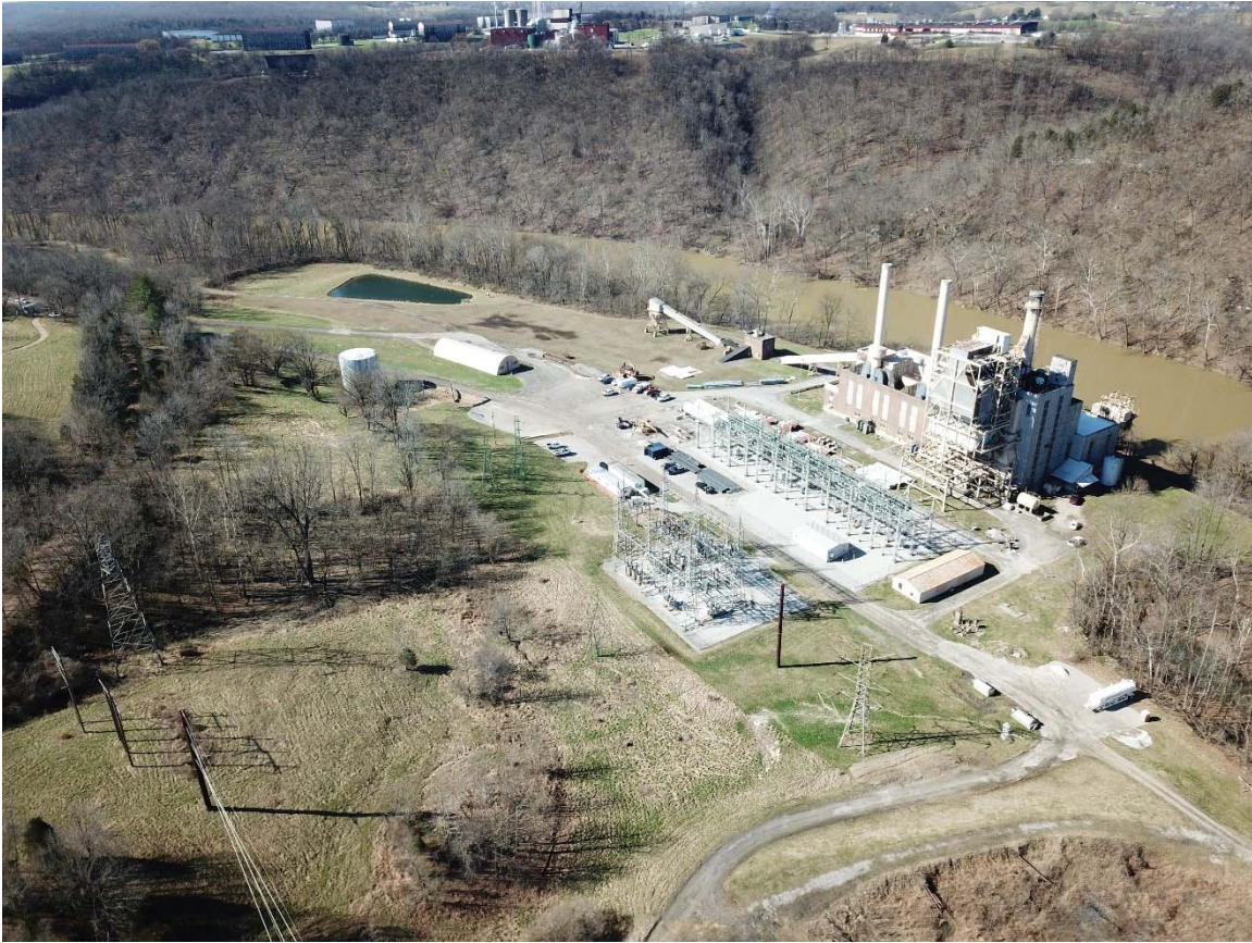
Tyrone Generating Station (2018)
