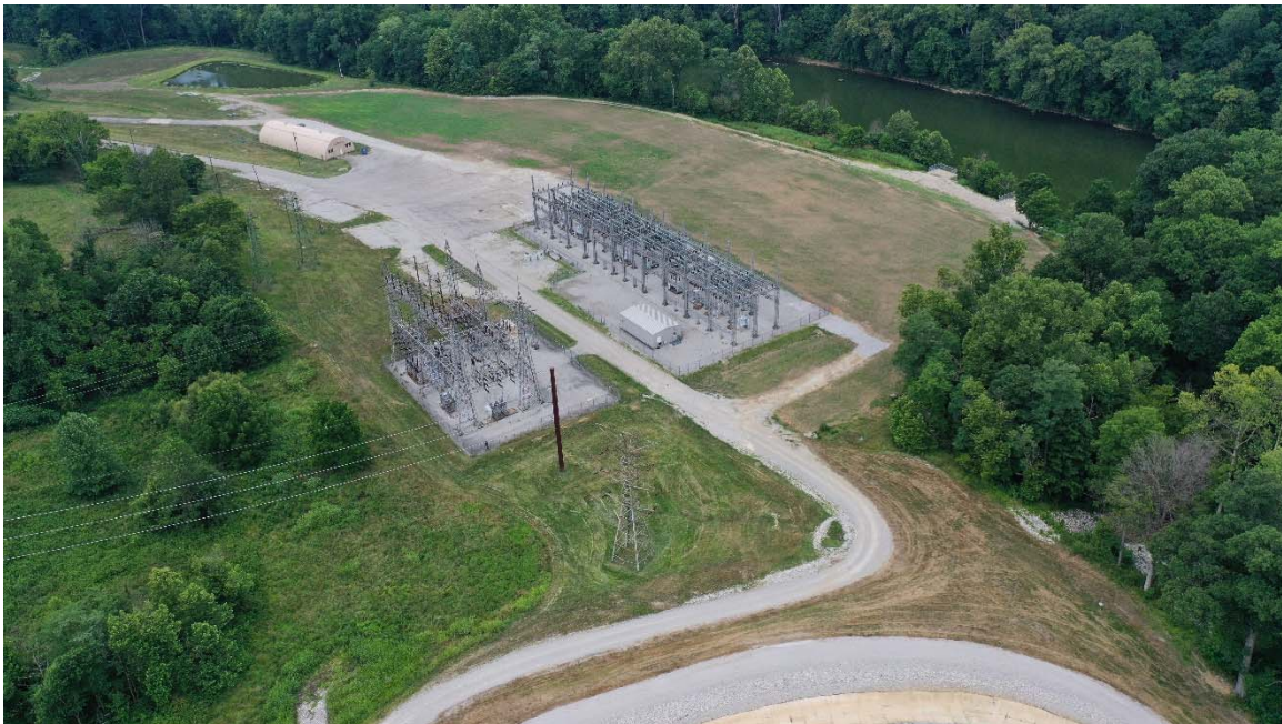
Tyrone Generating Station (2020)
