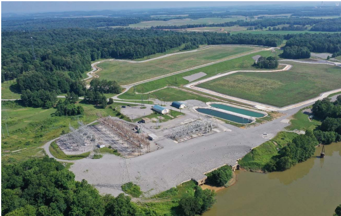
Green River Generating Station (2020)
