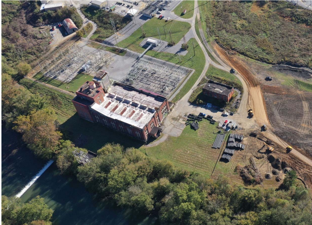
Pineville Generating Station (2018)
