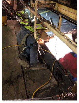
Figure 5. Employee grinding beneath F2 conveyor to install new panels.
