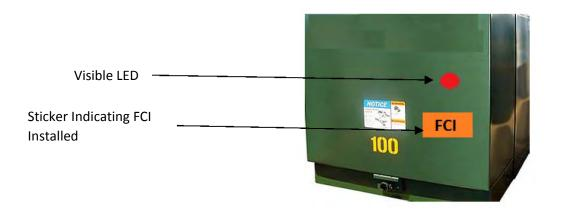
By locating the last flashing FCI and the first FCI not flashing, the trouble men have isolated the fault to a specific segment of the circuit.
