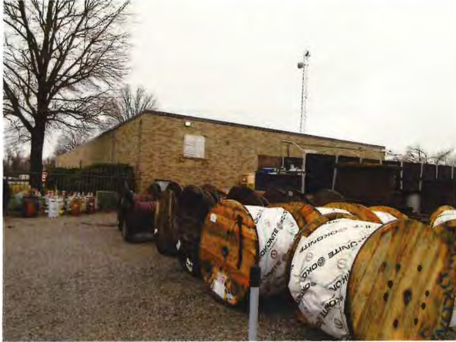
REAR & EAST SIDE OF BUILDING 3 (Photo Taken February 20, 2019)
