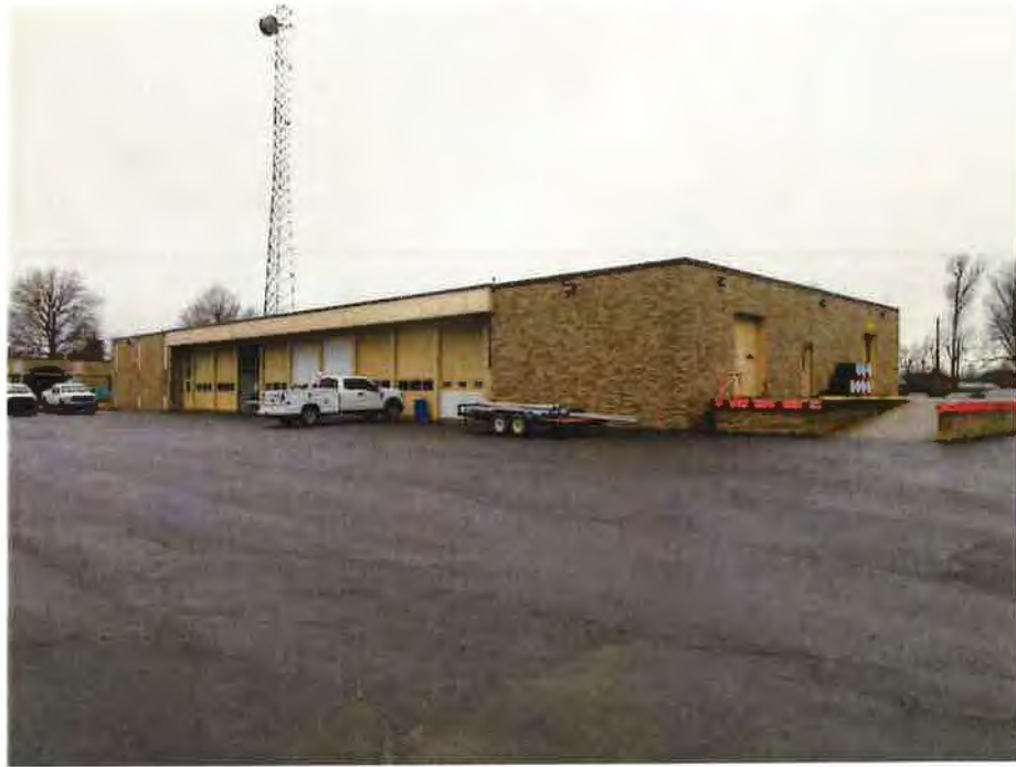
REAR & EAST SIDE OF BUILDING 2 (Photo Taken February 20, 2019)
