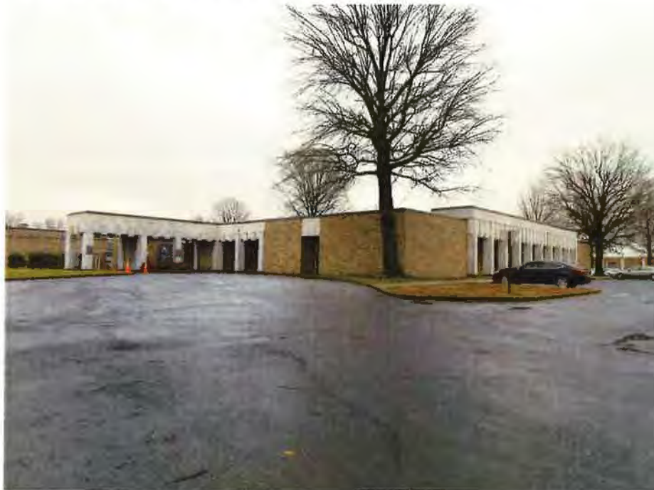
FRONT & WEST SIDE OF BUILDING 1 (Photo Taken February 20, 2019)
