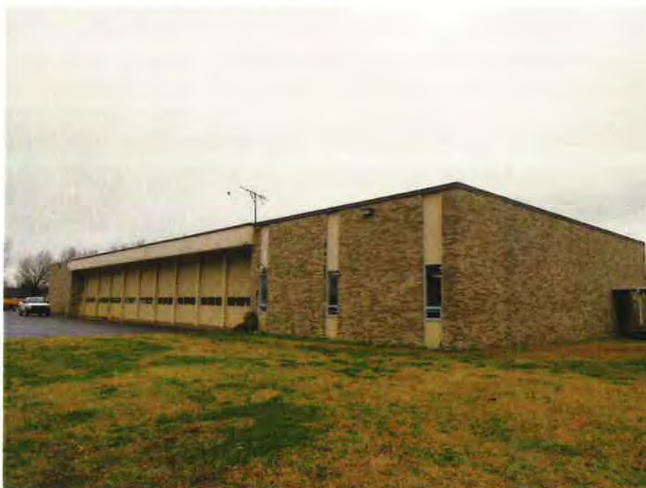
FRONT & WEST SIDE OF BUILDING 2 (Photo Taken February 20, 2019)
