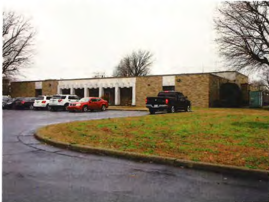
REAR & EAST SIDE OF BUILDING 1 (Photo Taken February 20, 2019)
