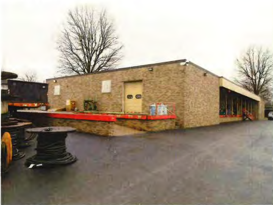
REAR & WEST SIDE OF BUILDING 3 (Photo Taken February 20, 2019)
