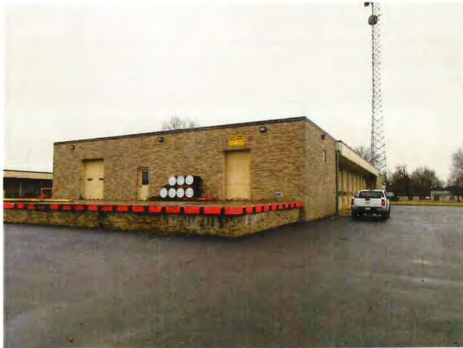
REAR & WEST SIDE OF BUILDING 2 (Photo Taken February 20, 2019)
