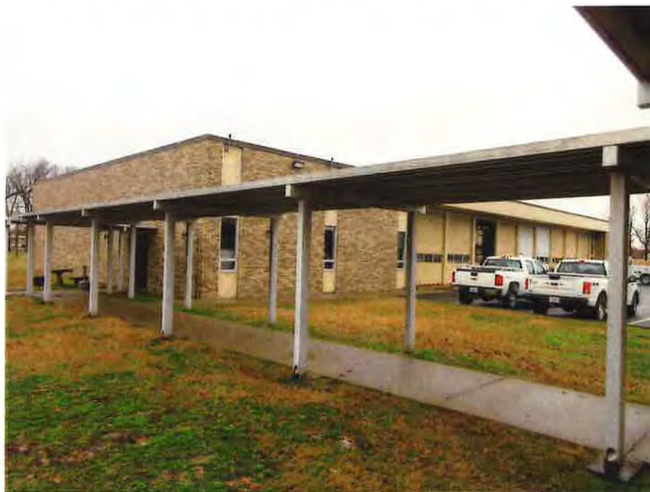
FRONT & EAST SIDE OF BUILDING 2 (Photo Taken February 20, 2019)
