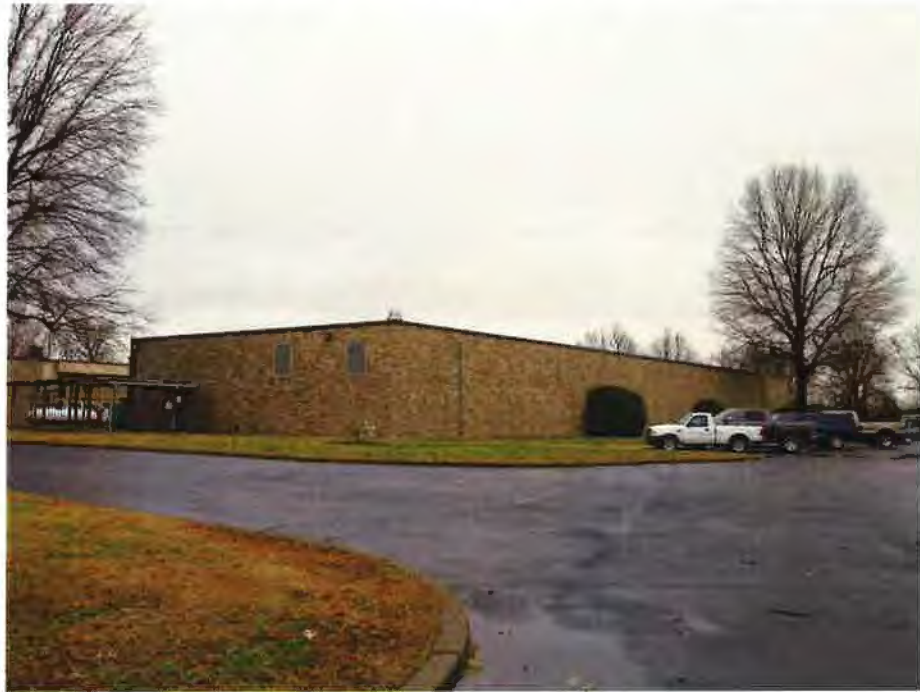
FRONT & EAST SIDE OF BUILDING 3 (Photo Taken February 20, 2019)
