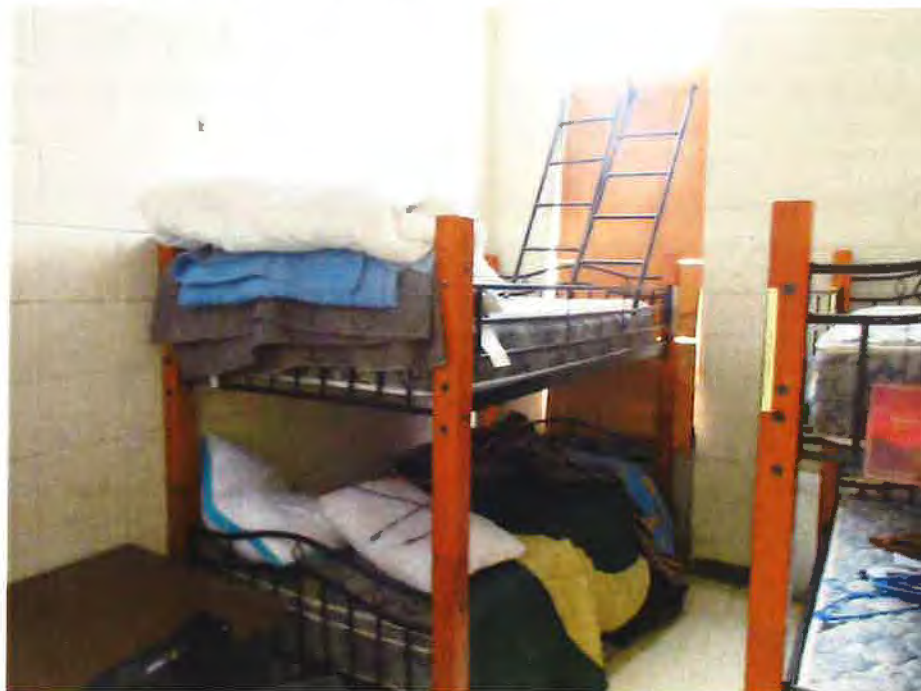
INTERIOR OF BUILDING 2 (Photo Taken February 20, 2019)
