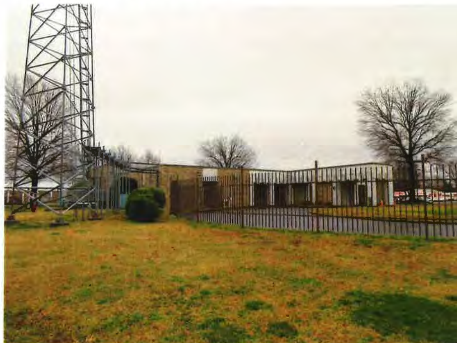
REAR & WEST SIDE OF BUILDING 1 (Photo Taken February 20, 2019)
