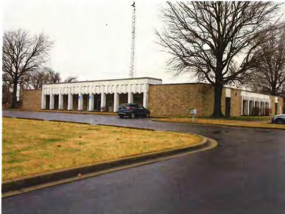
FRONT & EAST SIDE OF BUILDING 1 (Photo Taken February 20, 2019)
