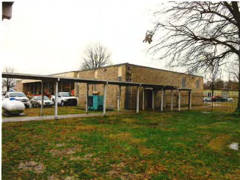
FRONT & WEST SIDE OF BUILDING 3 (Photo Taken February 20, 2019)
