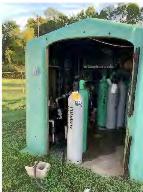
Gaseous Chlorine Storage
