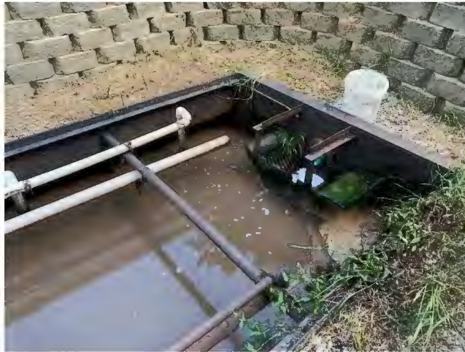
Manually Cleaned Bar Screen
