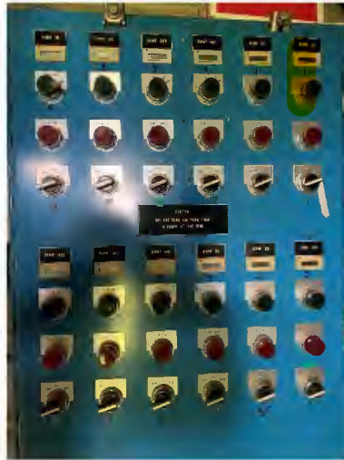
Irrigation Pump Stations Control Panel
