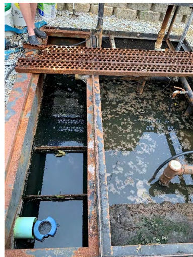
Clarifier and Contact Tank
