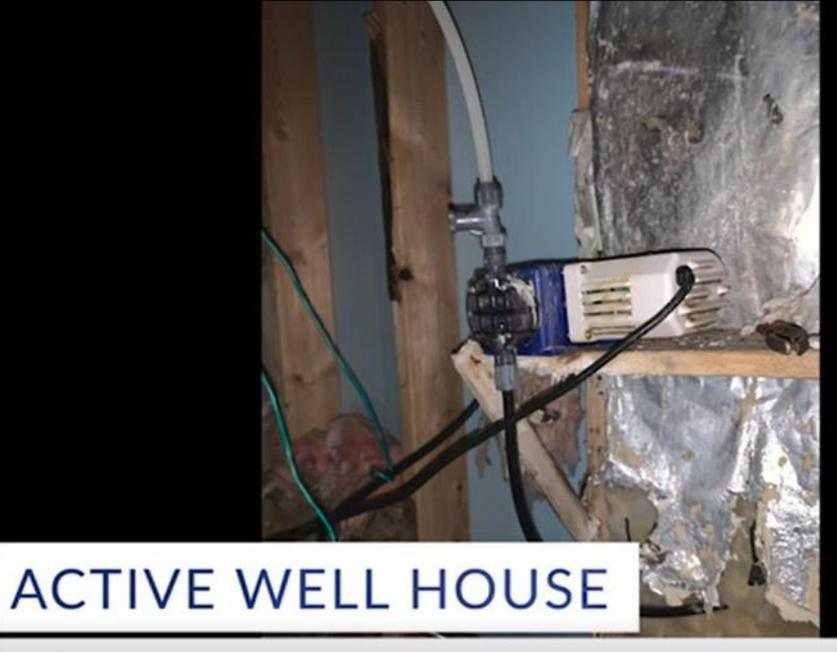
STATUS: OBSOLETE AND IMPROPERLY INSTALLED DOSING PUMP, EXPOSED WIRING
