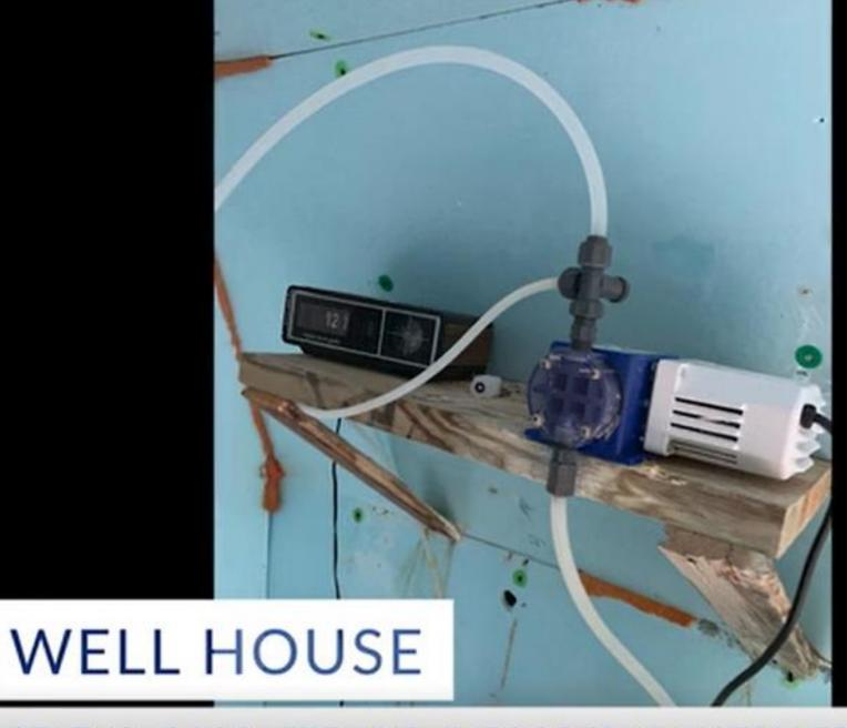
STATUS: OBSOLETE AND IMPROPERLY INSTALLED DOSING PUMP
