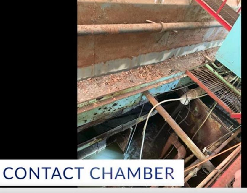
STATUS: EXCESSIVE CORROSION, IMPROPER CHLORINE DOSING
