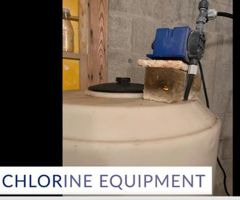
STATUS: OBSOLETE AND IMPROPERLY INSTALLED DOSING PUMP
